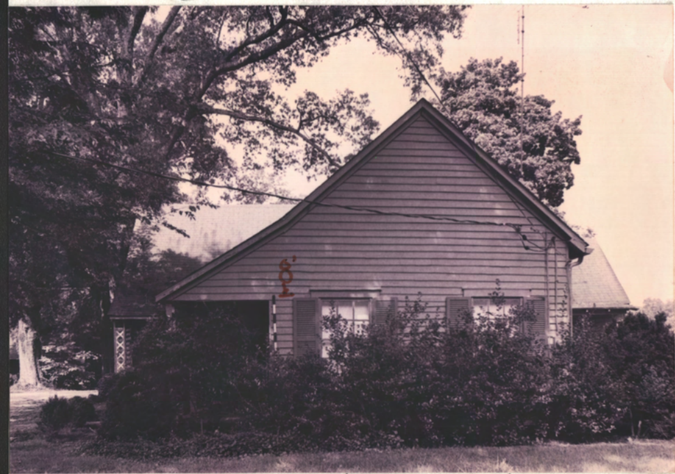
Vic. east wall →
