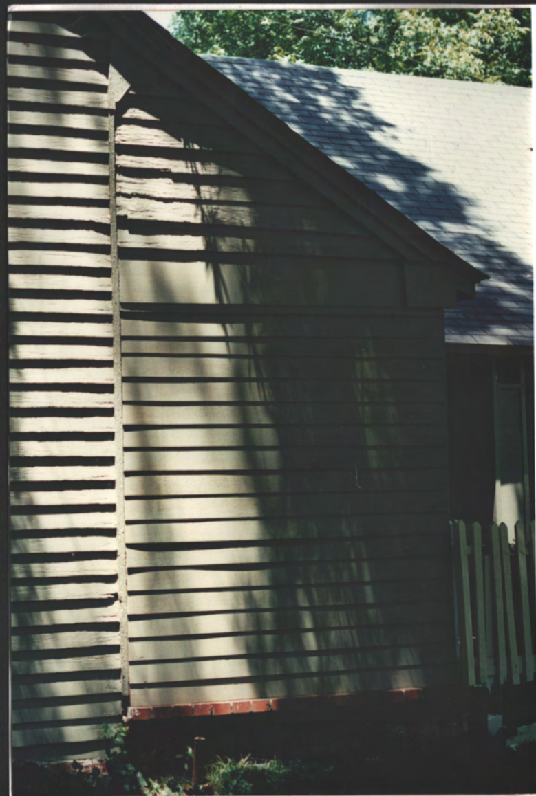
↙ S.E. corner of Fed. Period house
