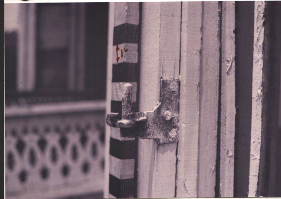
C.I. Blind-hinge at fl. 1, S.W. bay
