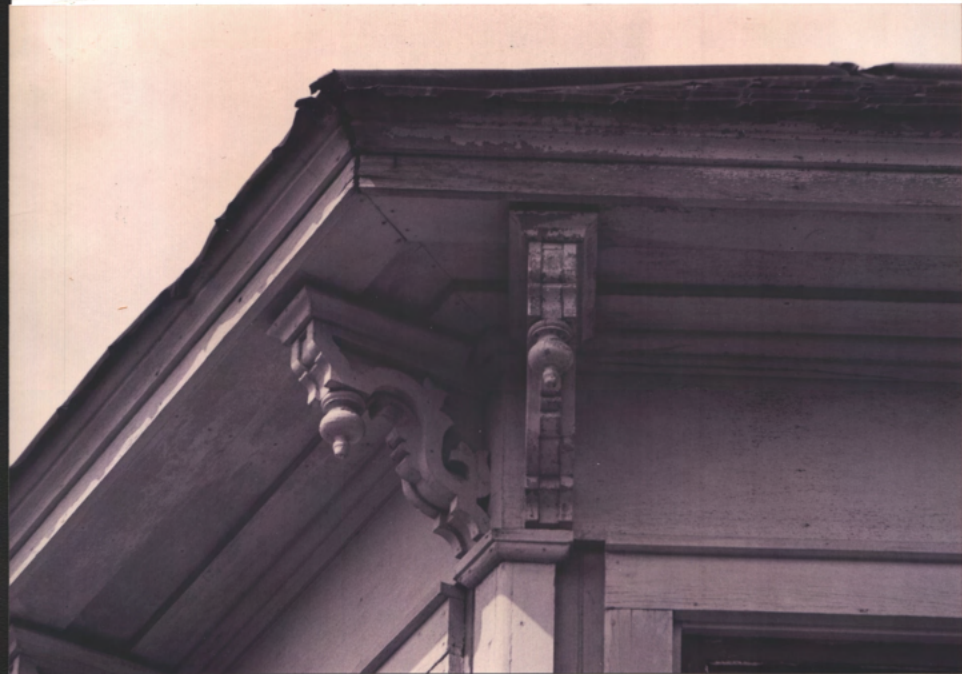
H ← S.W. Bay Window at roof
