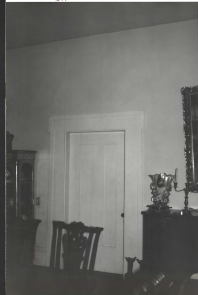
Orig. 2-pm. Gl. Rev. bi-fold doors between entry & double-parlor (this is S. jamb at ext. parlor)
