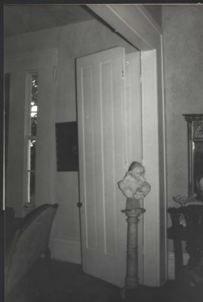
Orig. 2-pm. Gl. Rev. bi-fold doors between entry & double-parlor (this is S. jamb at ext. parlor)
