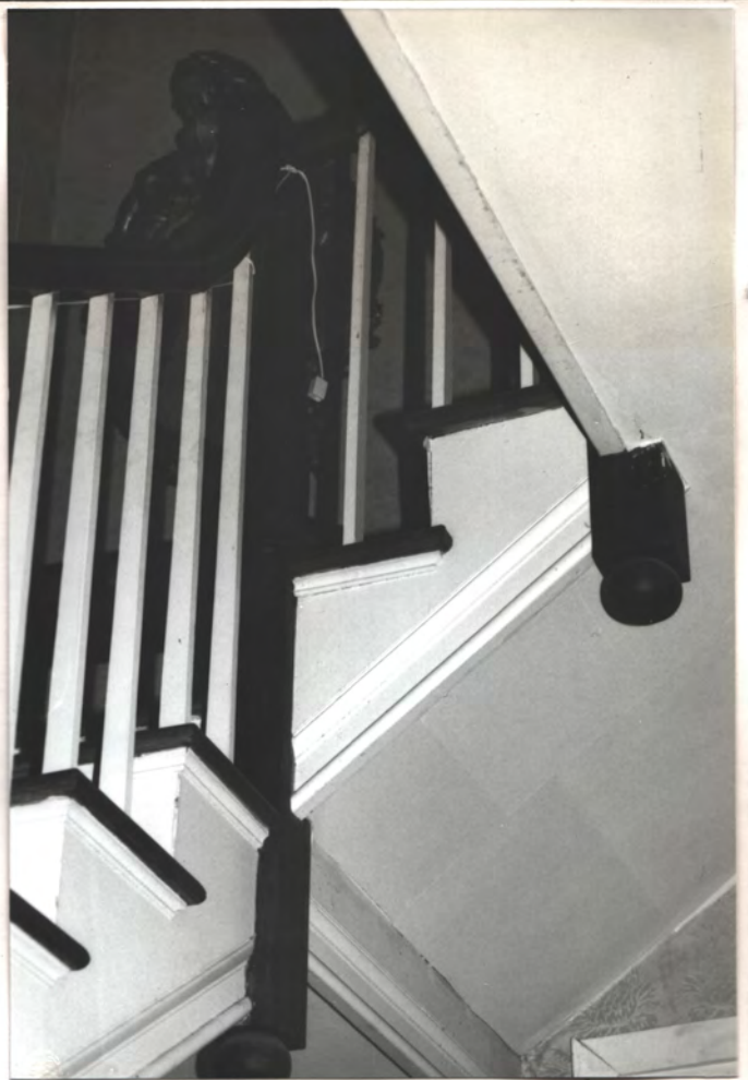
MID- LNDING → N Crown (N.) door frame
