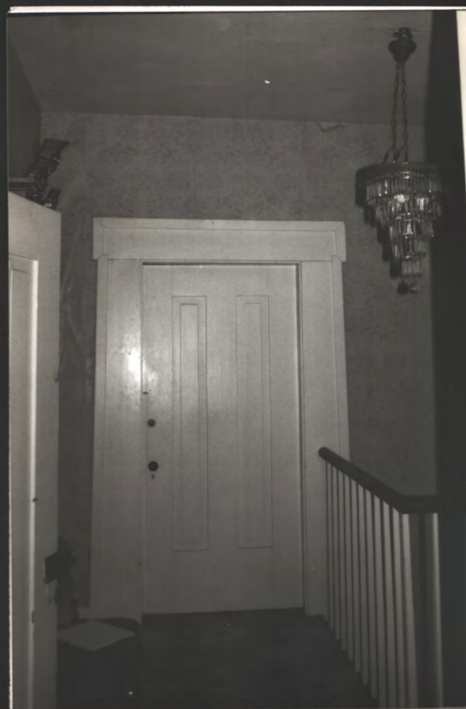
Fl. 2, door to N.W. Rm from stairwell
