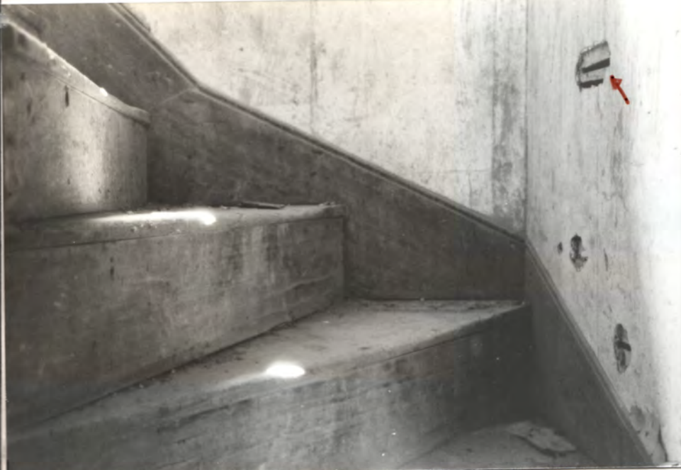
HALL STAIR AT "TURN" 22 1/2" windows
