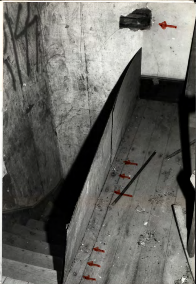
HALL STAIR AT FL. 2 thin plywd "rail" HALL STAIR FROM FL. 2
