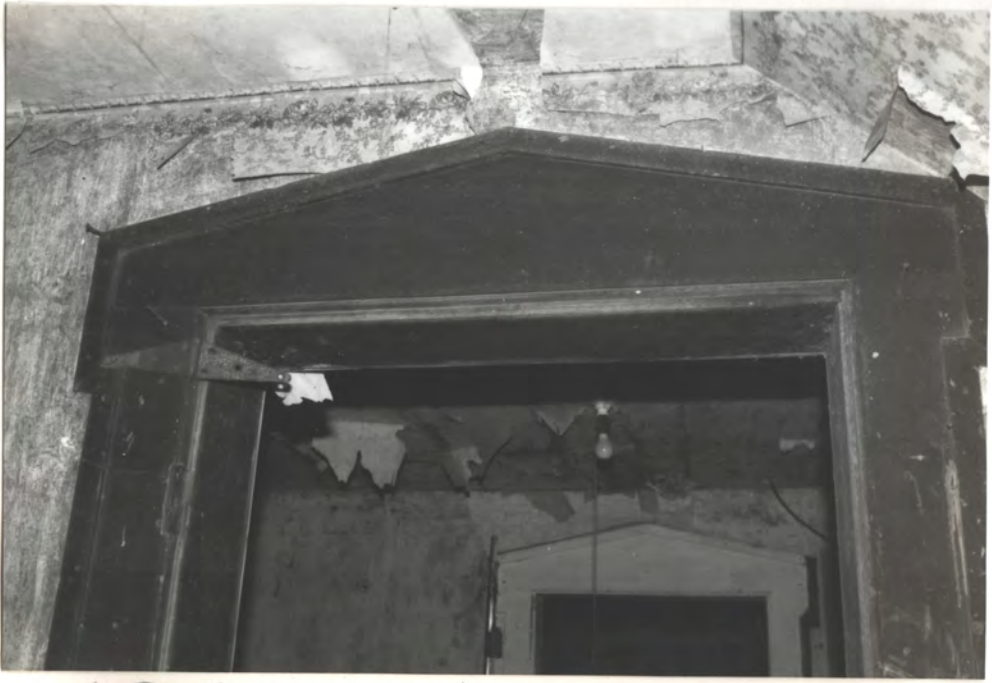
S. DOOR TO HALL (look S. into hall)
