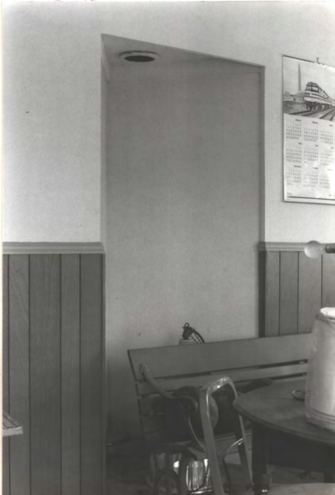
TRIANGULAR OPNG WAS OPEN TO GRILLE, HAD STOVE IN TRIANGLE. SEE LEFT
