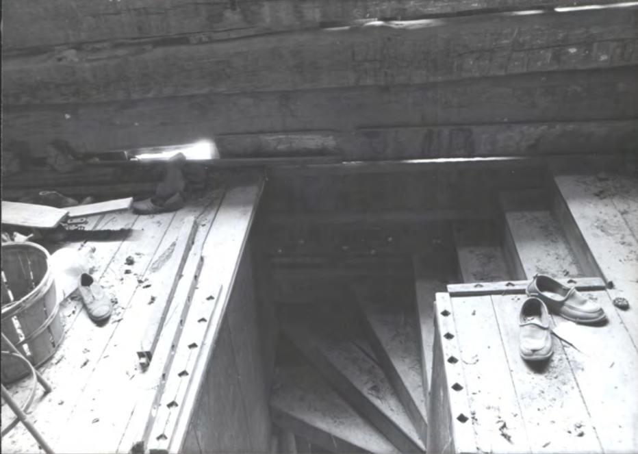
STAIR IN LOFT. Note baluster mortises
