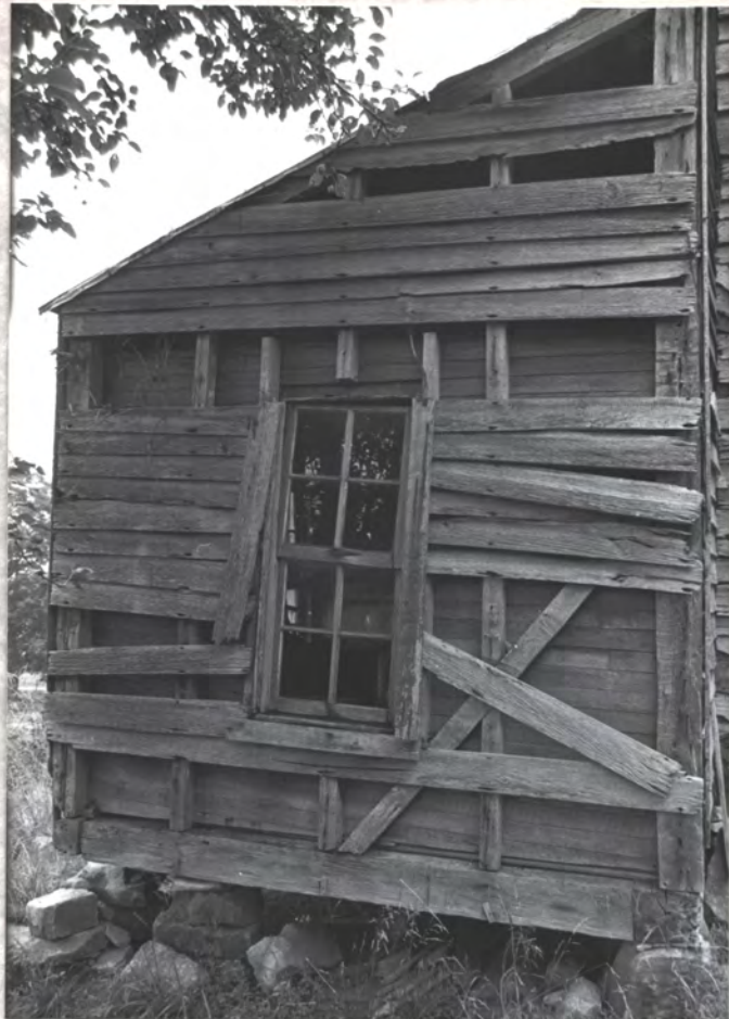
1st ADD. PHRAMING INDICATES PRE 1860 CONSTN - HEAVY SILLS, 2" X 4" STUDS 2' + 0" C., STUDS MORTISED INTO SILLS. V.C. SESS IS CUT IN LATER, PER PHRAMING
