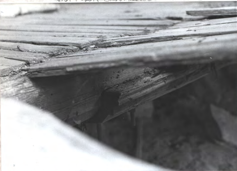
PUNCHHOLE JOIST UNDER DECK
