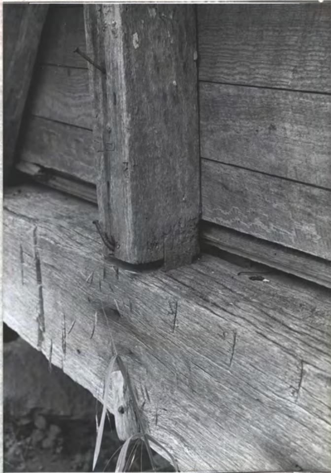
1st ADD. PHRAMING INDICATES PRE 1860 CONSTN - HEAVY SILLS, 2" X 4" STUDS 2' + 0" C., STUDS MORTISED INTO SILLS. V.C. SESS IS CUT IN LATER, PER PHRAMING
