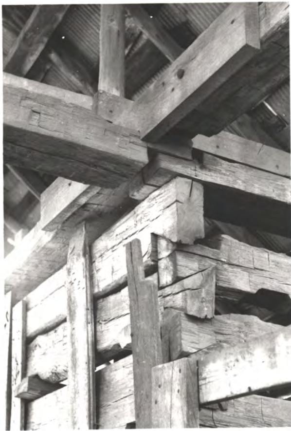
Detail at ridge, N → E. end
