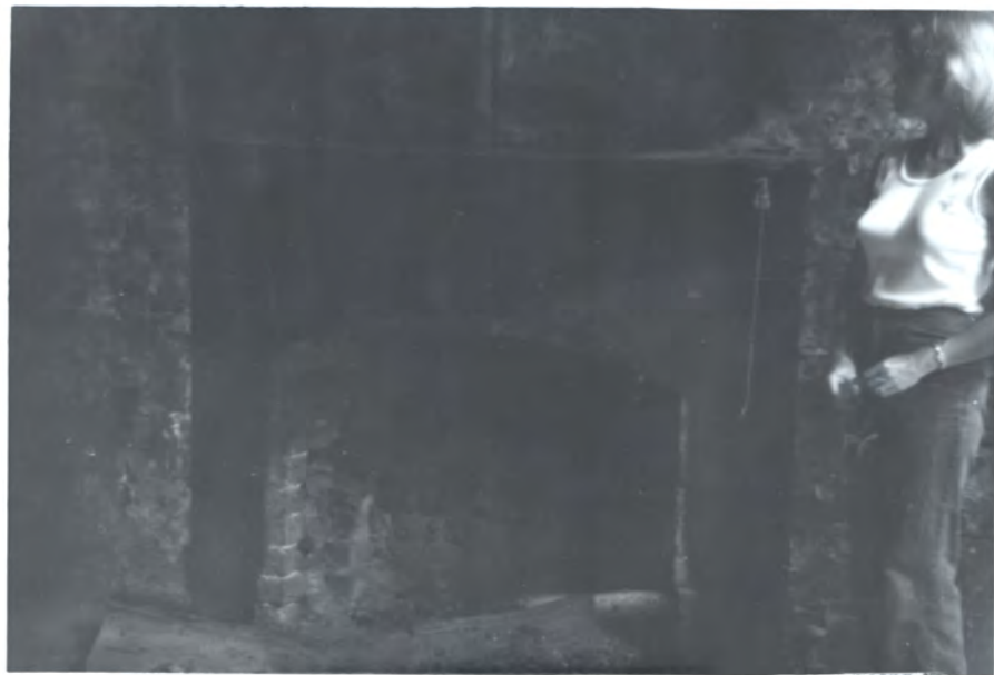
Mantel - Fl. 1 E. Rm (bottom is patched) Original finish = black (typical for 1850-1860) Arch is unusual
