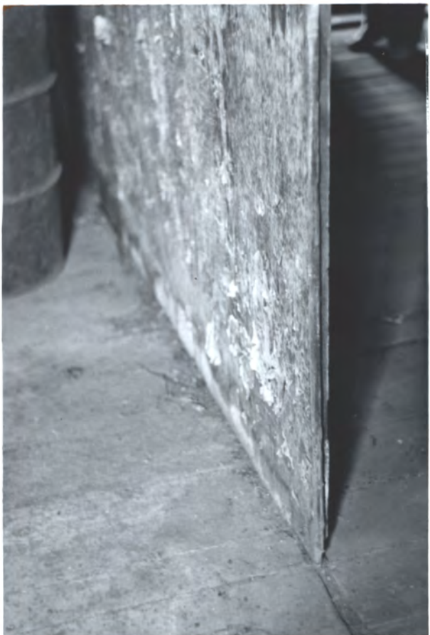
Fl. 2 center partition N of Vert. \pm 5/4 \times 6 T&G planks. No base
