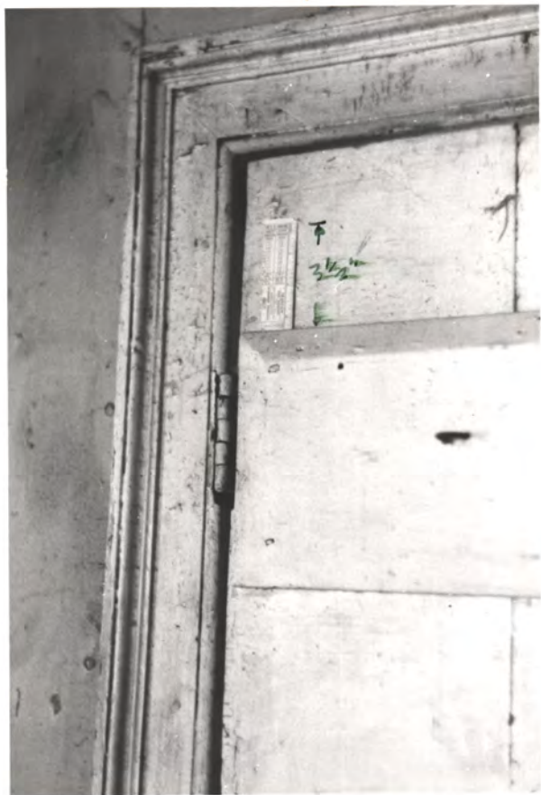
Fl. 1, E. Rm., door to W. Rm. hinge = unitary cast iron Note 3 1/2" ruler on batter
