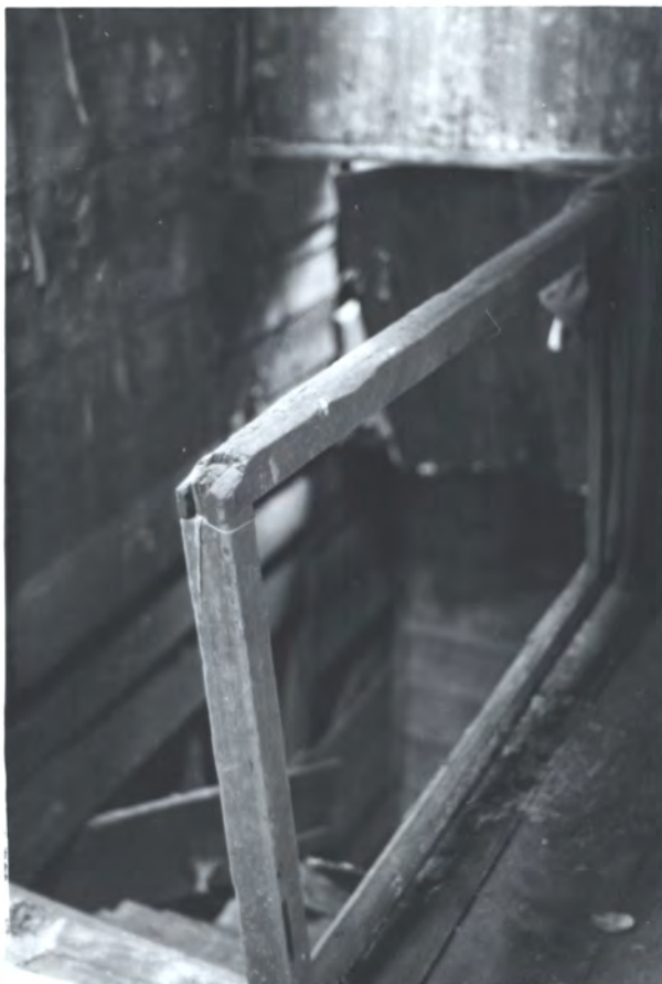
Fl. 2 center partition N of Vert. \pm 5/4 \times 6 T&G planks. No base
