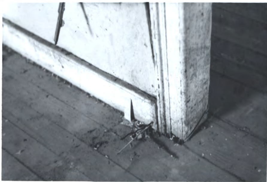
Chop-beaded \pm 5/4 \times 6 base (typical of Fed. Period)
