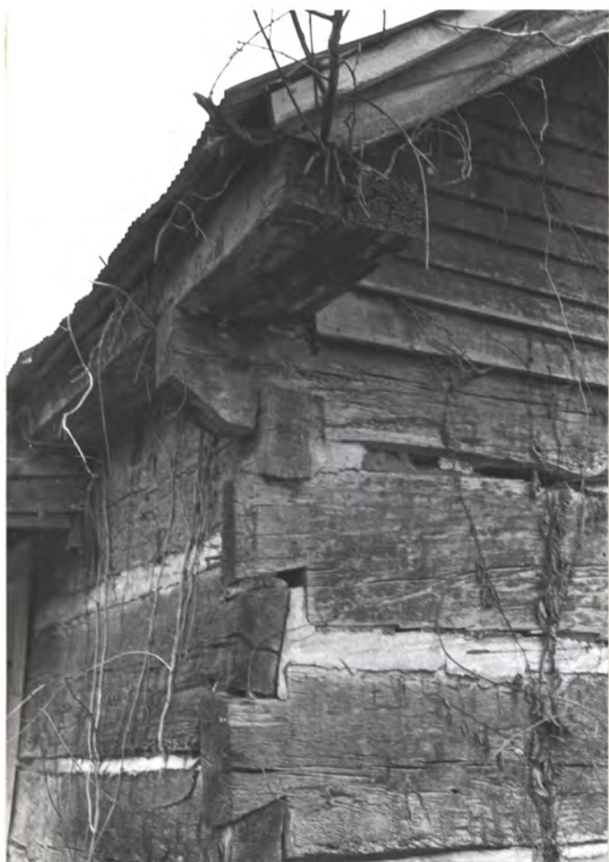
S.E. corner - half dovetail notch
