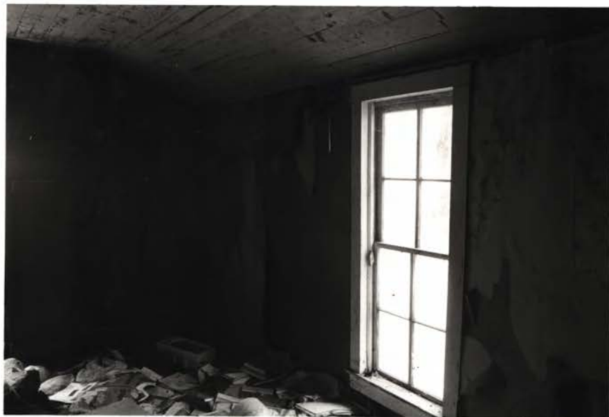
SOUTH WEST CORNER OF ROOM D.
