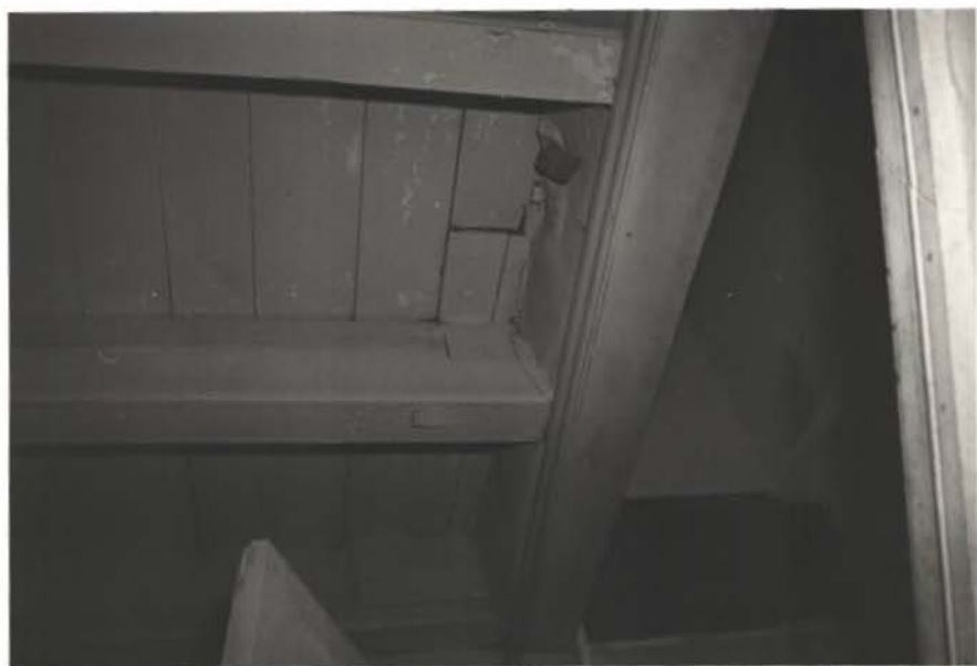
CEILING BEAMS BY STAIRWAY IN ROOM B. NOTE PLUGS IN BEAMS.
