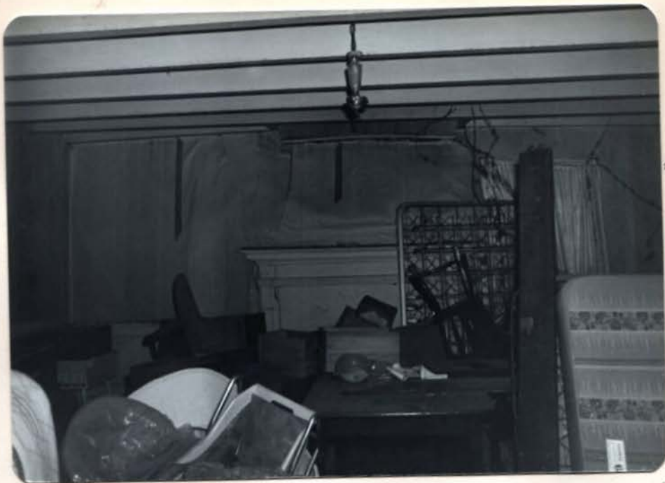
SOUTH WALL OF ROOM A. MANTEL IS NOT ORIGINAL TO CABIN BUT ADDED PROBABLY IN LATE 19 th CENTURY.
