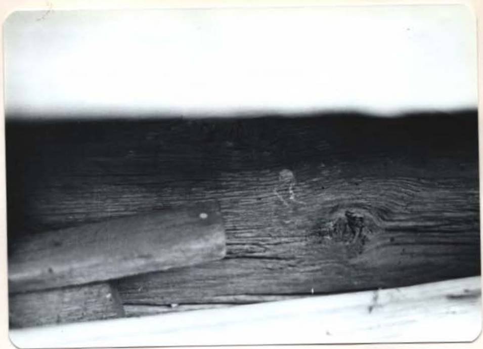
VIEW OF LOG AS SEEN THROUGH CLAPBOARDS
