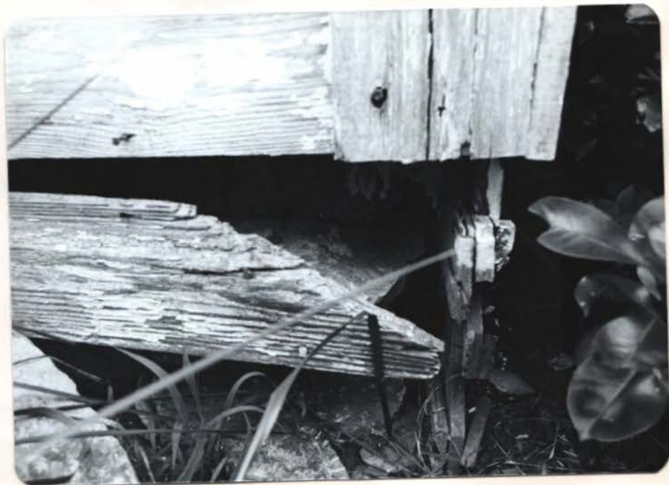
SOUTHEAST CORNER SHOWING SILL BEAM RESTING ON STONE
