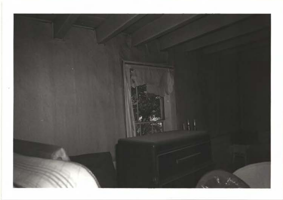
SOUTH EAST VIEW OF ROOM A
