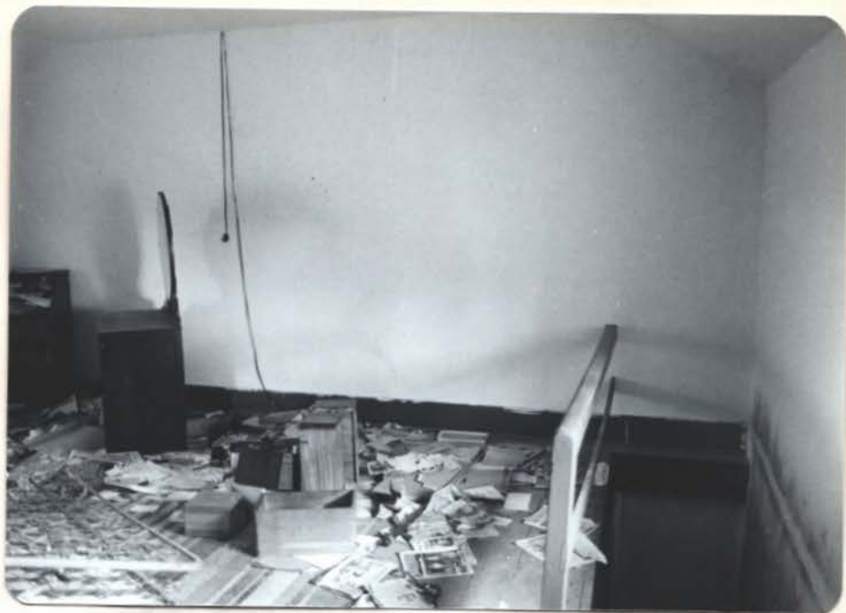
SOUTHWEST CORNER OF BEDROOM 1, STAIRWAY IN LOWER RIGHT HAND CORNER.
