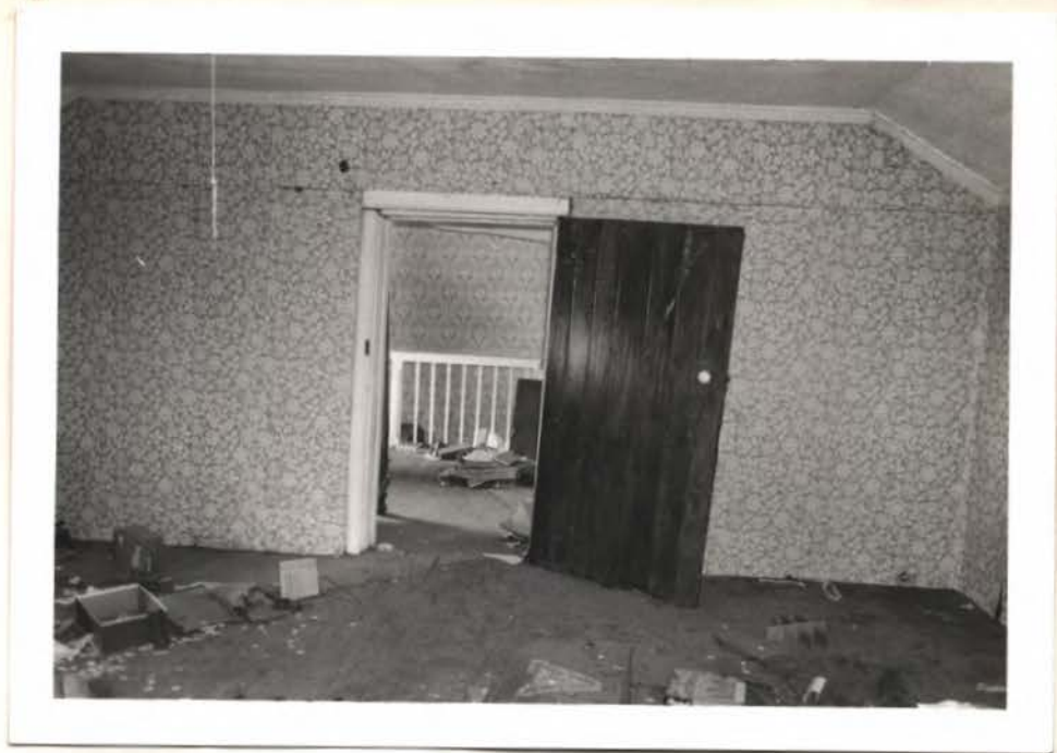
NORTH WALL OF BEDROOM 3.
