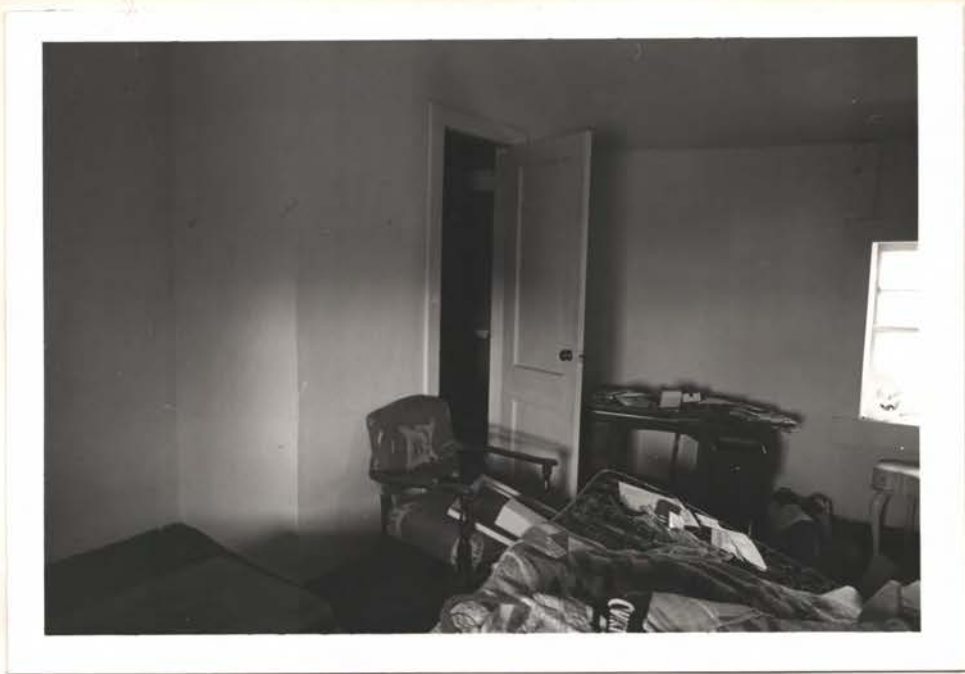
NORTHEAST CORNER OF BEDROOM 1. CLOSET IS MODERN ADDITION
