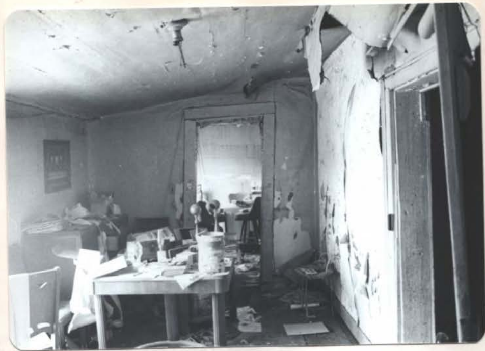
NORTH VIEW OF ROOM C, LOOKING TOWARD KITCHEN
