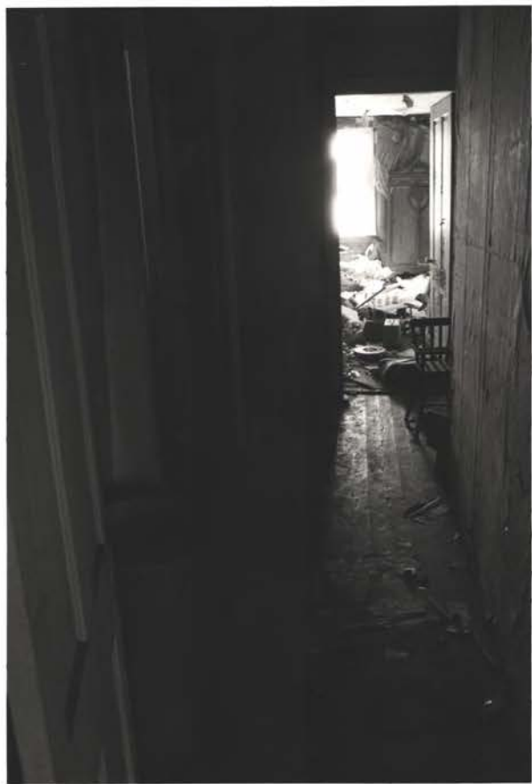
SOUTH VIEW OF HALLWAY LEADING TO ROOM D
