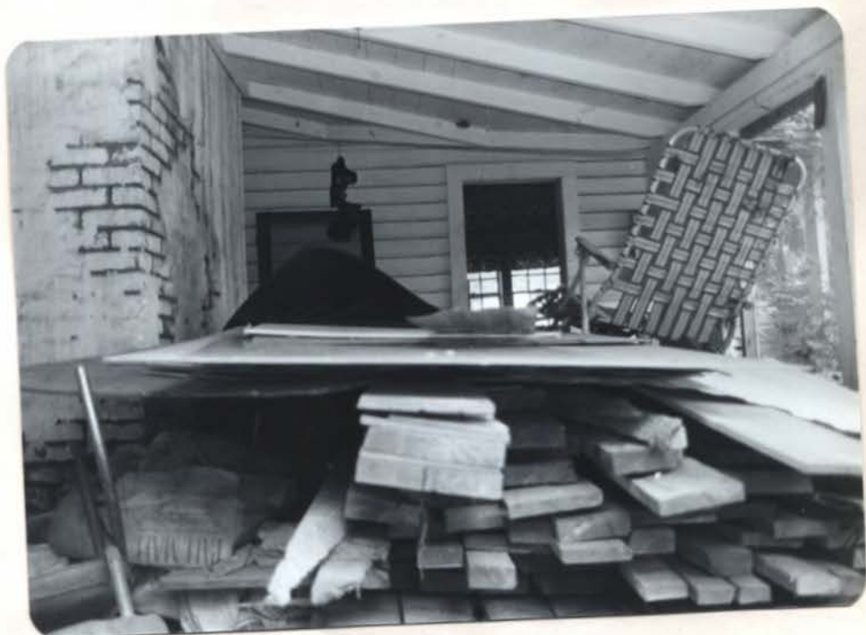
INTERIOR VIEW OF PORCH, LOOKING WEST TOWARD KITCHEN
