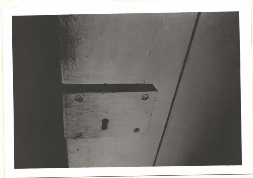
LOCK BOX ON CLOSET DOOR
