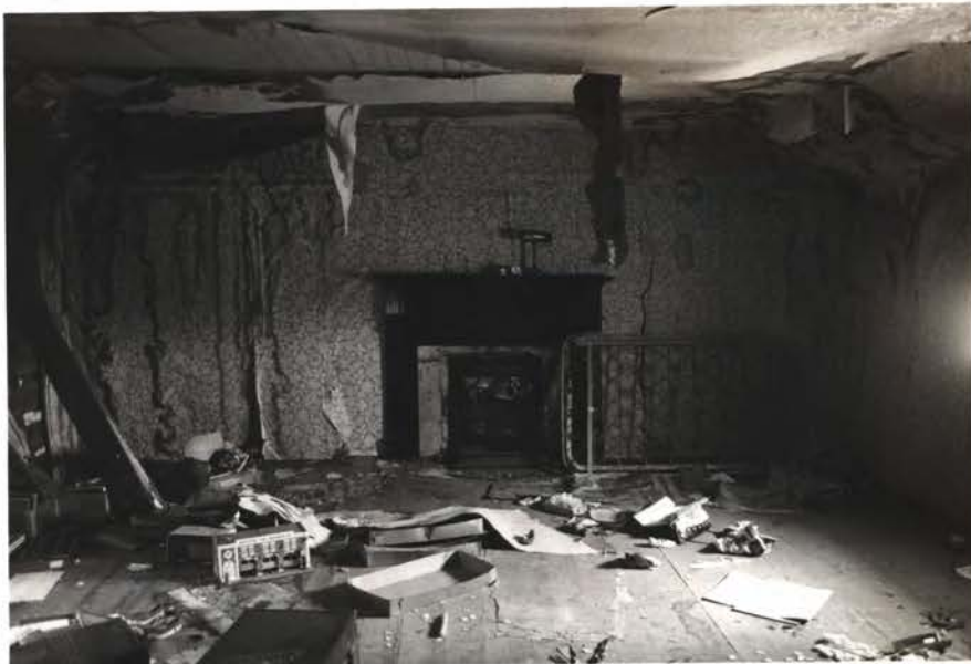
SOUTH WALL OF BEDROOM 3
