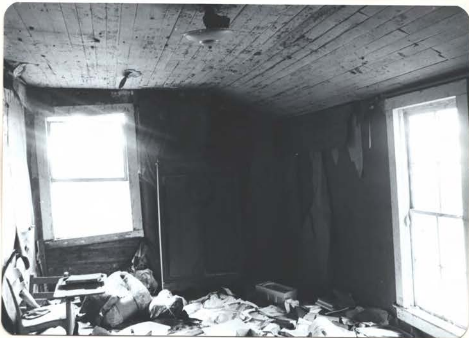
SOUTHWEST VIEW OF ROOM D
