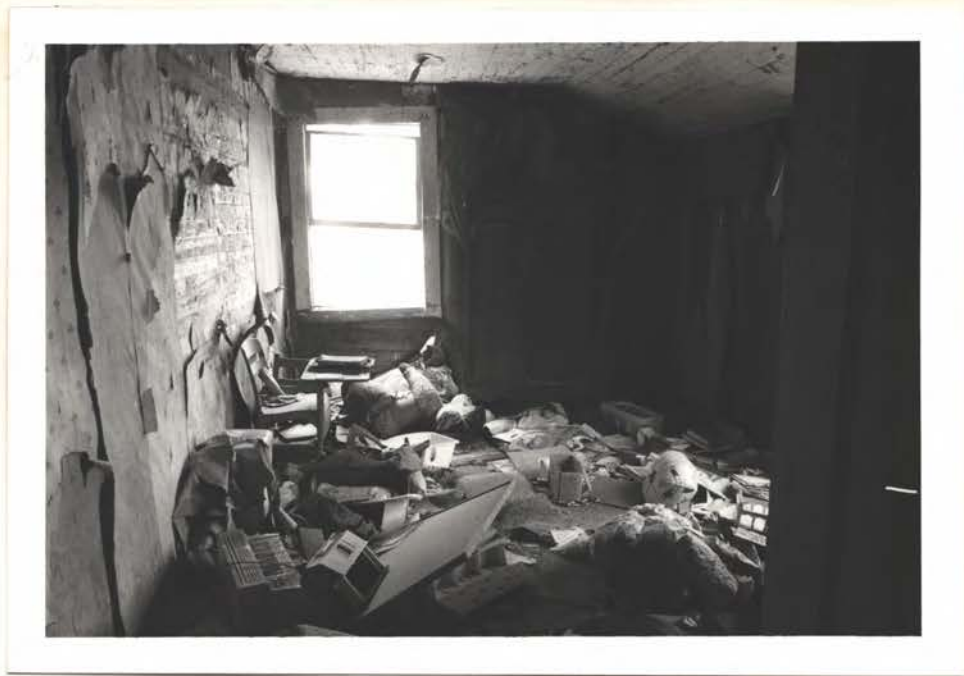
SOUTH VIEW OF ROOM D, PART OF 1ST ADDITION
