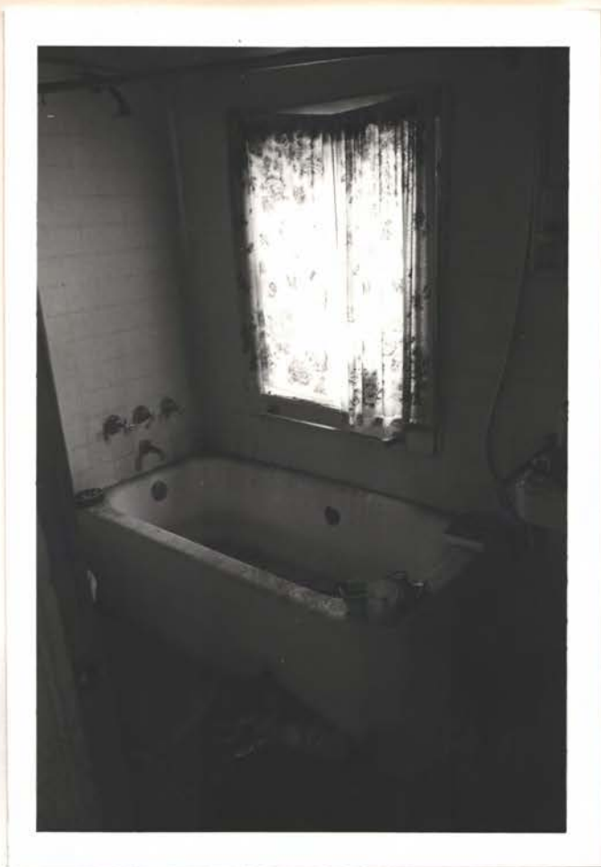
WEST VIEW OF BATHROOM OFF OF HALLWAY
