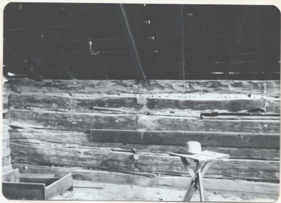
SOUTH WALL AND EAST CORNER OF LOFT
