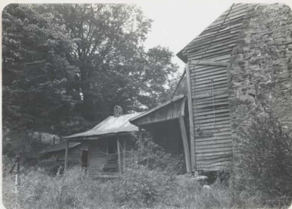
EAST FACADE OF 2 ND AND 3 RD ADDITION
