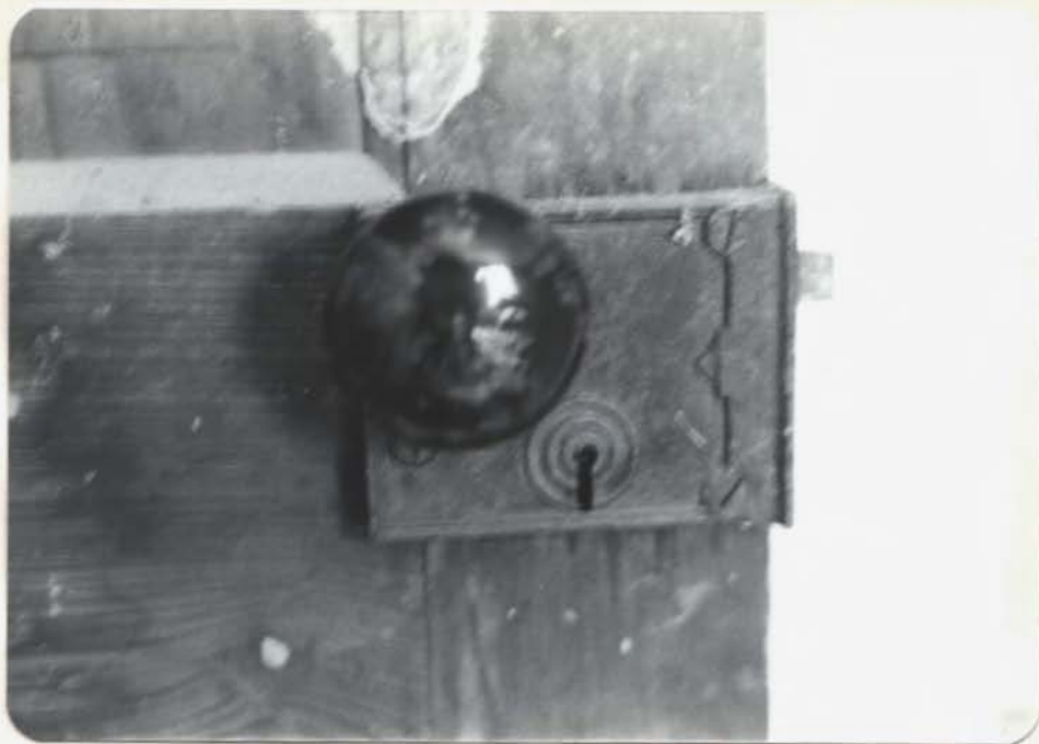
DOORKNOB AND LOCKBOX ON DOOR TO ROOM C
