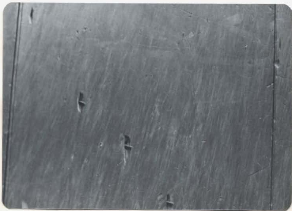
CLOSEUP OF PANELING ON WALL OF THE STAIRWAY
