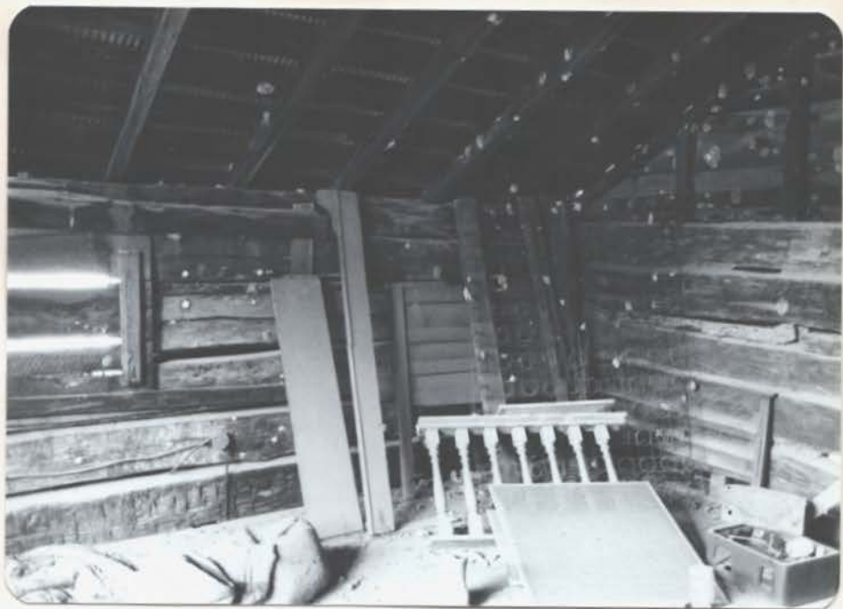
NORTHEAST CORNER. NOTE ADZE MARKS OF BOTTOM LOG
