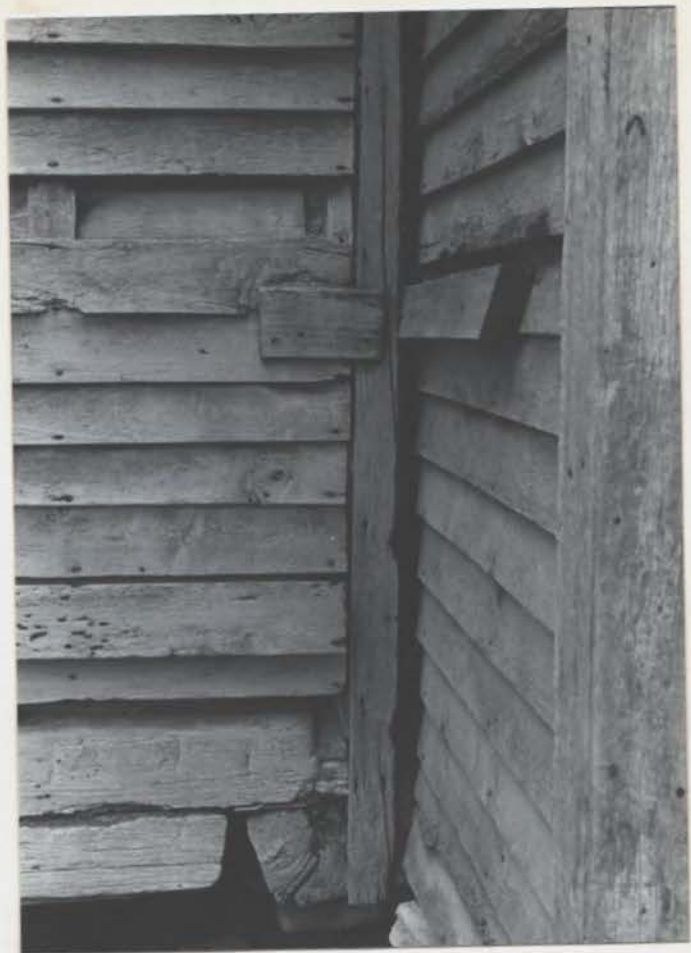
JUNCTION OF CABIN AND 2 ND ADDITION NOTE EXPOSED CORNER LOG
