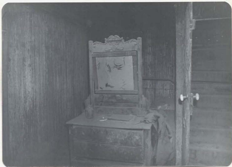
SOUTH WEST CORNER OF CABIN SHOWING DOOR TO STAIRWAY
