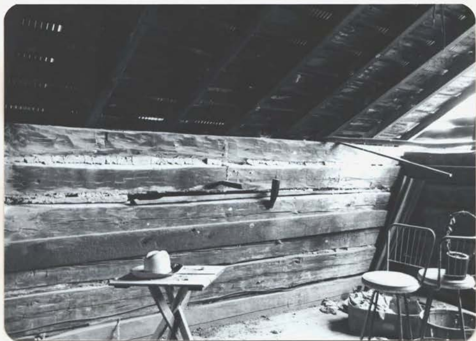
SOUTH WALL AND WEST CORNER. ALL LOGS ARE OF CEDAR
