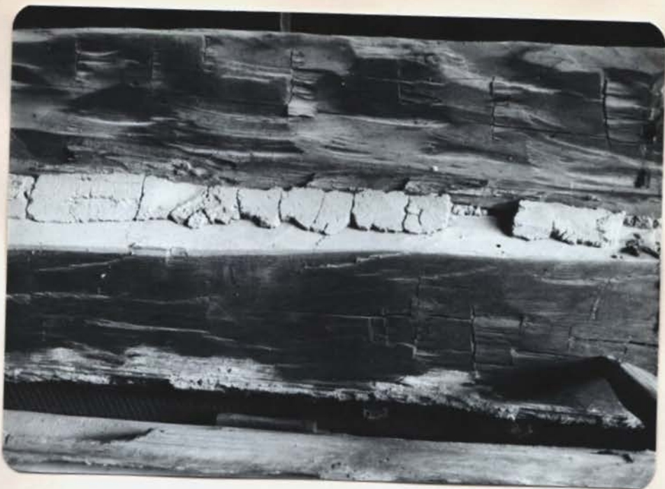
CLOSEUP OF LOGS AND CHINKING
