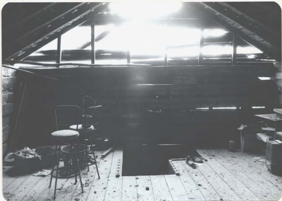
WEST VIEW OF LOFT SHOWING STAIR OPENING FLOORBOARDS ARE OF POPLAR
