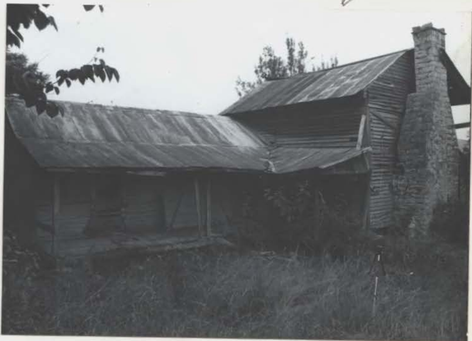
EAST FACADE OF ADDITIONS AND SOUTH FACADE OF ORIGINAL CABIN
