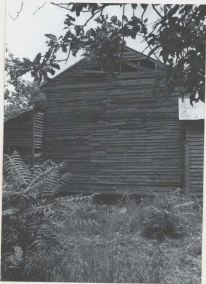
WEST FACADE OF ORIGINAL CABIN SHOWING JUNCTION OF ADDITIONS
