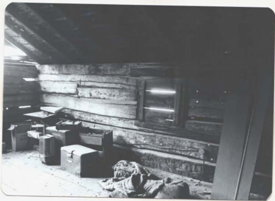
NORTHWEST CORNER SHOWING SMALL WINDOW THAT HAS BEEN BOARDED OVER
