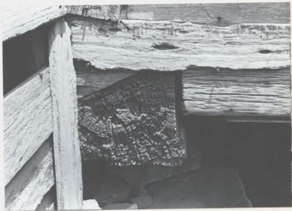
NORTHWEST CORNER OF CABIN SHOWING LOG NOTCHING
