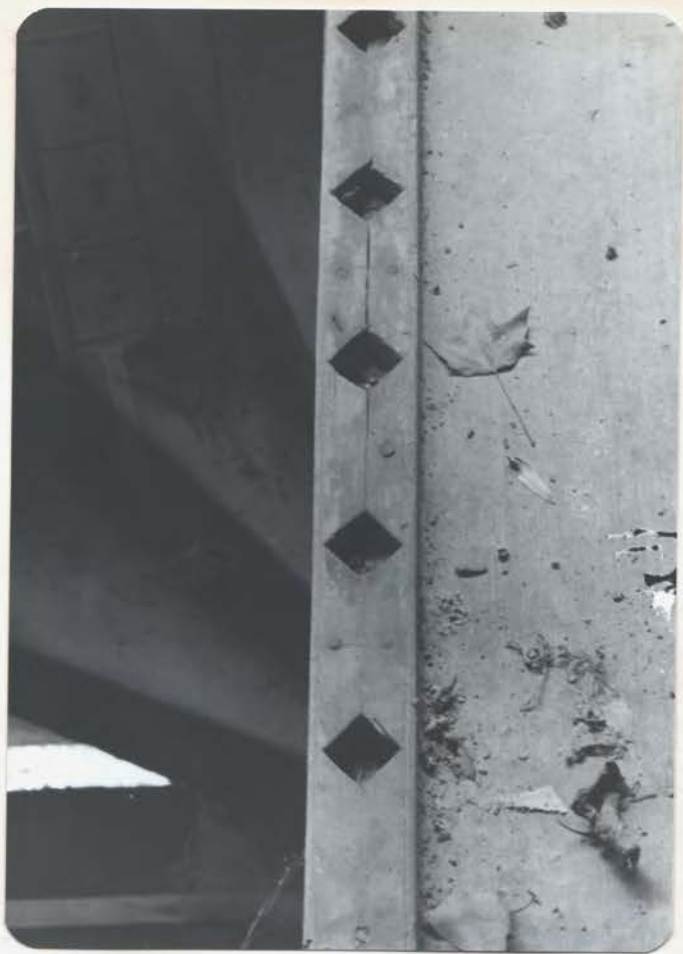
CLOSEUP OF RAFTING SUPPORT
