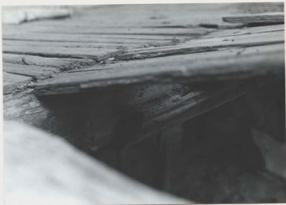
PORCH DETAIL SHOWING SUPPORT BEAM UNDER PORCH FLOOR
