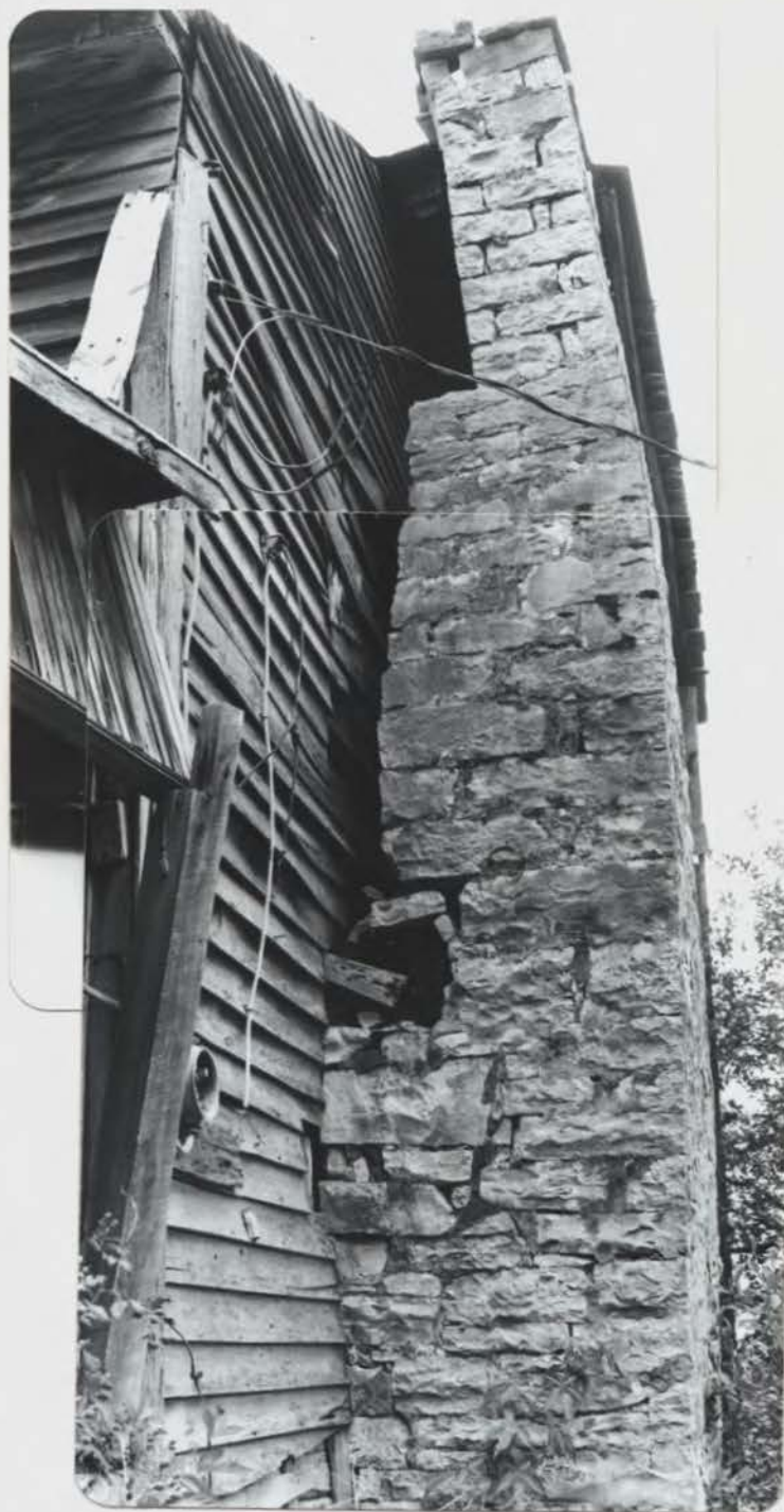
SOUTH VIEW OF CHIMNEY SHOWING ARCH LOG MARKING HEIGHT OF FIREPLACE
