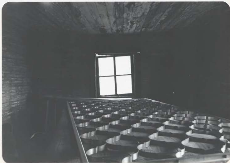
INTERIOR VIEW OF 1ST ADDITION TAKEN FROM DOOR OPENING ONTO PORCH
