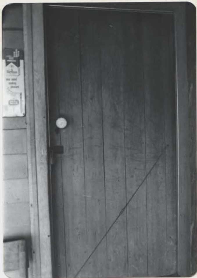
MAIN DOOR WITH SCREEN DOOR OPEN
