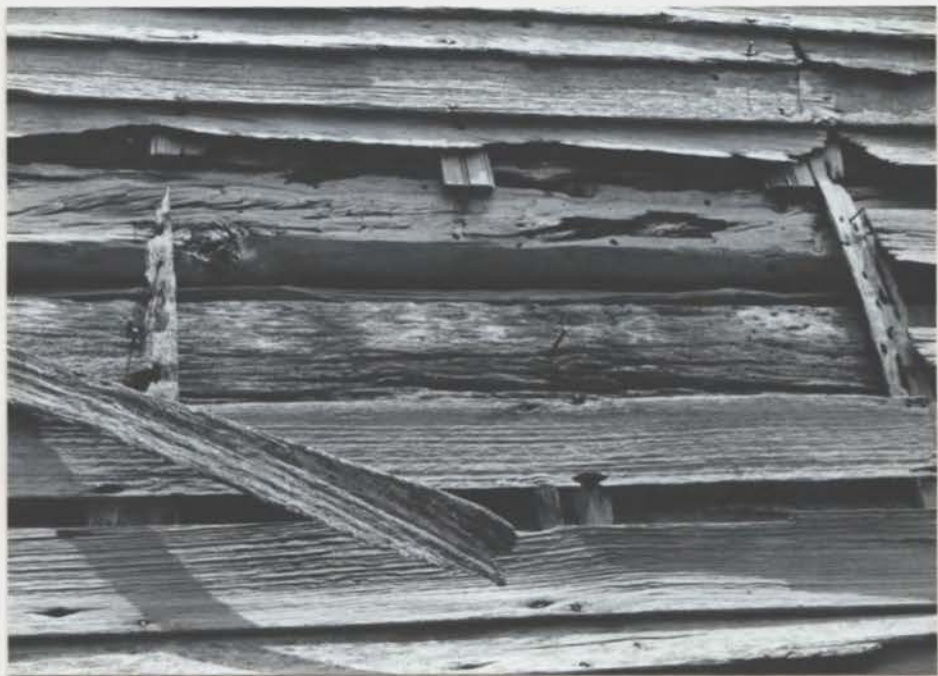
CLOSEUP OF SIDING ON WEST FACADE OF CABIN
