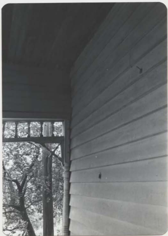
SOUTHEAST CORNER OF PORCH SHOWING JUNCTION OF SIDING AND RAILING
