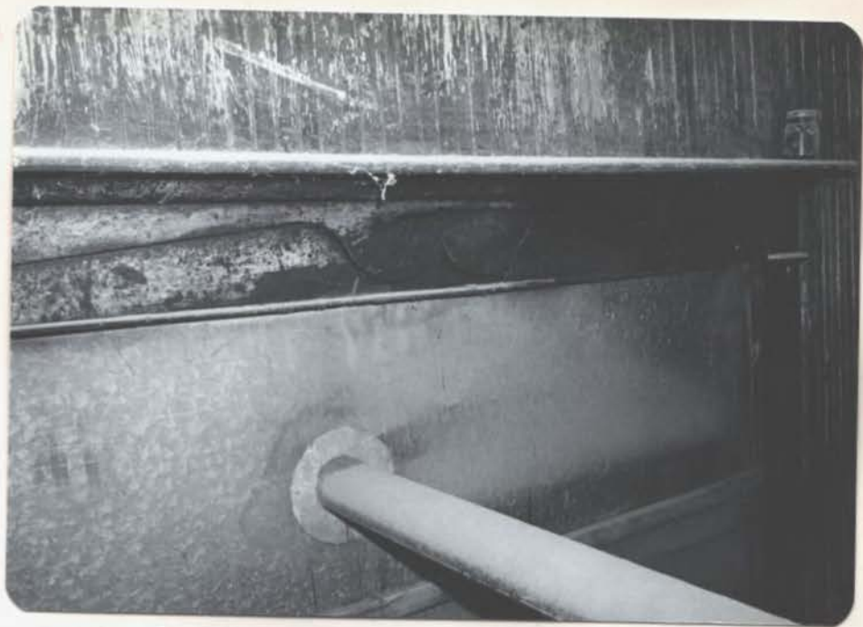
DETAIL OF MANTLE SHOWING ORIGINAL CARVING
