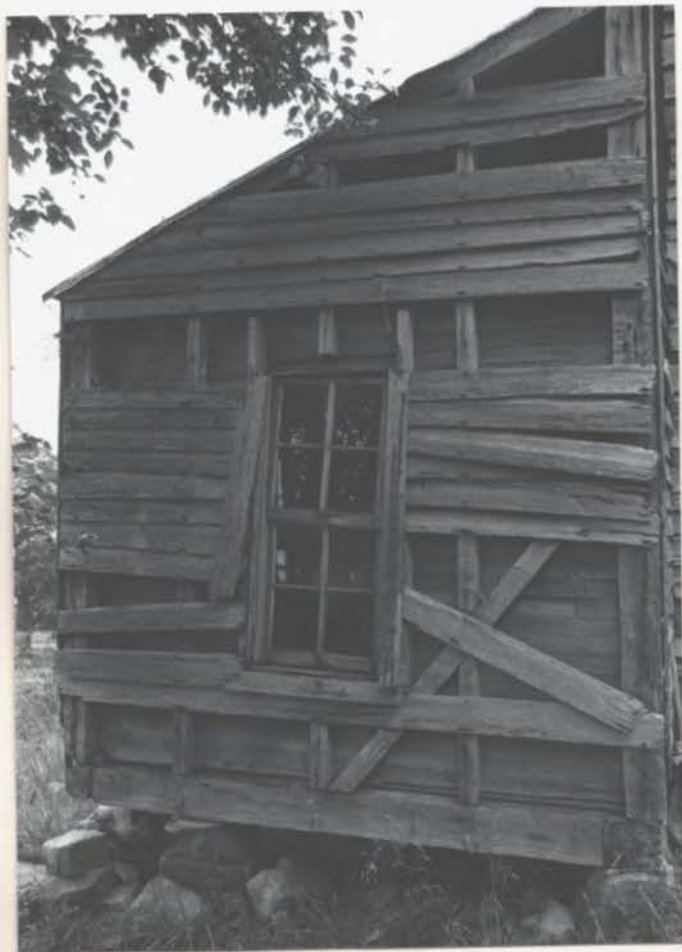
WEST WALL OF FIRST ADDITION
