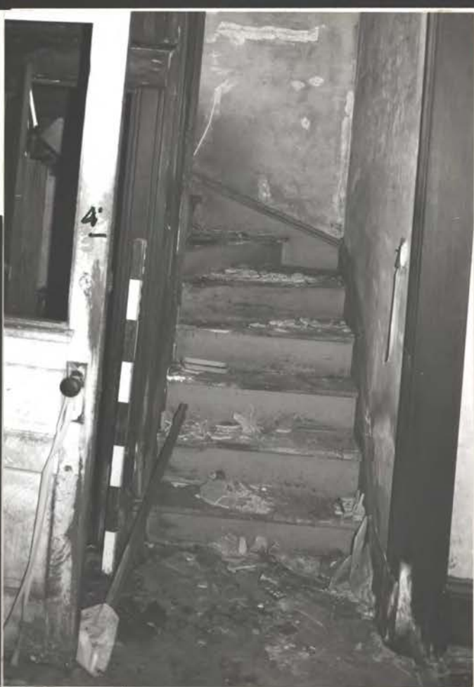
← Back Stair at fl. 1
