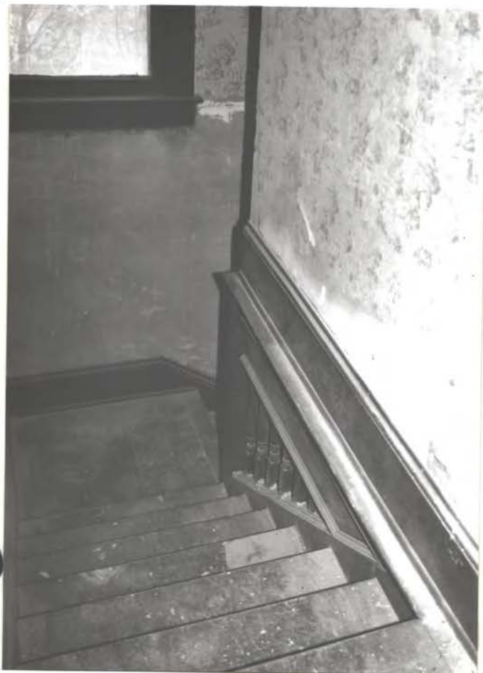
7 of 9 Front stair at fl. 2 ←
