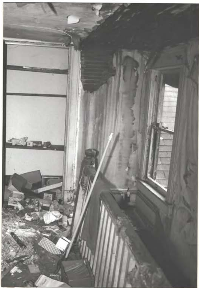
Back Stair at fl. 2 →
