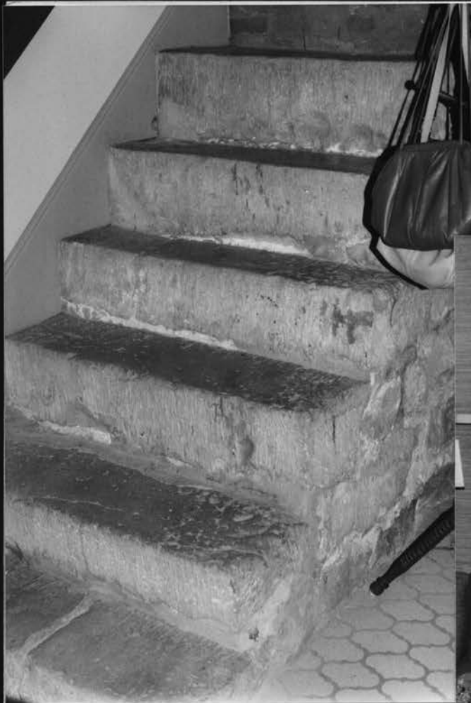
hand-chiseled limestone \nearrow AM steps from 1970's addition up into orig. hse. remnant rms. These steps were originally outdoors.
