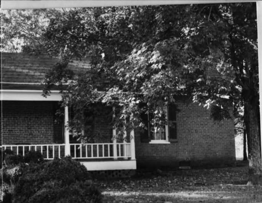
↳ 2x4 balustrade is 1980's, incorrect
