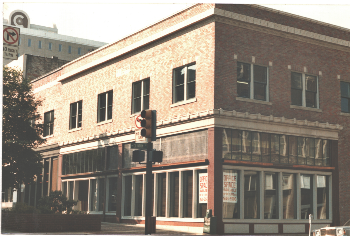
← c. 1918 Hutcheson Howard Street + 1986 Renov. for Law Offices by Jones & Herrin, Arch. (A Jones)
