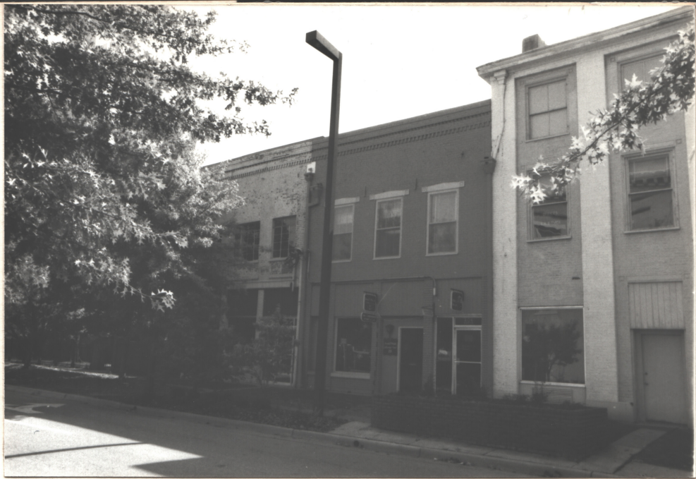
Photo 1 Looking S.E. Kaufman Store in center.
