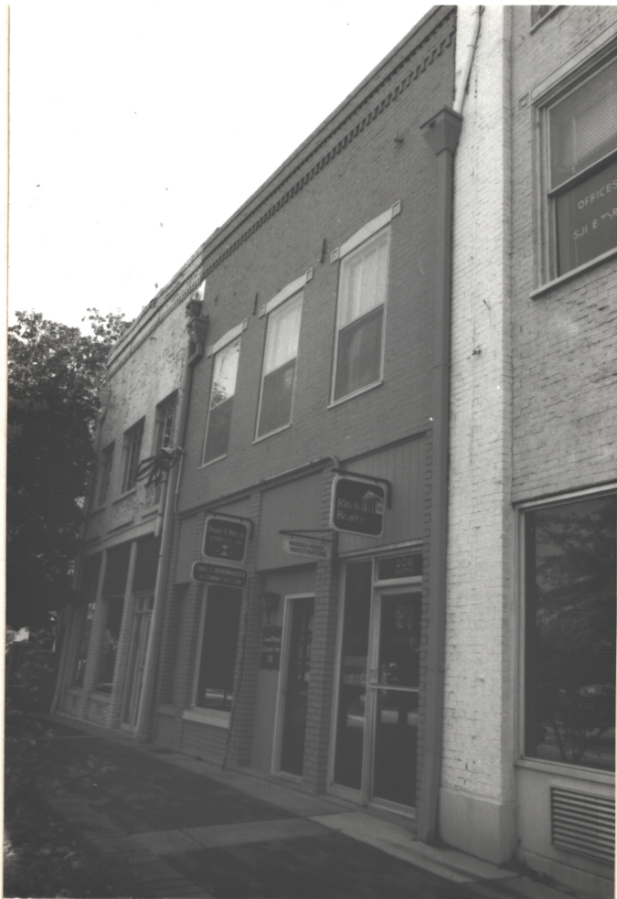
Photo 2 Looking E.S.E Kaufman Store in center.
