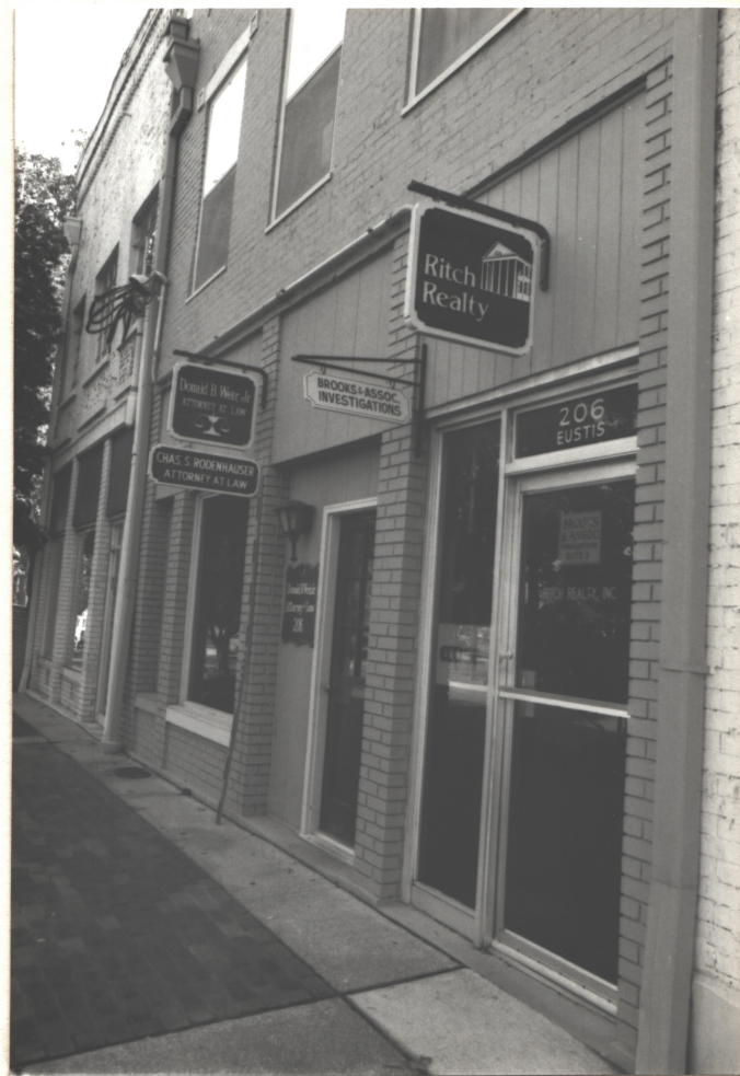
Photo 3 Looking E.S.E at ground floor. Clerestories are boarded over.
