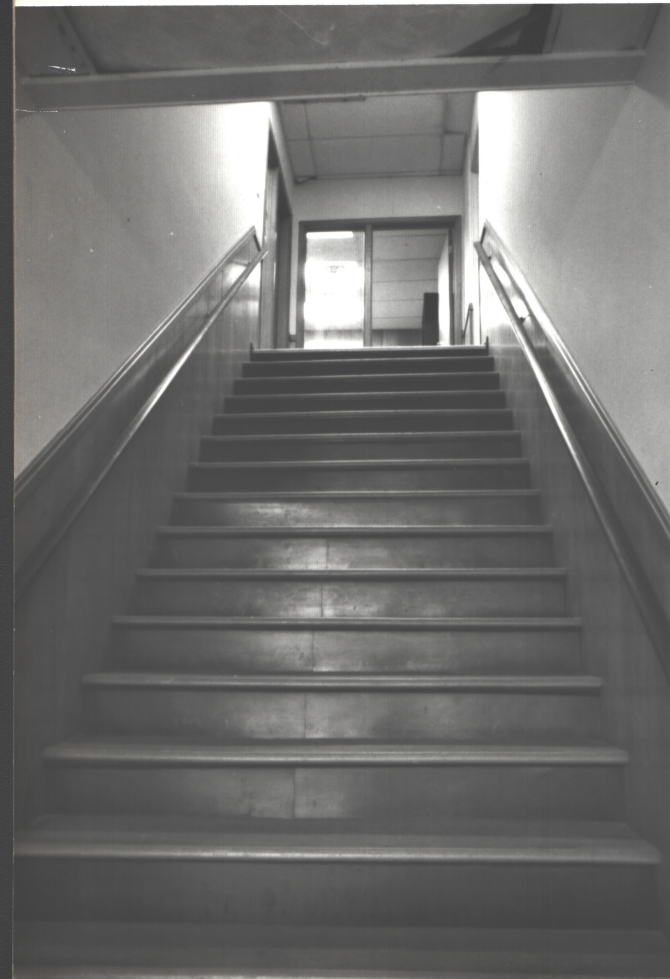
Photo 5 Stair to 2nd floor.
