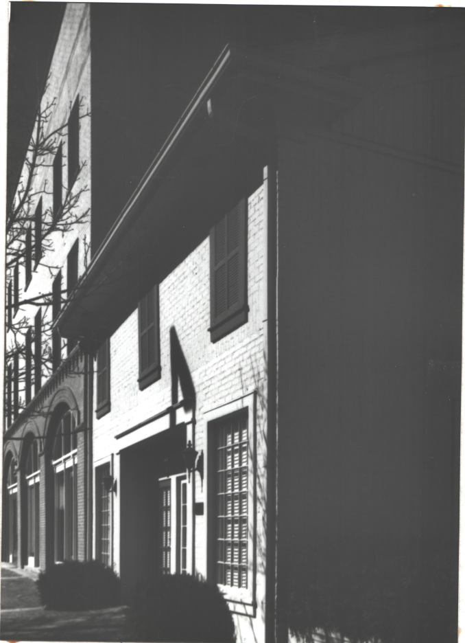
Off. remodeled from a plain box bldg. abt 1940 for Corp. trans. & Jones & Herrin Arch, c. 1960 (HJ)
