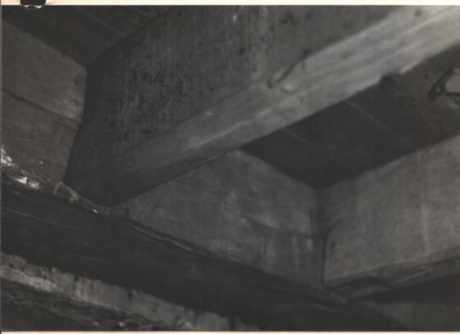
1st fl. S.E. Corner - brace is mortised + pegged
