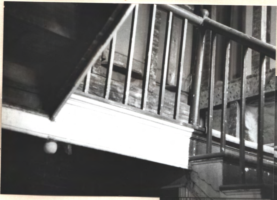
STAIR W/ PLASTER REMOVED = TYPICAL FED. TYPE
