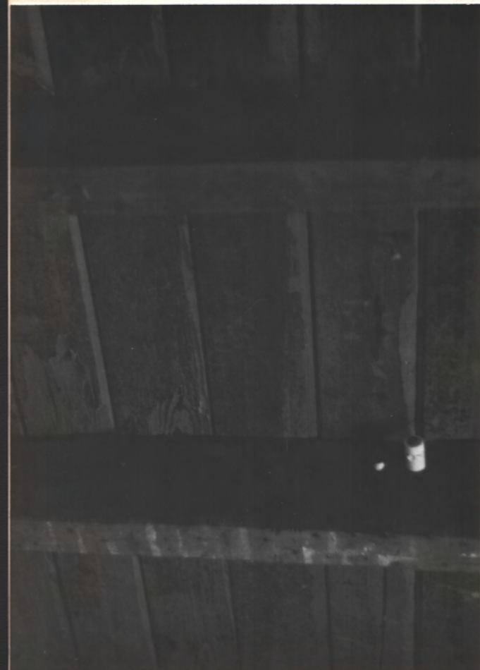
SASHSAWN FL. PLANKS, 5/4 x 6 JT + G BASEMENT
