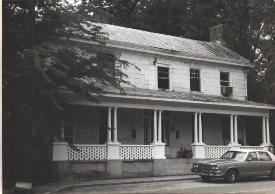
PORCH = 1920'S LOWER DOORS + WINDOW TYPES = 1920'S (8/12 UPPER SASH IS FED)
