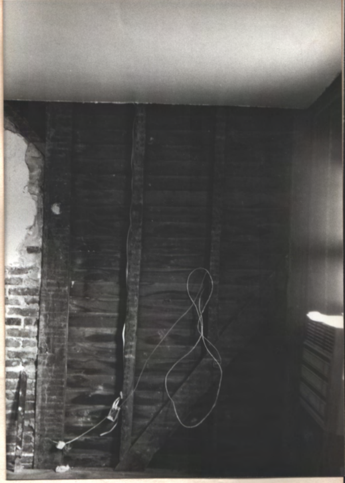
2nd fl. S.E. Corner brace
