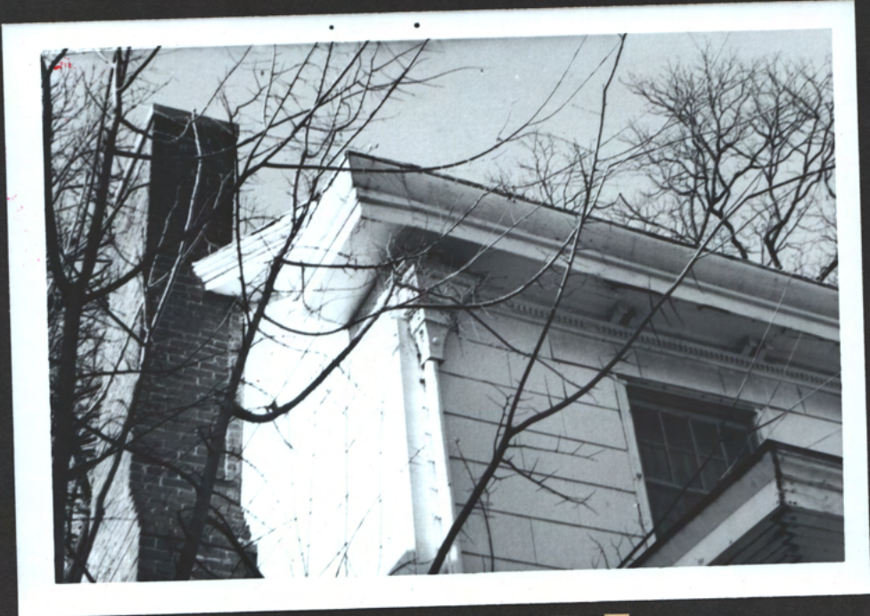
CLAPB'D UNDER CEM. ASBES. SIDING PORCH & 1ST FL. SASH = LATER. MOVED HERE IN EARLY 20TH CENT FROM 1 BLOCK WEST
