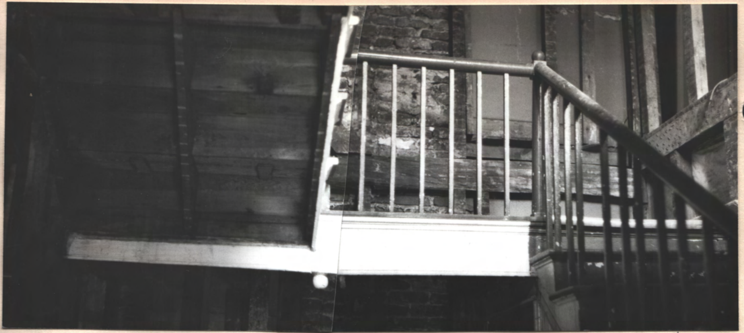
STAIR W/ PLASTER REMOVED = TYPICAL FED. TYPE
