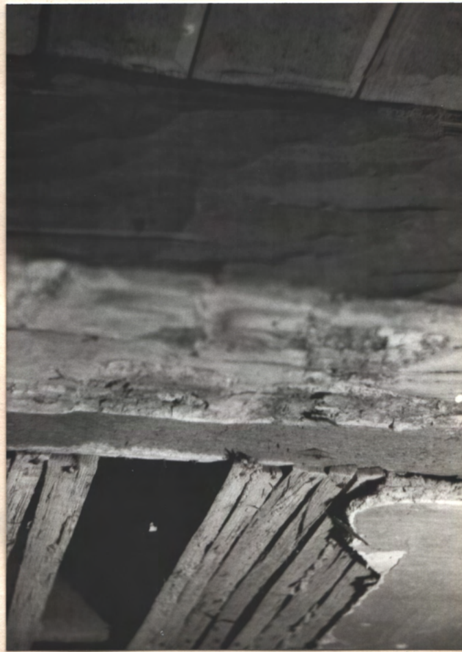
HEWN + PITSAWN JOISTS SPLIT LATH, HAIR-PLASTER
