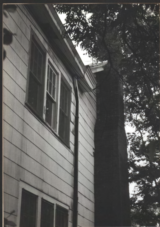
WEST SIDE 1920's → FED. MODERN ASPBESTOS SHINGLES OVER ORIG. CLAPBDS
