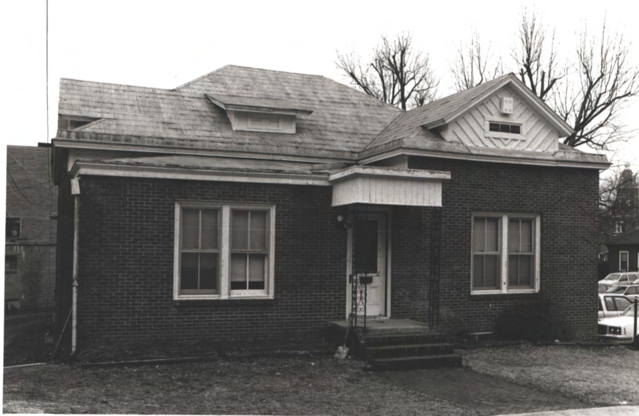
MAKESHIFT VIEW (1996) AFTER THE C.1960 BRICKS WERE WRAPPED AROUND THE HOUSE AND PORCH. THIS VENEER IS EASILY REMOVED TO RESTORE THE C.1894 DESIGN.
