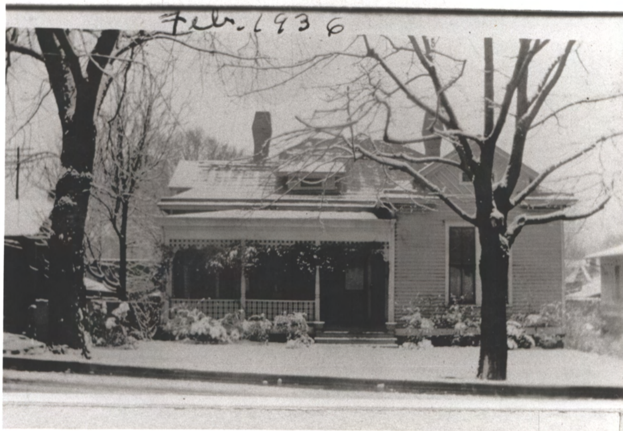
ORIGINAL APPEARANCE BEFORE C.1960 BRICK VENEER WAS WRAPPED AROUND THE HOUSE AND PORCH
