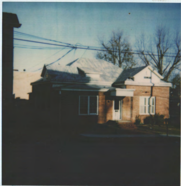
EXISTING VIEW WITH MODERN BRICK VENEER
