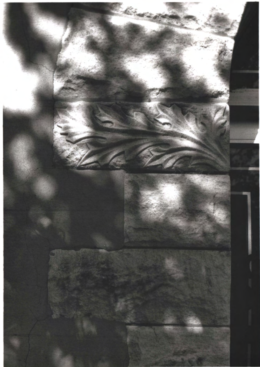
S. side entry arch (c.1905)
