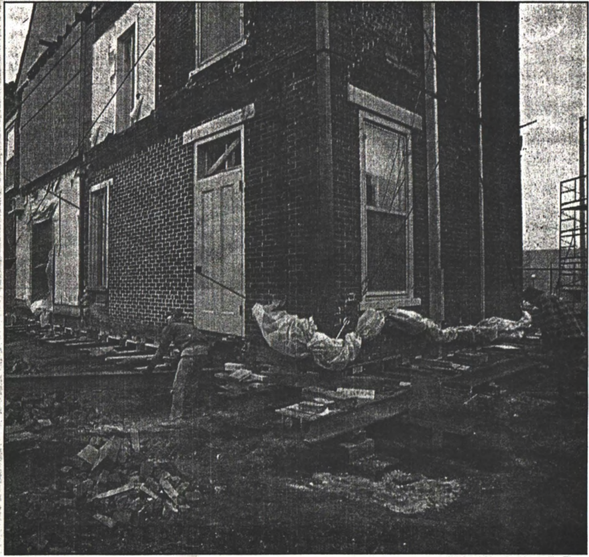
Employees of the Hollis Kennedy House Movers company prepare the Humphreys-Rodgers house for its move.
