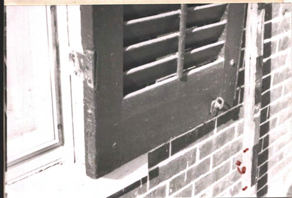
Exposed tenon-ends of posts at glaze
