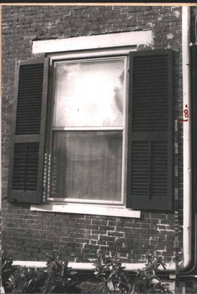
Sash at S. front, W. Rm (pre 1841, was 9/9 Gl. Rev., mortar cut out c. 1900. See pg. 35
