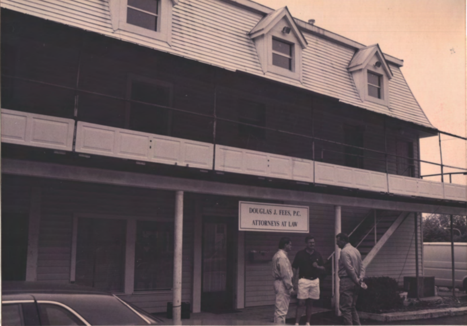
1980's St. Clair Bldg.
