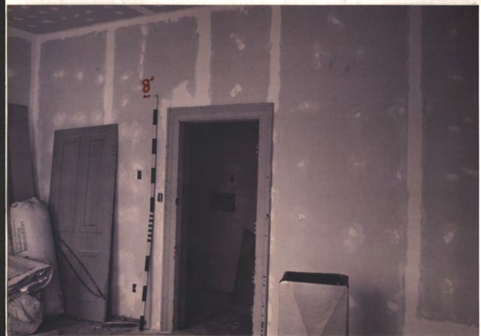
door to hall N. WALL
