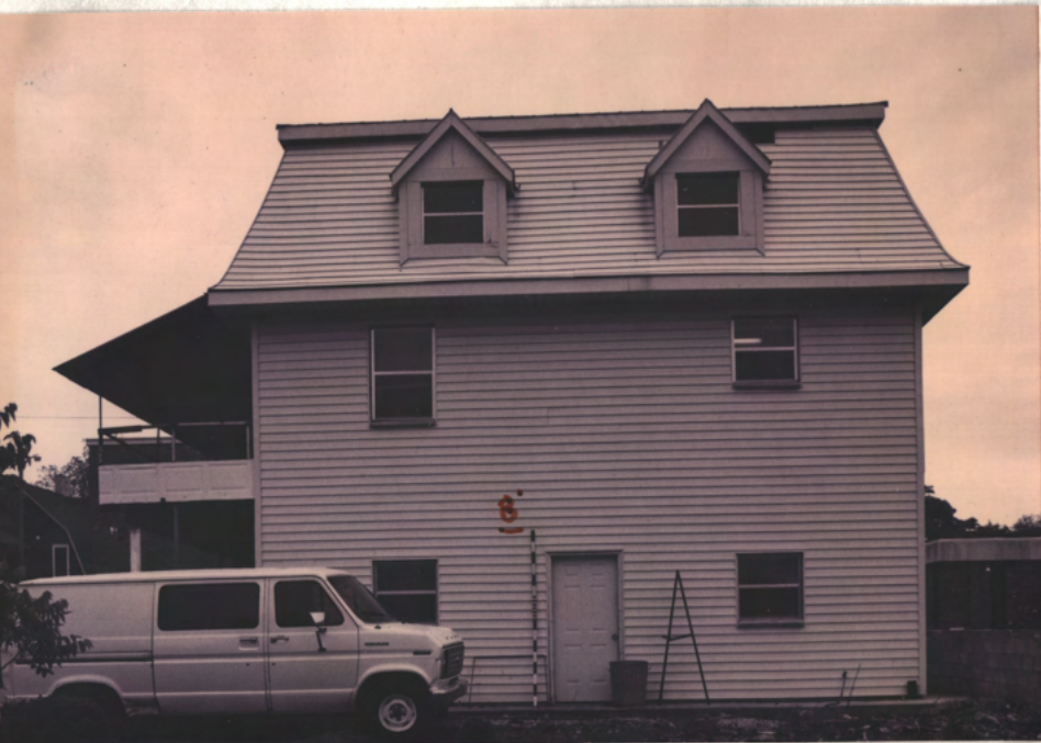
← N West fac. of St. Clair Bldg.
