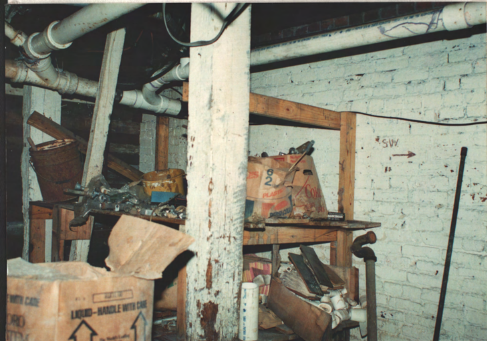
Rm. S. of N.E. Entry (look S.E.)
