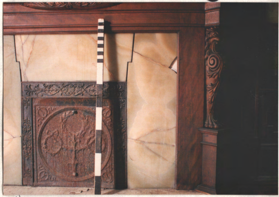
N Note missing piece
