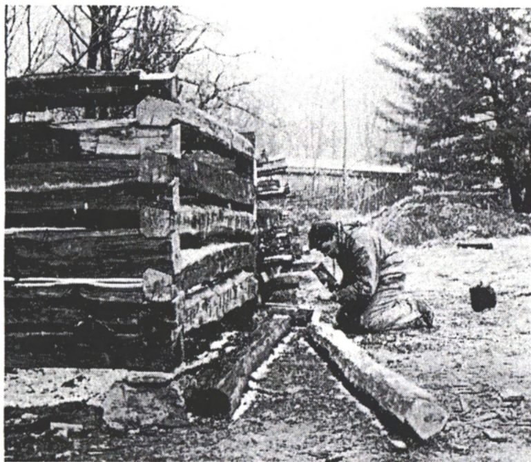
Curator of History Charles Pautler, chiseling corner notches on the corn crib in the snow, March, 1993.
