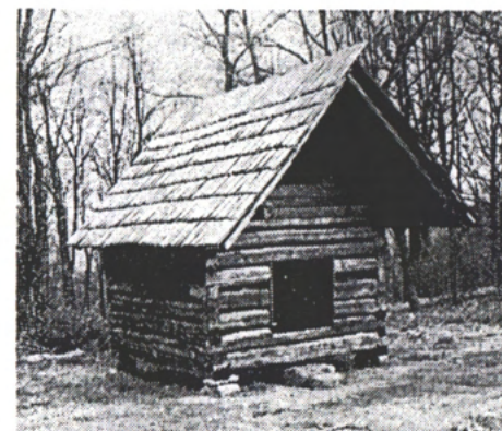
The finished corn crib, built by volunteer staff. Note the hand-riven oak roof boards. January, 1994.
