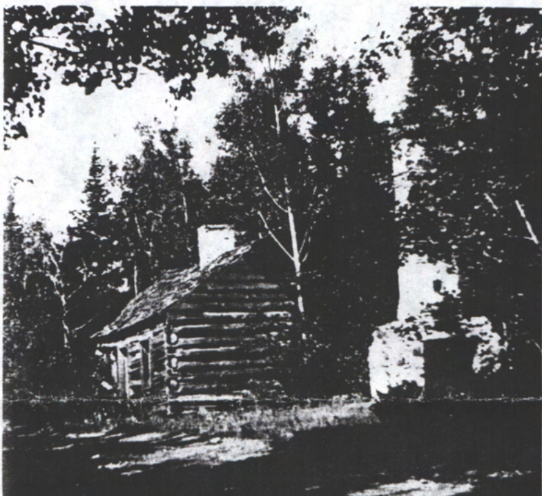
Figure 10. Taken in 1910, this photo shows the remains of the married soldiers' quarters at Fort Wilkins on Copper Harbor in the Upper Peninsula of Michigan. Built in 1844, the double room log house is characterized by huge round logs saddle-notched together and a central fireplace. A fireplace and chimney in the foreground are the only remains of an additional log building. Silver gelatin print, photographer unknown, courtesy of the Neville Public Museum of Brown County.
