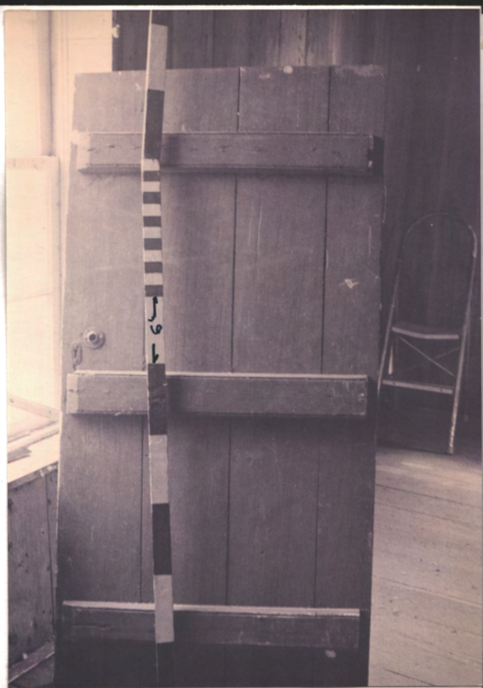
Stair door (detached) - good work. Apparently original or early (since planed wood)
