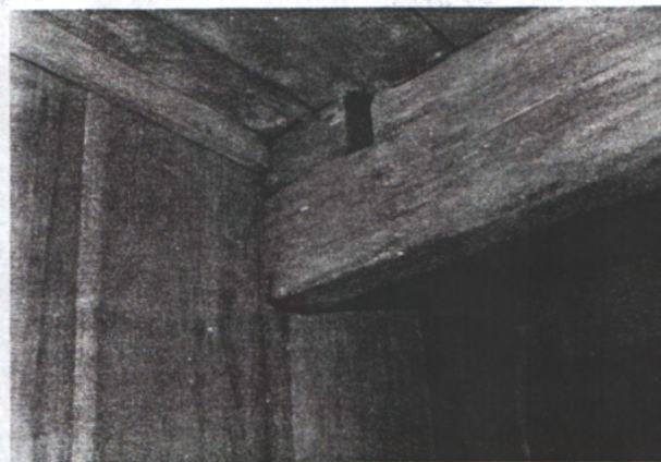
Re-used floor joists, June, 1994. Photograph by the author.
