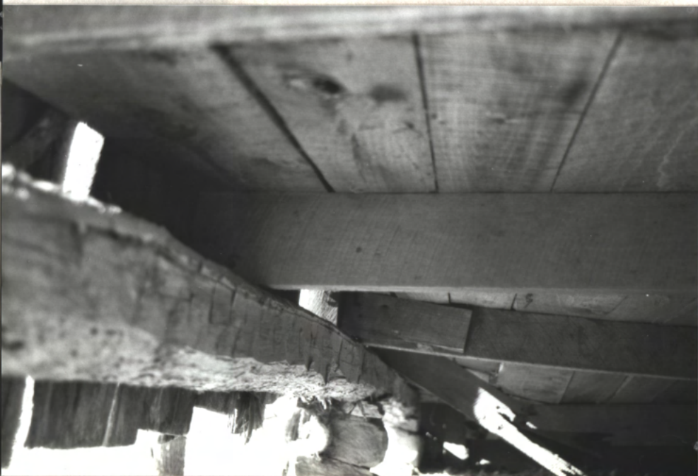
Under B.R. ♀ = all rotary sawn (post C.W. War) & small dimensions
