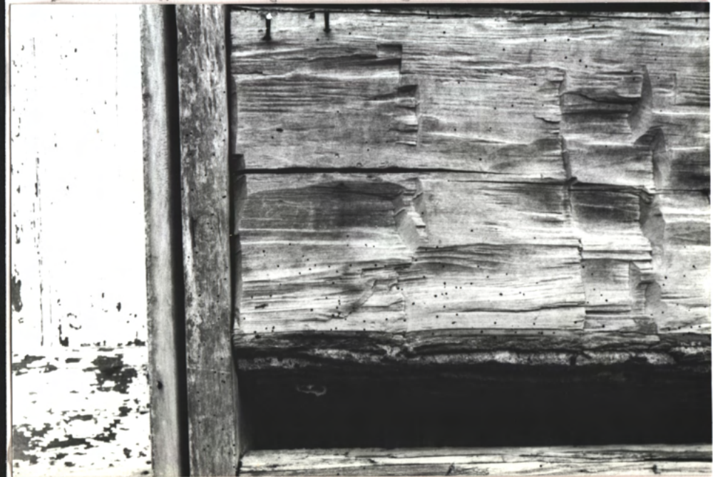
↑ door at rt. ↓ door frame
