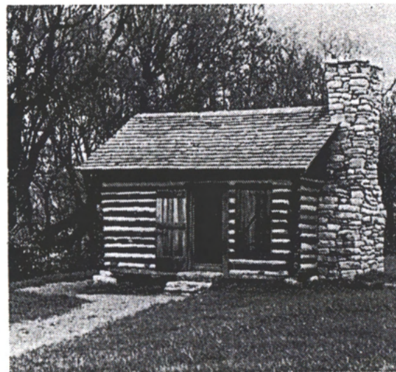
The Gardiner Cabin soon after restoration. Note the stacked rock limestone chimney. April, 1991
