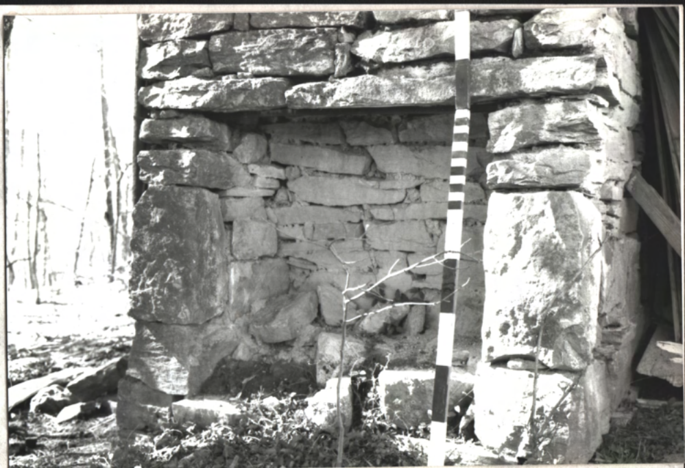
KM. fireplace (room gone) → N Note 90° sides + ±4" w. = typical of cooking fireplace
