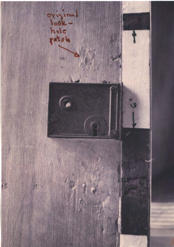
Stair door (detached) - good work. Apparently original or early (since planed wood)
