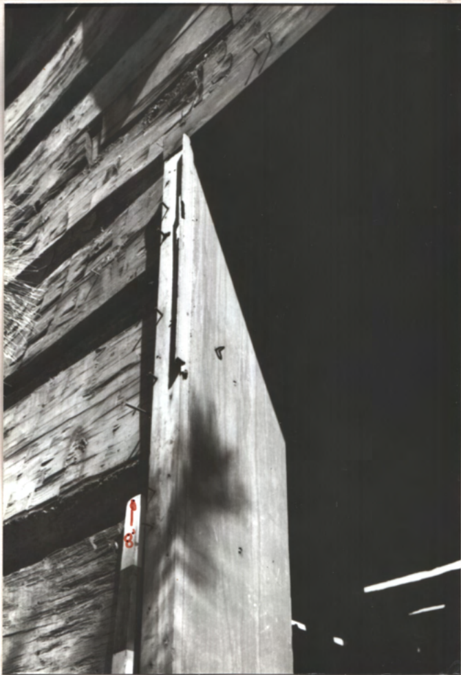
Door joints of head at orig. center door
