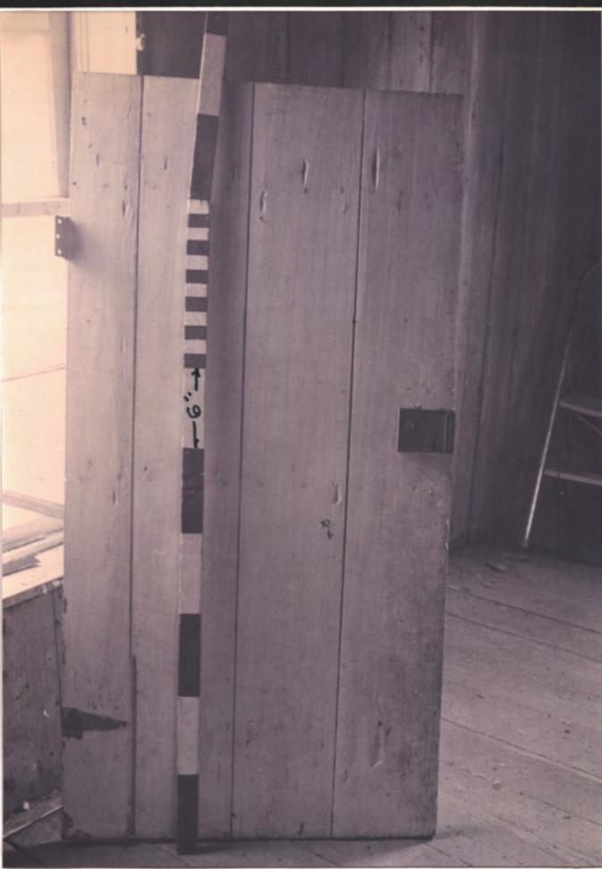
Stair door (detached) - good work. Apparently original or early (since planed wood)
