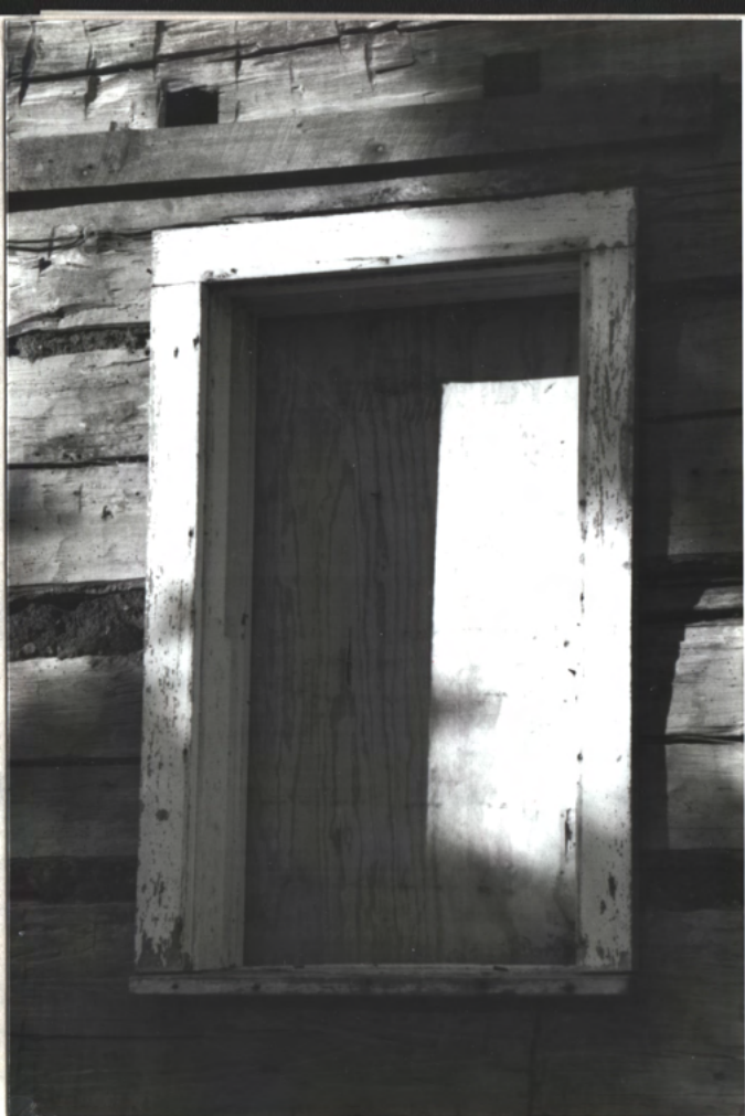
S.W. window (E. pm) (would have had backband like window at rt.) →
