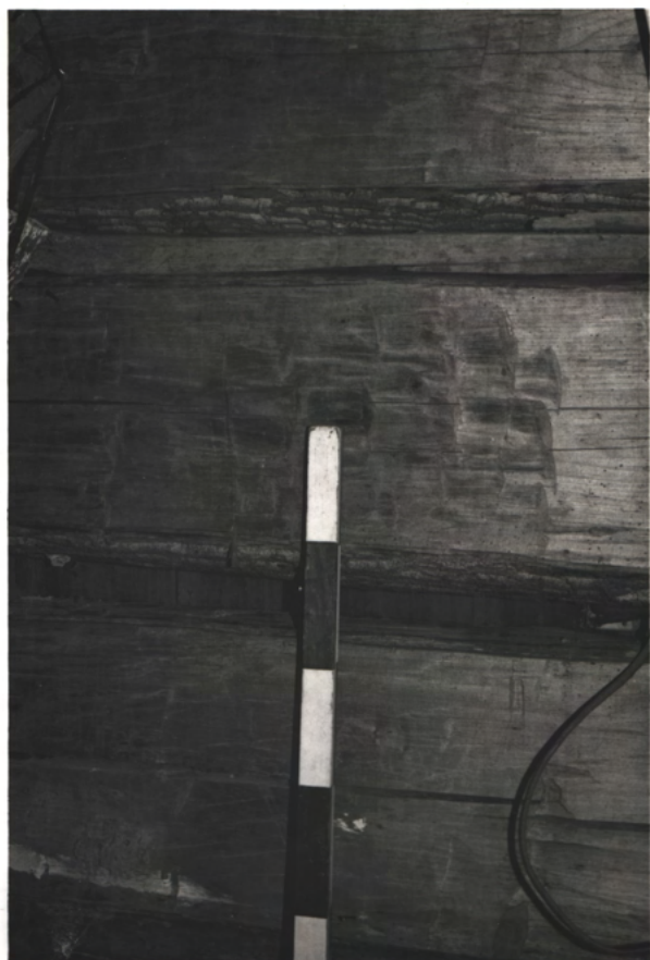
Logs ( \pm 16-18'' h.) bark still on (not unusual) Ads or ax marks
