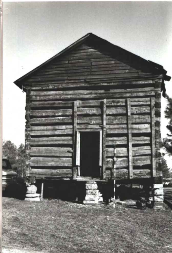
N ← ↑ Later W. door. Was a window. Note door opening. CURTS SIM-log
