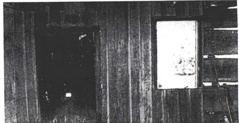
Paneling in the parlor of the Meals house after cleaning. Note the original door and window as well as board and batten door with cut-out for electricity hookup. The window sash and glass have been removed during the restoration. All paneling is tongue-in-groove with a double-beaded edge on each side. 1994
