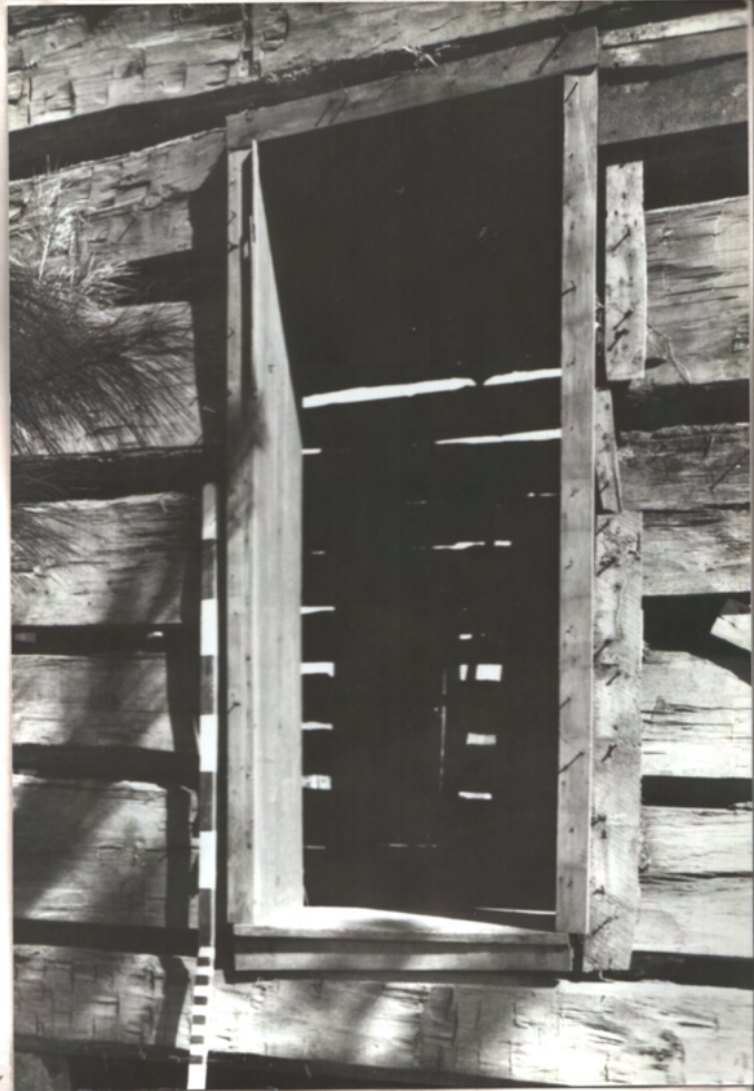
Orig. center door (later rotting - same sub-frame)
