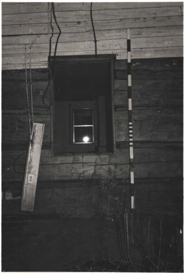
Sash opening at N. Wall, west end
