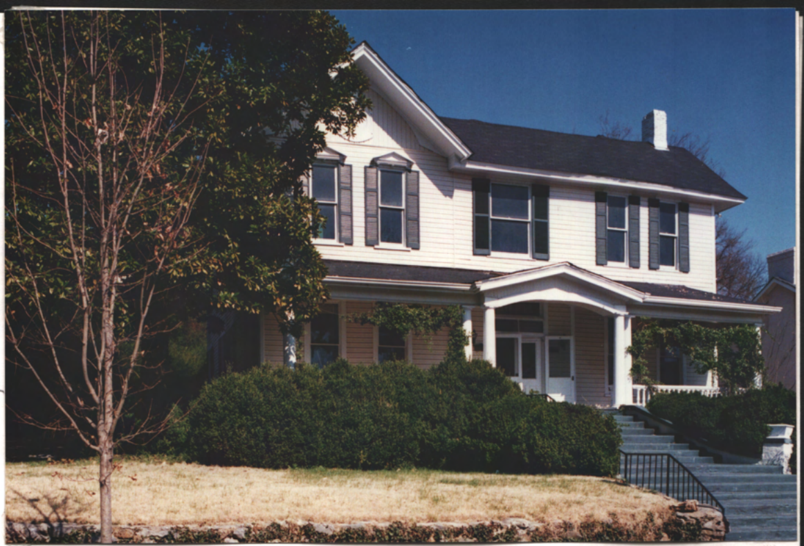
1893 "Gray Gables", 509 Adams St., Huntsville, AL (Front altered 1916 after a fire in the front center bathroom, fl. 2, for news paper account) Porch & steps & 1/1 bushes look 1916. There may have been more gables on front, based on the name of "gray gables"
