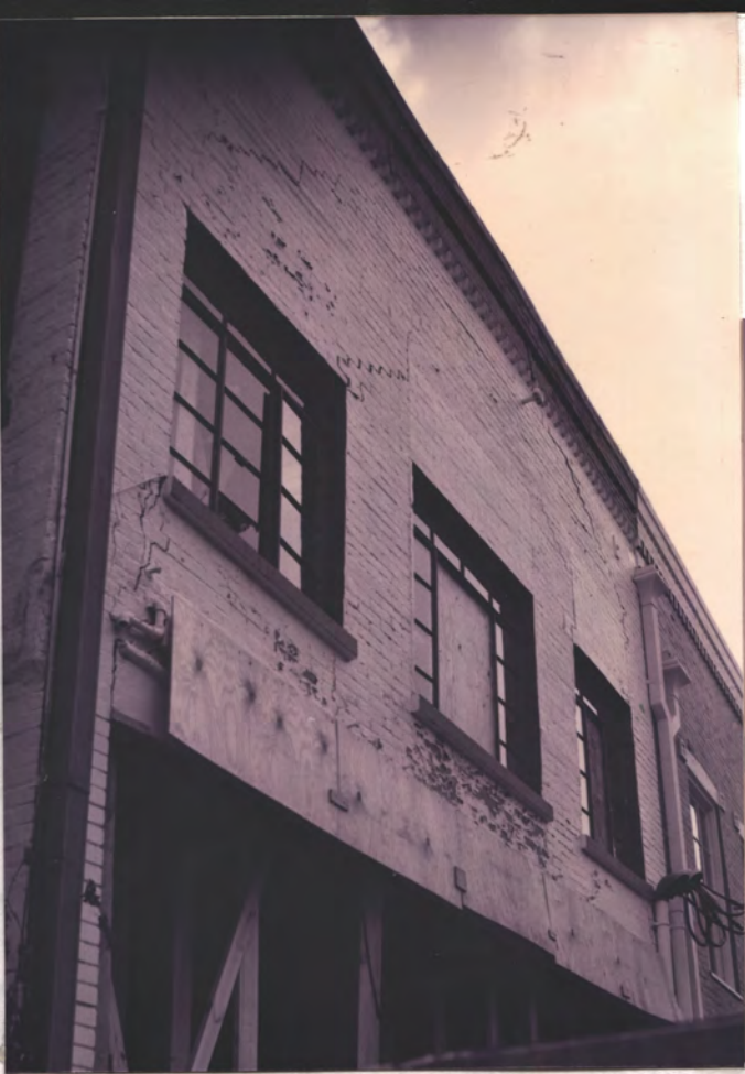
Wall not resupported securely before 1950's cols were removed. Dropped \pm 3'' & cracked
