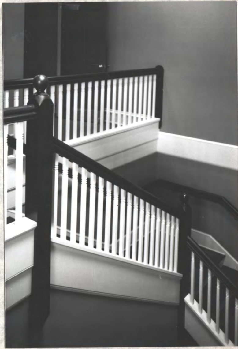
new Stair at fl. 2, HJ design per c. 1870 example
