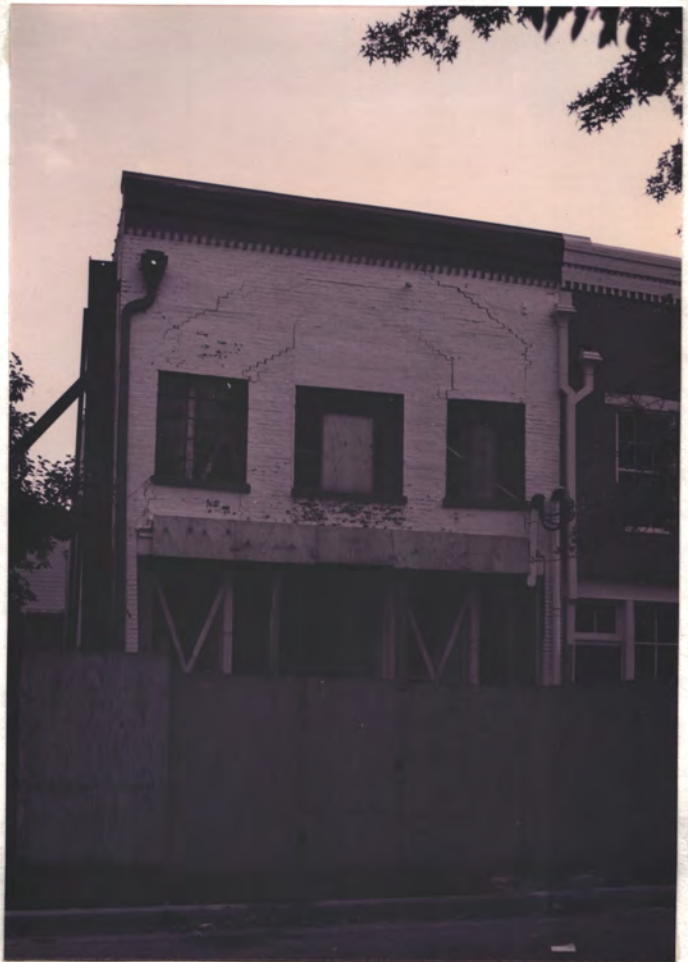
Note cracks & \pm 3'' sag in wall
