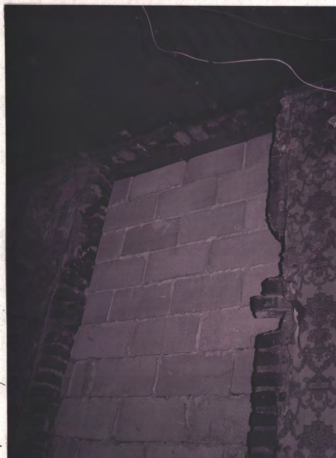
orig. window made into a door
