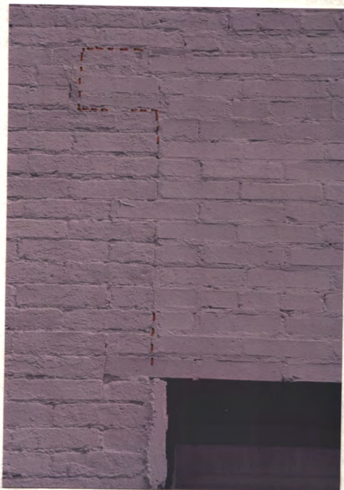
Top Center Sash head
