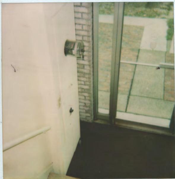
Elev. entry of SW INSIDE entry (no alarm)
