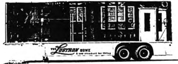
Lustron components were carefully loaded onto a flatbed truck for delivery to the building site. Assembly took approximately 350 hours. (Ohio Historical Society)
