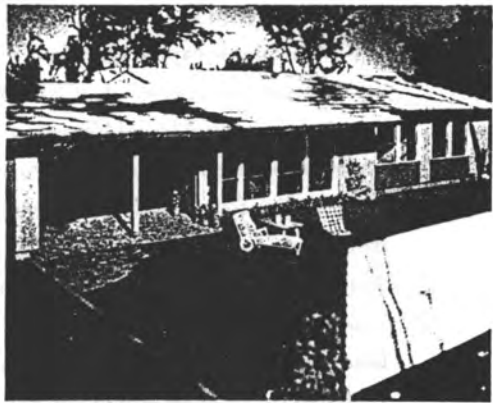
Model of Carl Koch's revamped Lustron house, which was never built. Standard panels were increased to two by eight feet, joints were concealed, and window units were simplified. (Carl Koch)
