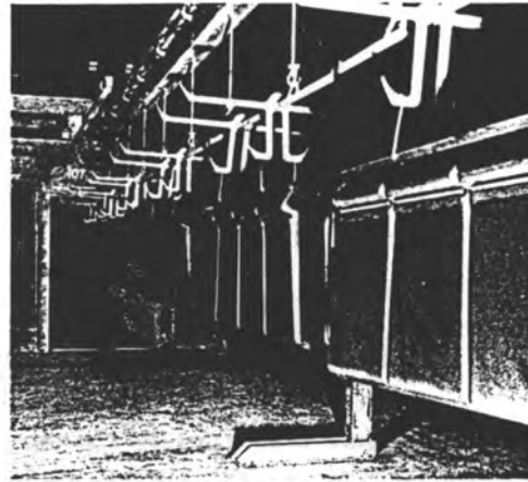
Metal panels emerge from the drying ovens in this interior view of the Lustron plant. (Ohio Historical Society)
