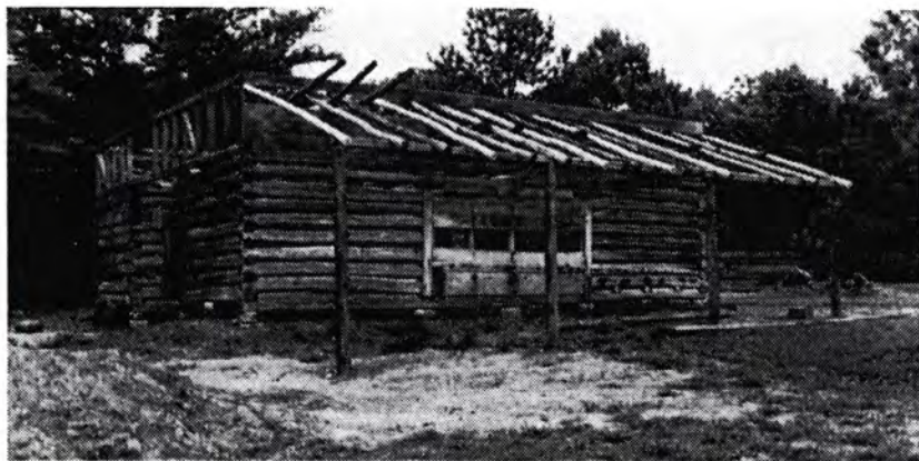
Barn in progress, 1993.
