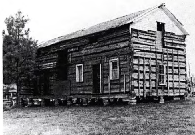
Above: James A. Meals house on site at Burrirt Museum. The clapboard siding has been removed to determine which logs need to be replaced. 1994.
