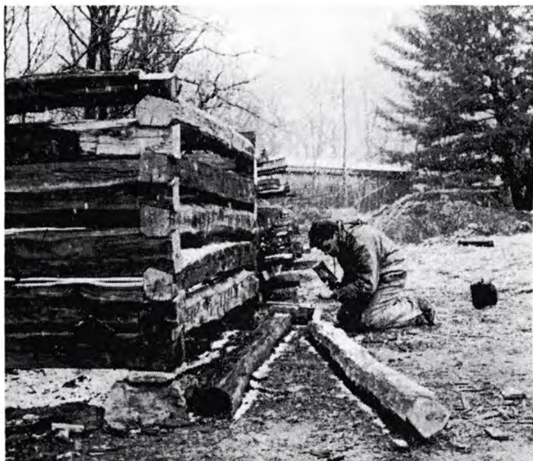
Curator of History Charles Pautler, chiseling corner notches on the corn crib in the snow, March, 1993.
