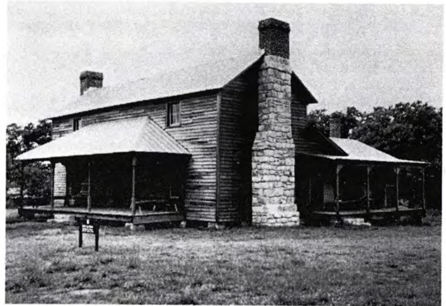
The Samuel Balch House soon after completion, 1992. Note the 1898 rear kitchen addition.
