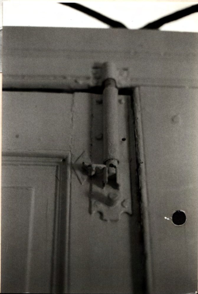
orig or entry door bell (see pull-knob on photo at left)
