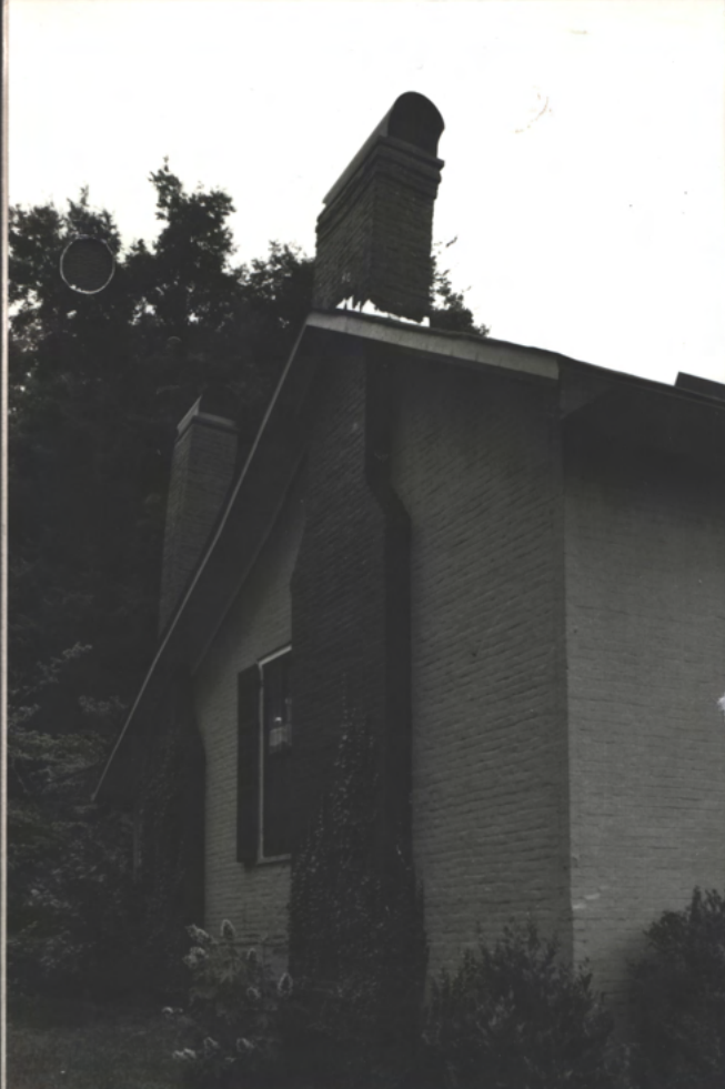
N ← Note bowed chimneys N ← = typical of 150 yrs +
