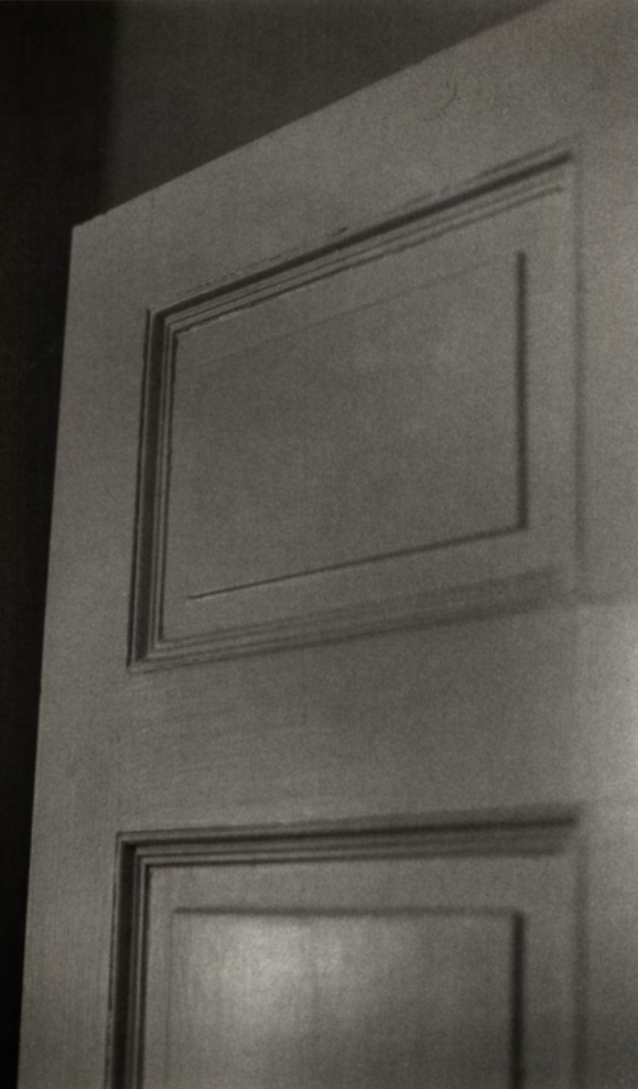
"front" (hall side) of door
