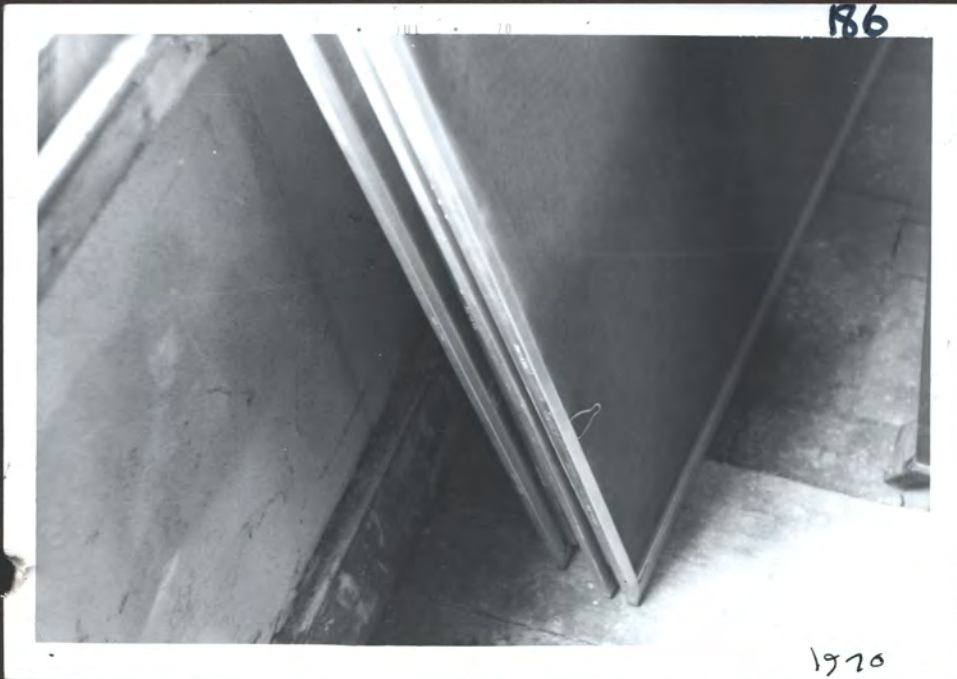
2ND FL (SERVANTS) BEADED BASE, WINDOW SILL (STORED SCREENS = MODERN)
