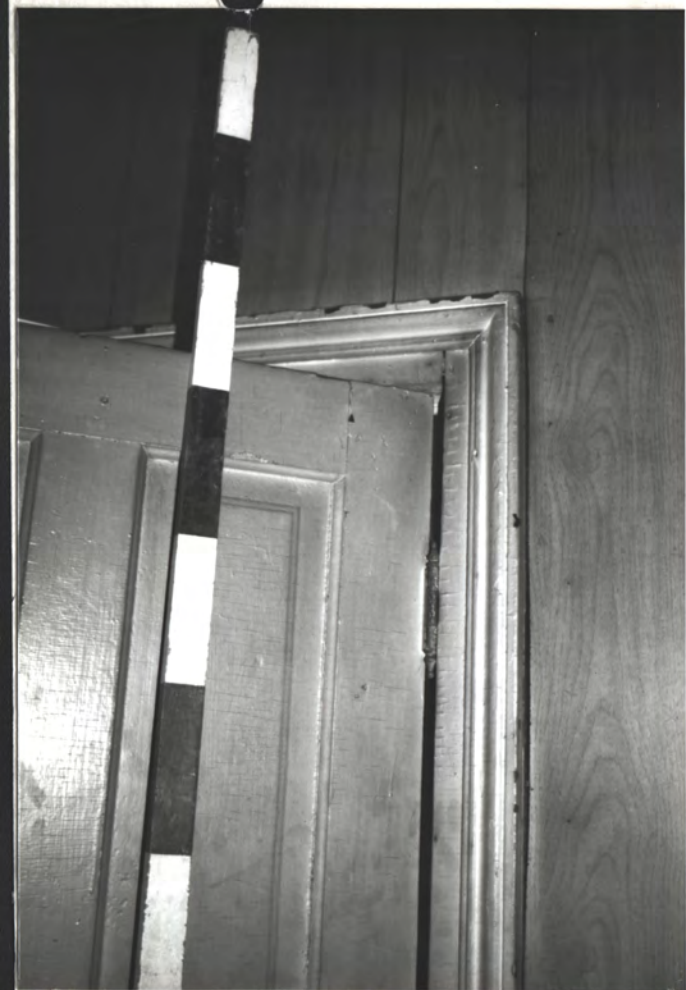
1888 door & frame at Parker to space below stairs
