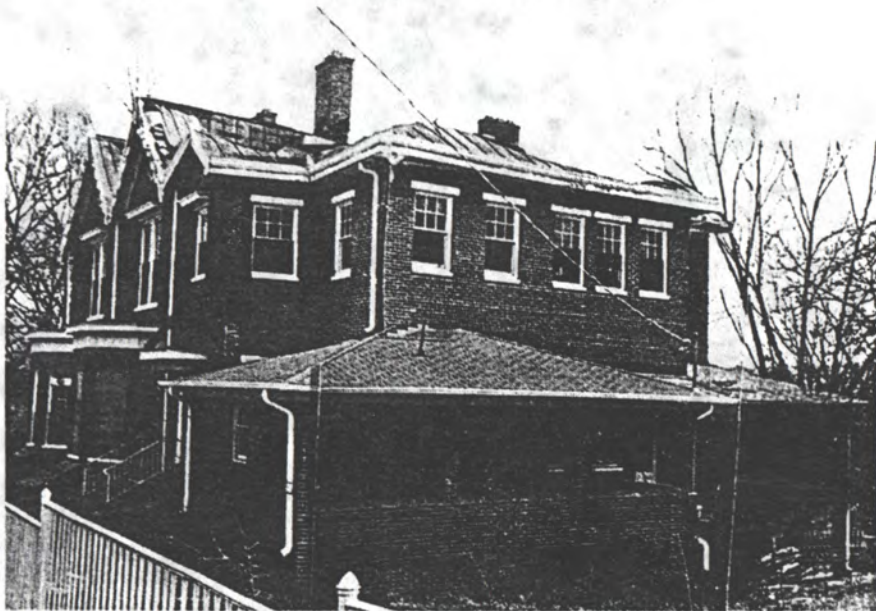
BEFORE Picture taken in 1974. Includes a 1960s carport and kitchen addition. (Taken after the 1973 fire.)
