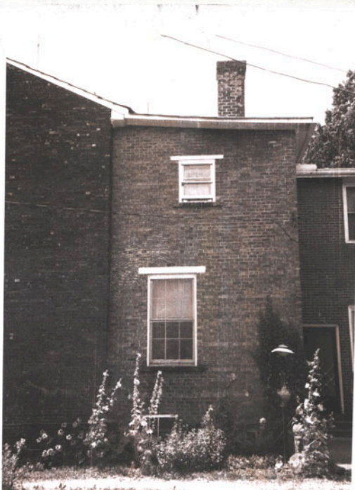
20th. cent. ↑ NW cor. of N.E. (reused 1830's sash at addn 1st fl.)
