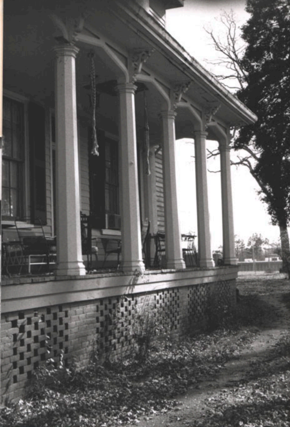
N → WEST SIDE PORCH
