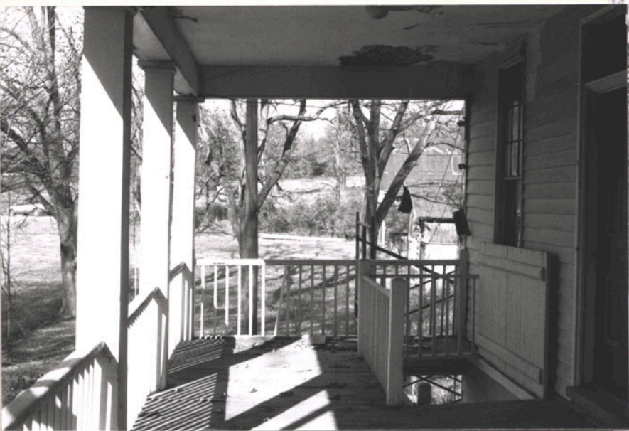
Serv. bldg stair - parts apparently reused from removed stair at main house (see pg. 6 sketch)
