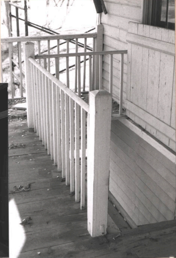
Serv. bldg stair - parts apparently reused from removed stair at main house (see pg. 6 sketch)
