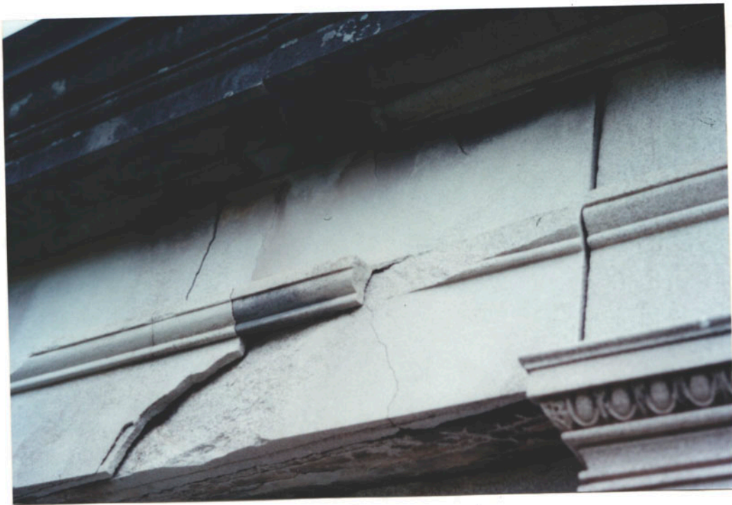
Before (freeze-spalls)
