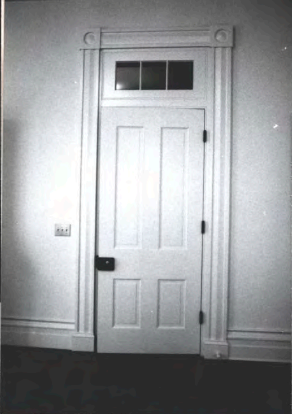
Door to hall (replicated 1848 door + lock. All trim & frame = orig. Transom = Replic)
