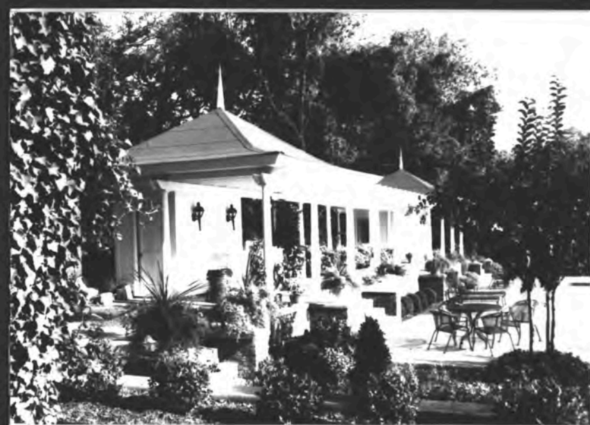
← OLD PAVILION 1980 - N Jones MIDDLE TOWER - EXIST. IN 1980 (1950's?)
