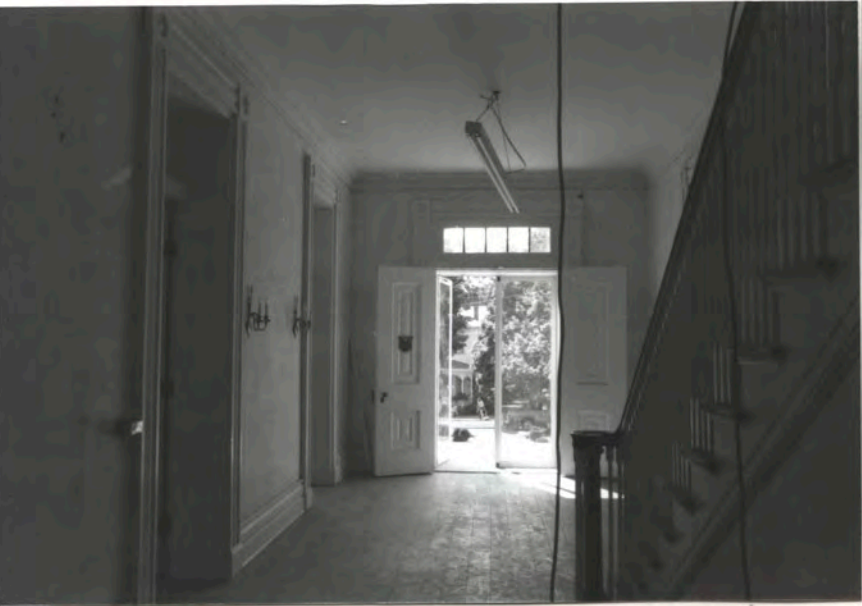
ENTRY + STAIR BALUSTRADE IS C. 1920'S "COLONIAL REVIVAL" STAIRCASE SAID C. 1925 BY HENRY CHASE
