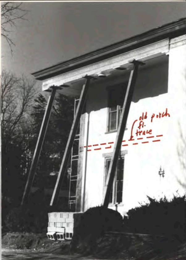
↳ Cols. take dn. to rebuild sunken porch fl. N ←
