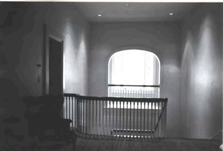
Looking east from 1848 Fl. 2 into 1989 gallery, Fl. 2 N.S.
