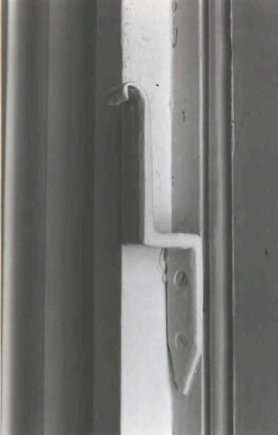
LATCH-BAR HOLDER (2x4 BD. BAR)
