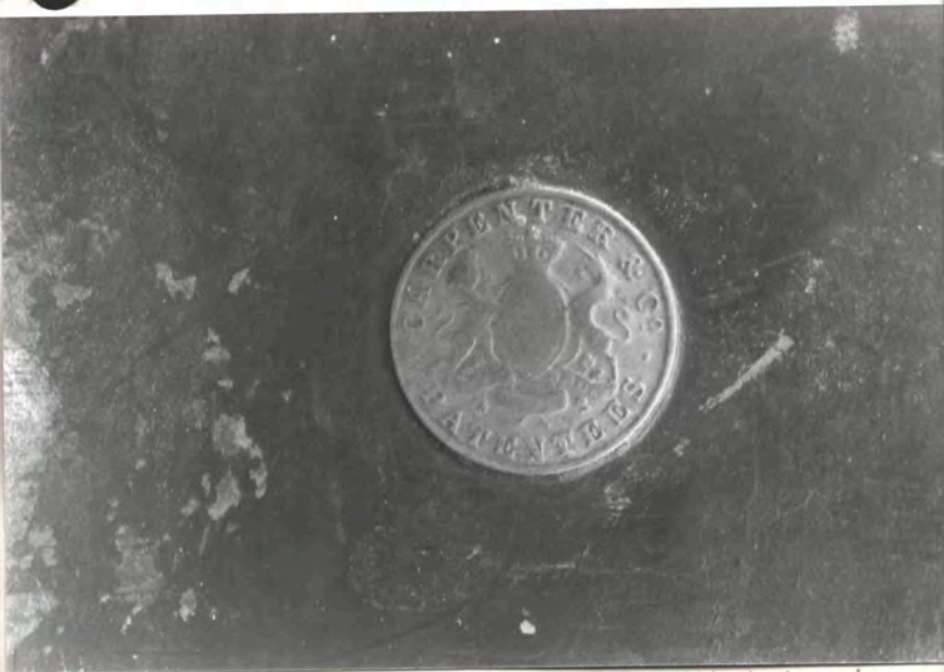
BOLTS TRADEMARK, \pm 5/8" \phi ENTRY HARDWARE ( ONLY ORIGINAL IN ENTIRE HSE)
