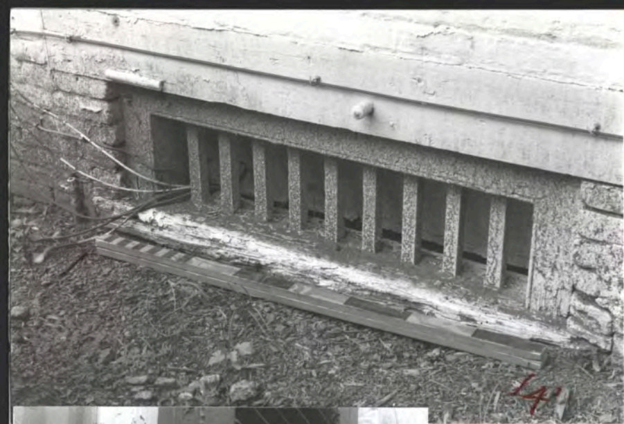
FOUNDATION VENT (TYPICAL OF 1800-1860) S. WALL
