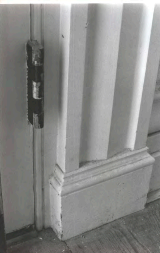
JAMB AT PLINTH ← ONE-PC. CAST IRON HINGE 1848 TYPE, TYPICAL
