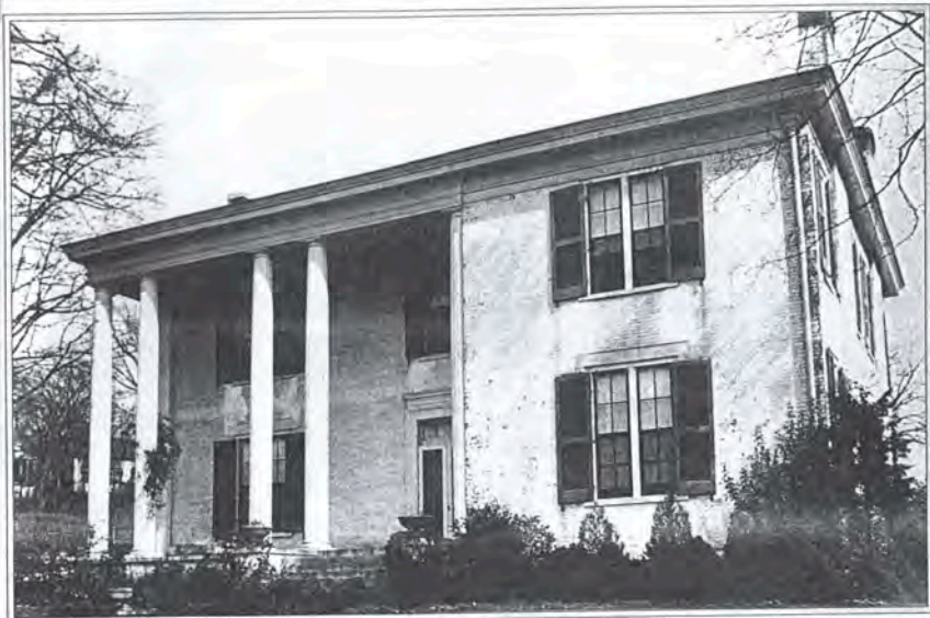
The house at 517 Adams Street, known locally as the "backwards house," was used as headquarters by General Mitchel during his occupation of Huntsville in 1862. According to legend, the prospective owner went to Europe on business and left his building plans in the hands of an uneducated overseer, who constructed the house facing the wrong way. Today, the house—now much enlarged—still faces the street from a recessed rear porch. Photograph c. 1934. (Courtesy Huntsville Public Library)
