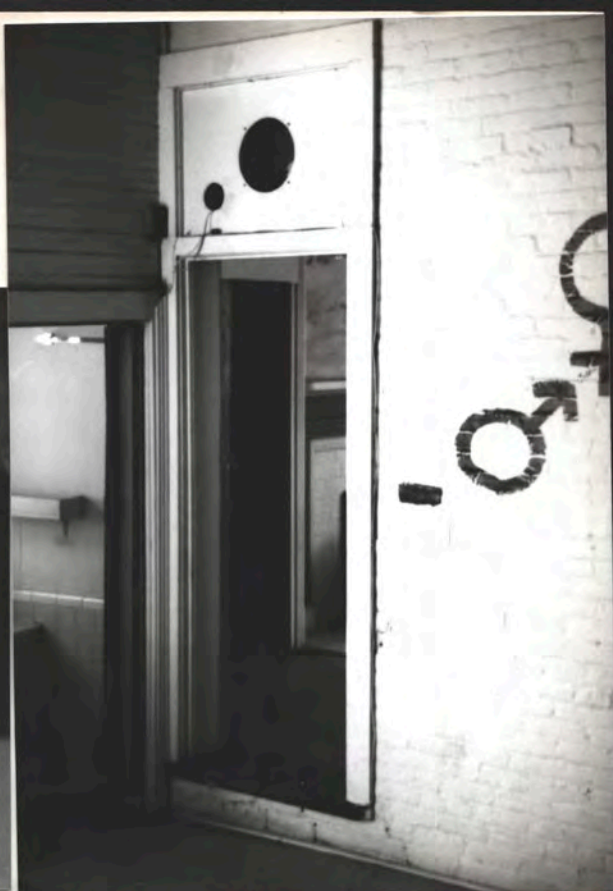
N ↗ Ø TO 2ND FL. N. E. RM 2ND FL. ENCLOSED PORCH
