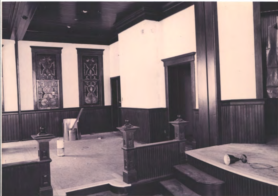
In the 1970's, the Bema (plat.) was enlarged to front, about 4'. Viewed orig. in 1994, & restored, as seen here, at urging of AJares.
