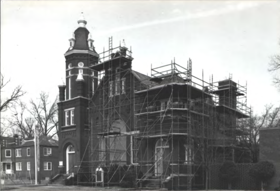
Restored - out gable, metal finish being replicated in painted copper (excellent job by "Coppersmiths") 3 Finishes at tower already repaired in this photo
