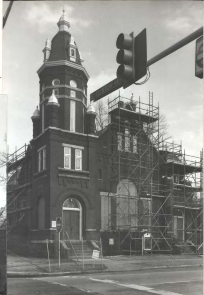
Restored - out gable, metal finish being replicated in painted copper (excellent job by "Coppersmiths") 3 Finishes at tower already repaired in this photo
