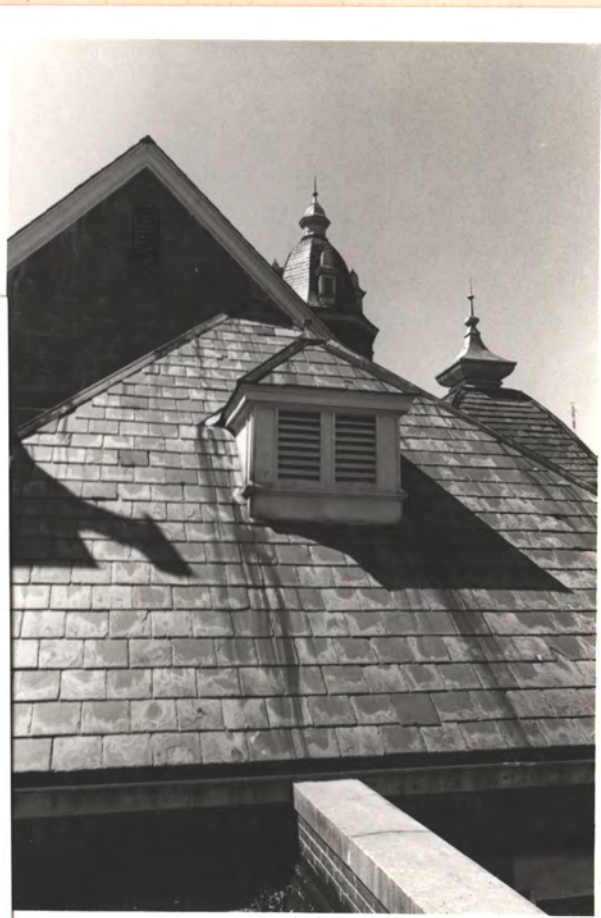
E. SIDE OF ROOF
