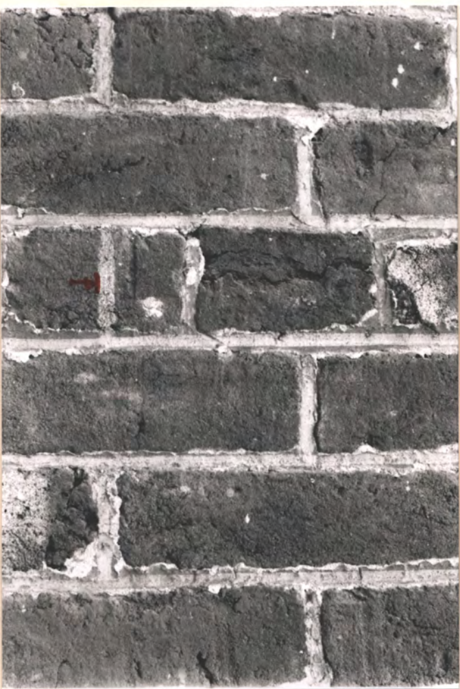
white paint "pencilled" joints (typical of 19th c.)
