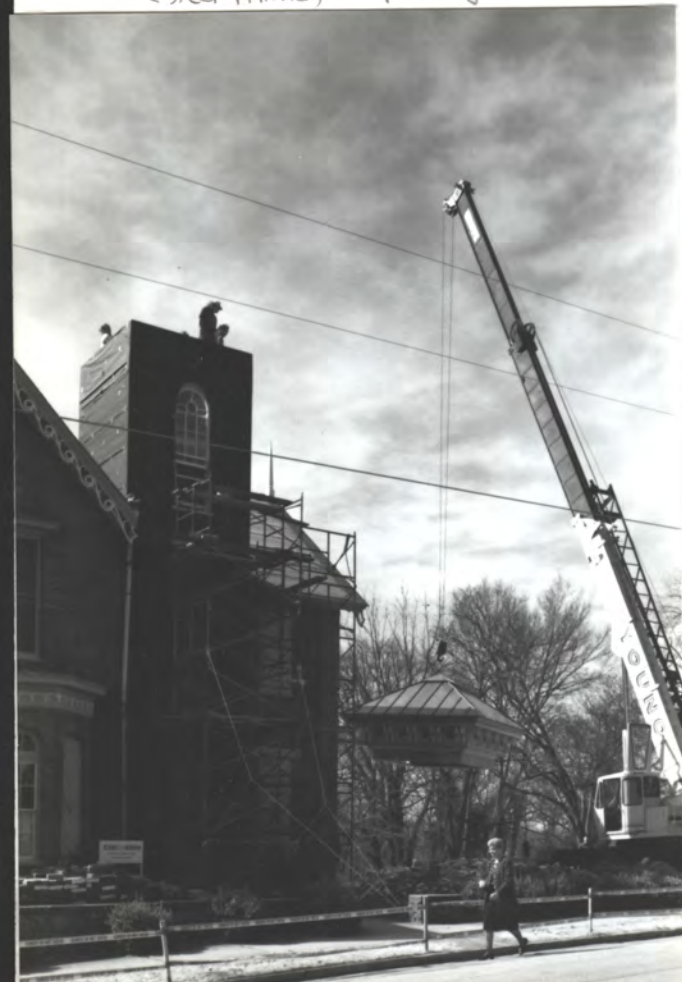
② Tower cap being raised ↑ Revelle Gwynn (Mrs Dwirsky)
