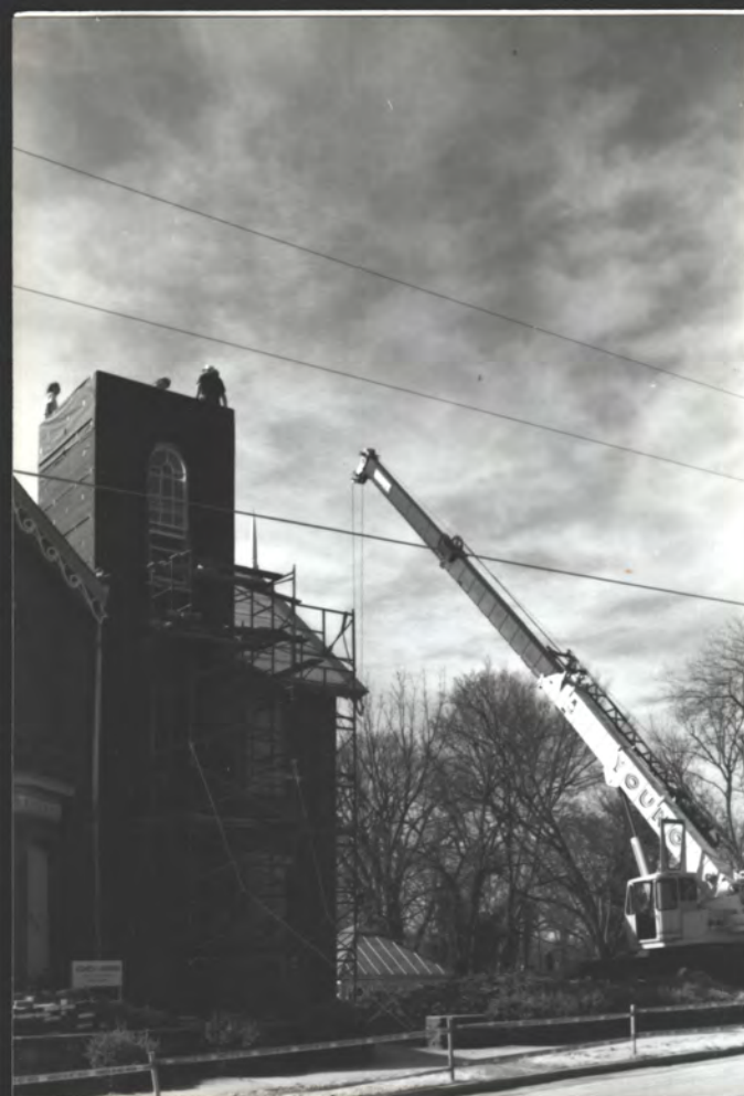
① Prebuilt tower (steel frame) ↑ Pre assembled tower top on ground
