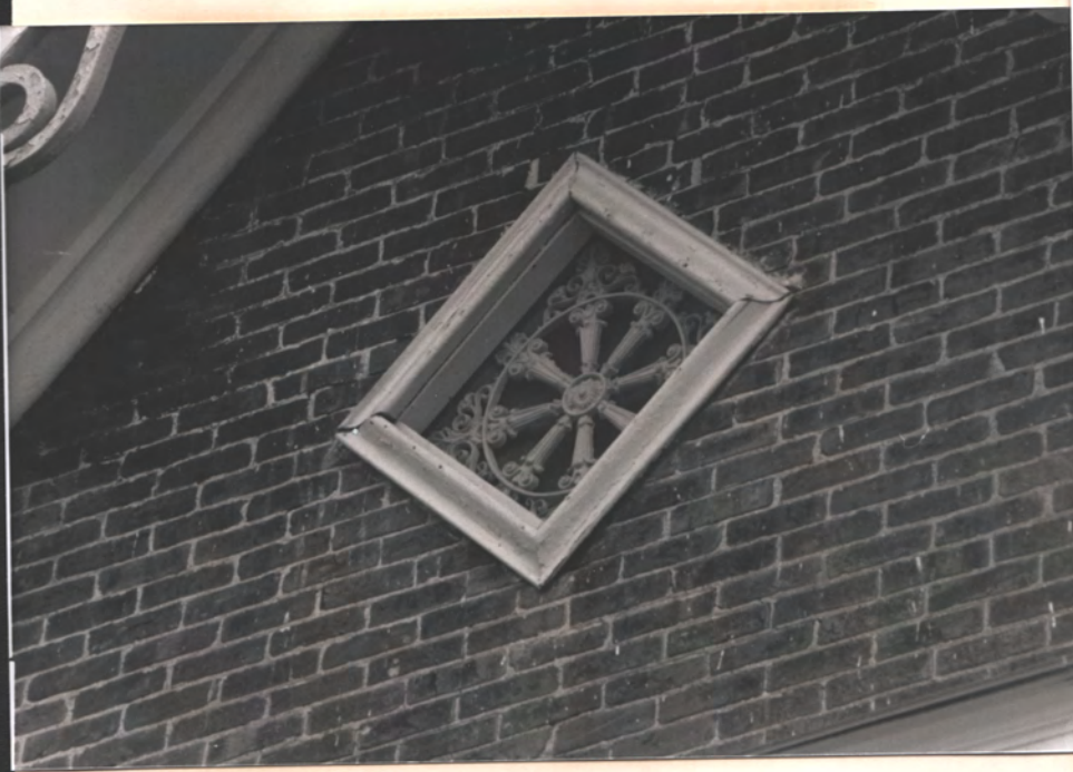
Cast iron vent front gable
