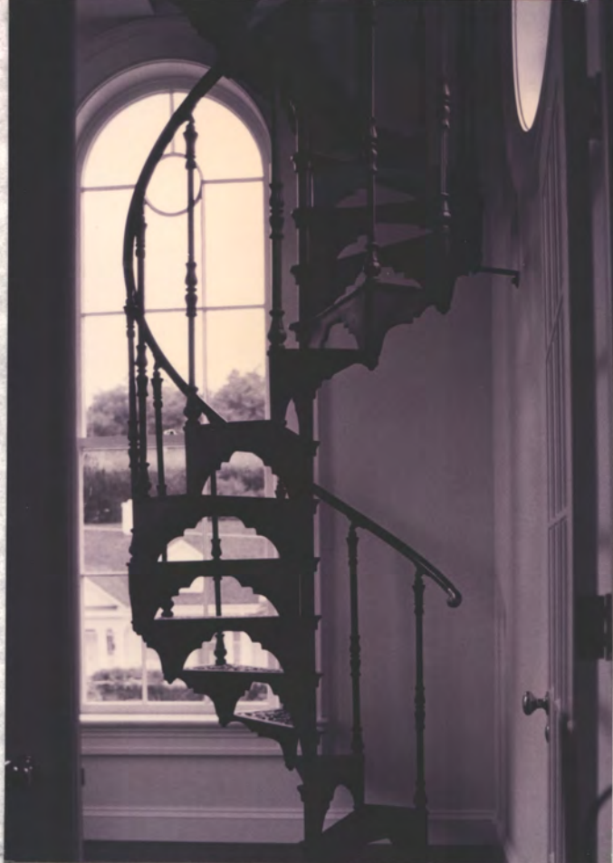
New (1993) CI Stair up to tower rm (HW)
