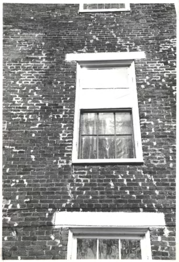
S. Wall Poorly patched bricks etc
