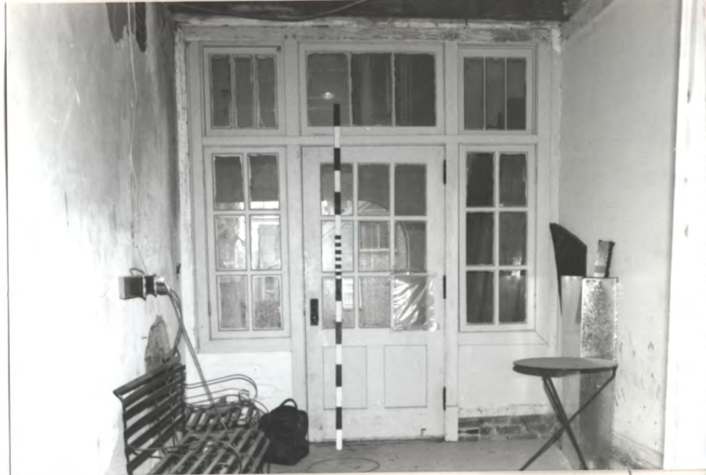
Basement, East door to lower porch N ←
