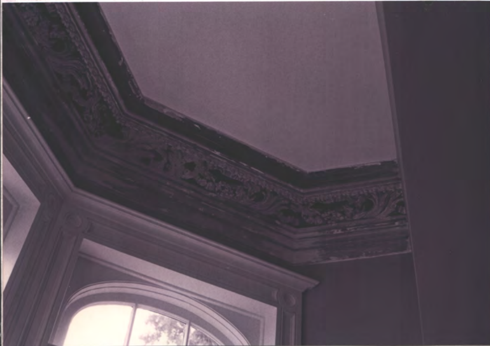
← Undamaged orig. plaster cornice in NW Bay ↑ N DBL PARLORS
