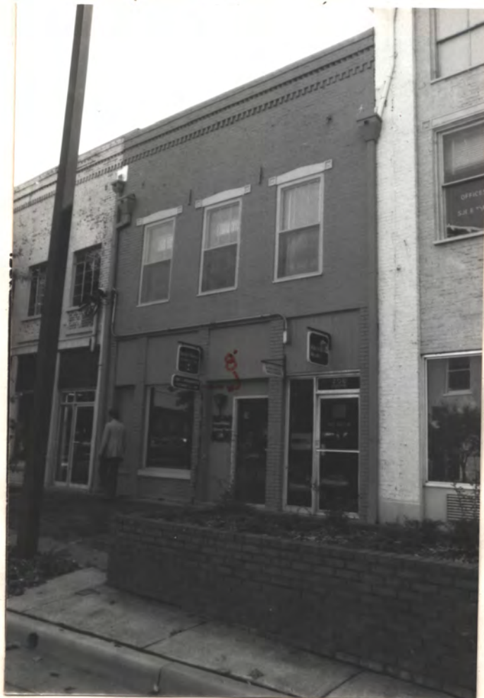
Photo 2 Looking E.S.E Kaufman Store in center.
