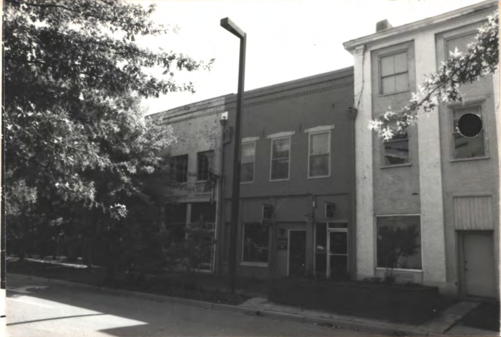
Photo 1 Looking S.E. Kaufman Store in center.
