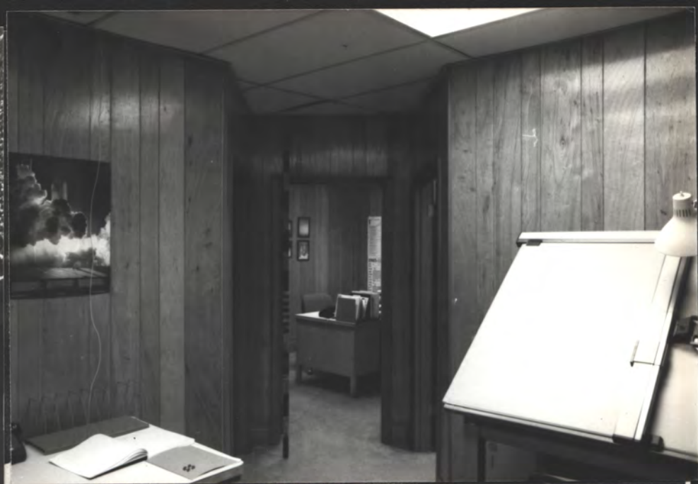
Photo 6 Second floor modern finishes. Ceiling is dropped about 16 inches below original plaster ceiling.
