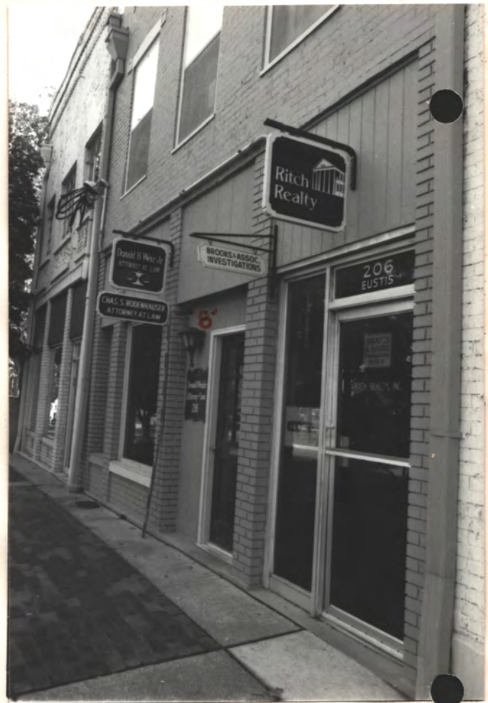
Photo 3 Looking E.S.E at ground floor. Clerestorys are boarded over.
