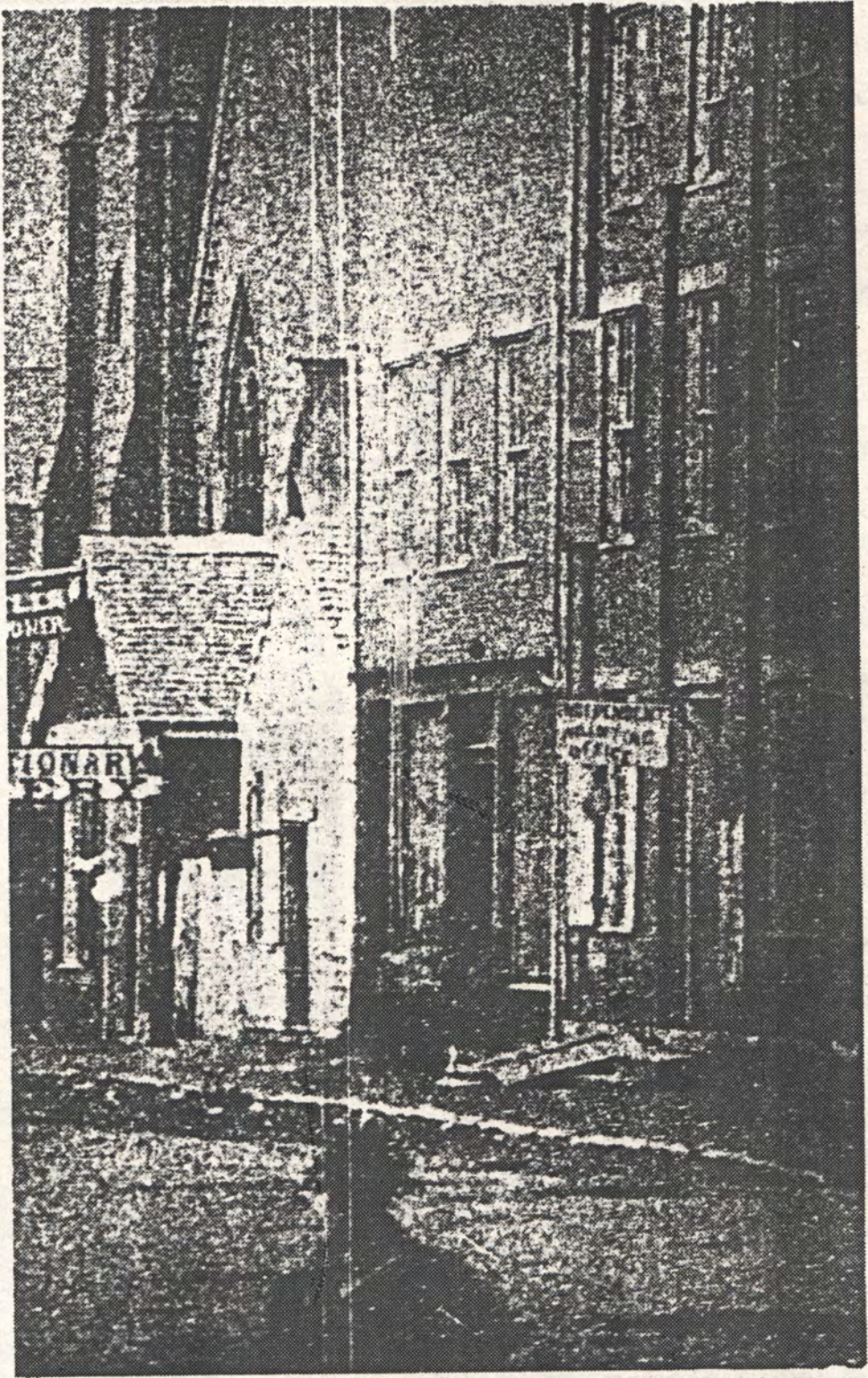
PHOTO 1 - PRE-1884 PHOTOGRAPH SHOWING ORIGINAL FACADE. (SEE PHOTO 2 FOR DETAIL)
