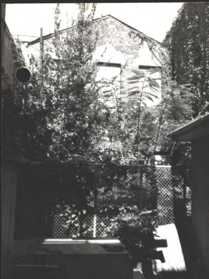
Photo 4 Looking north at rear ( 2 and 2/3 story).
