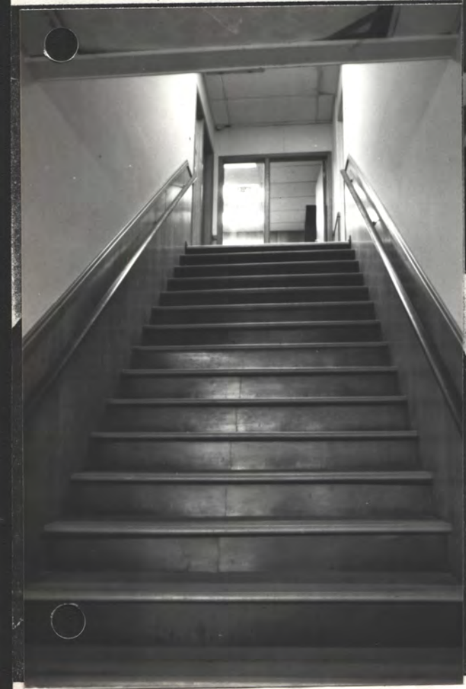
Photo 5 Stair to 2nd floor.
