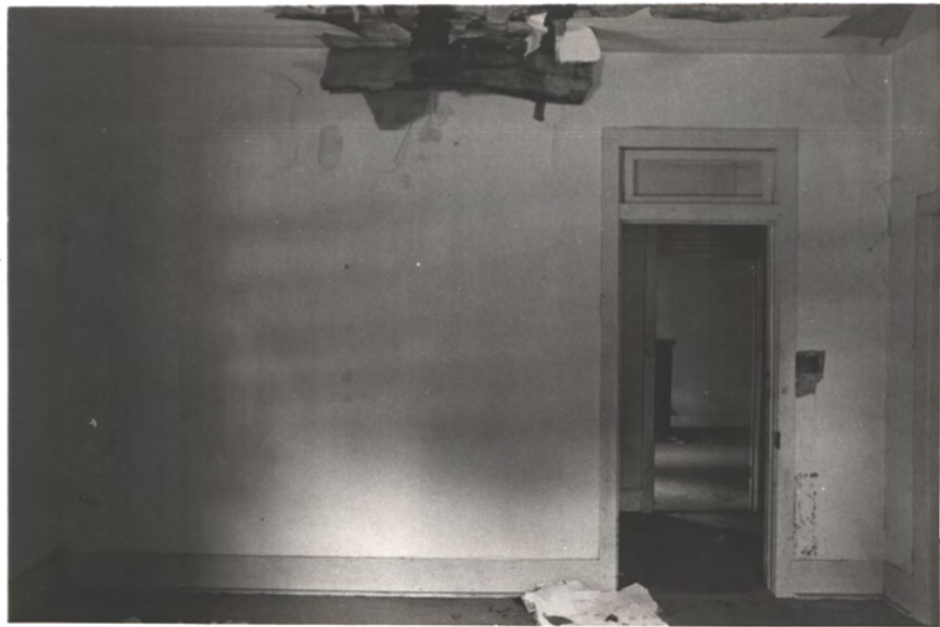
North wall of SE Room
