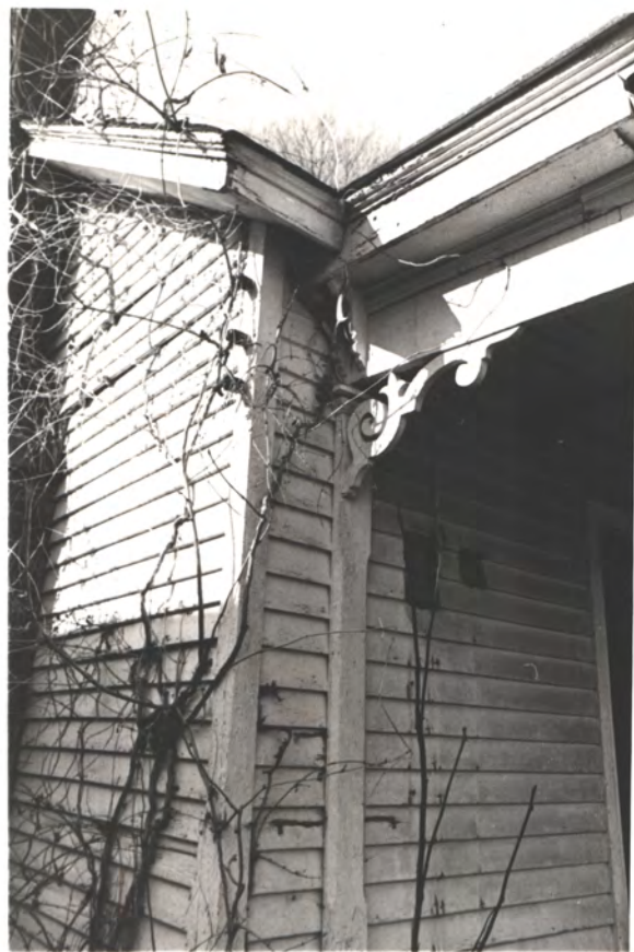
South EAST CORNER
