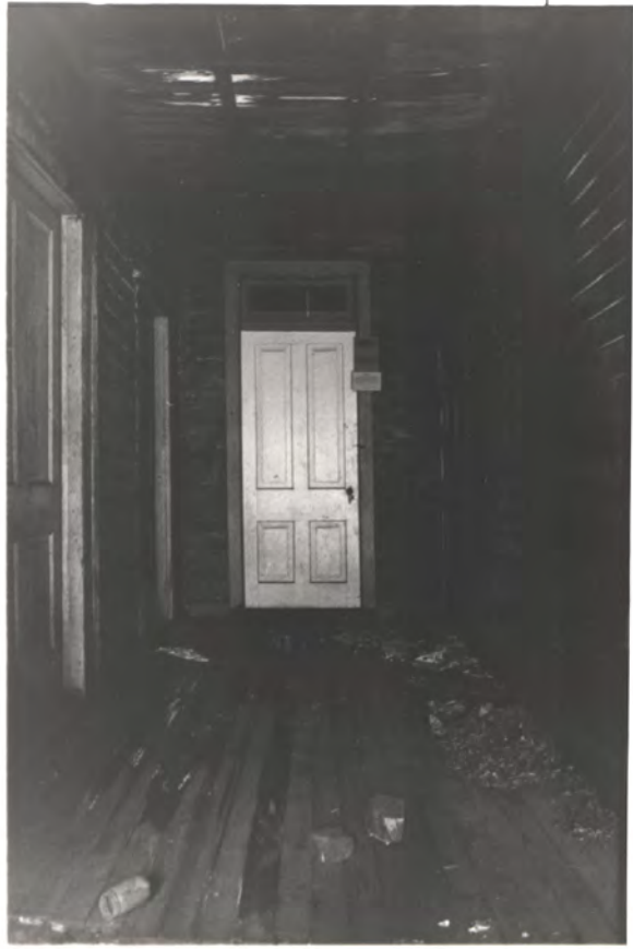
BACK HALL- LOOKING EAST
