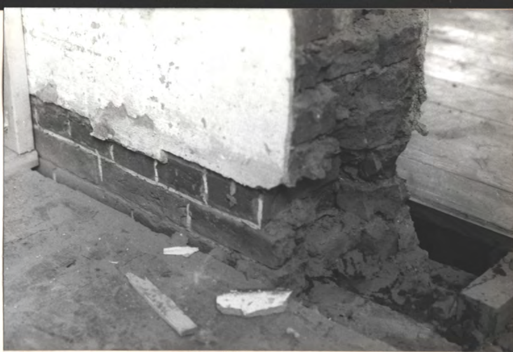
West wall of back stairs hall. "Pericilled" brick to face brick prove that this was an exposed wall, w/ N.E. wing added later in Fed period
