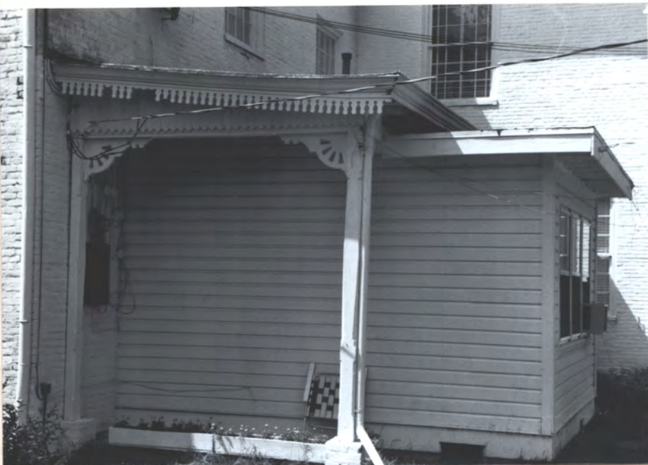
20TH. CENT. RM INSERTED UNDER VICTORIAN PORCH AT REAR S.E. YARD
