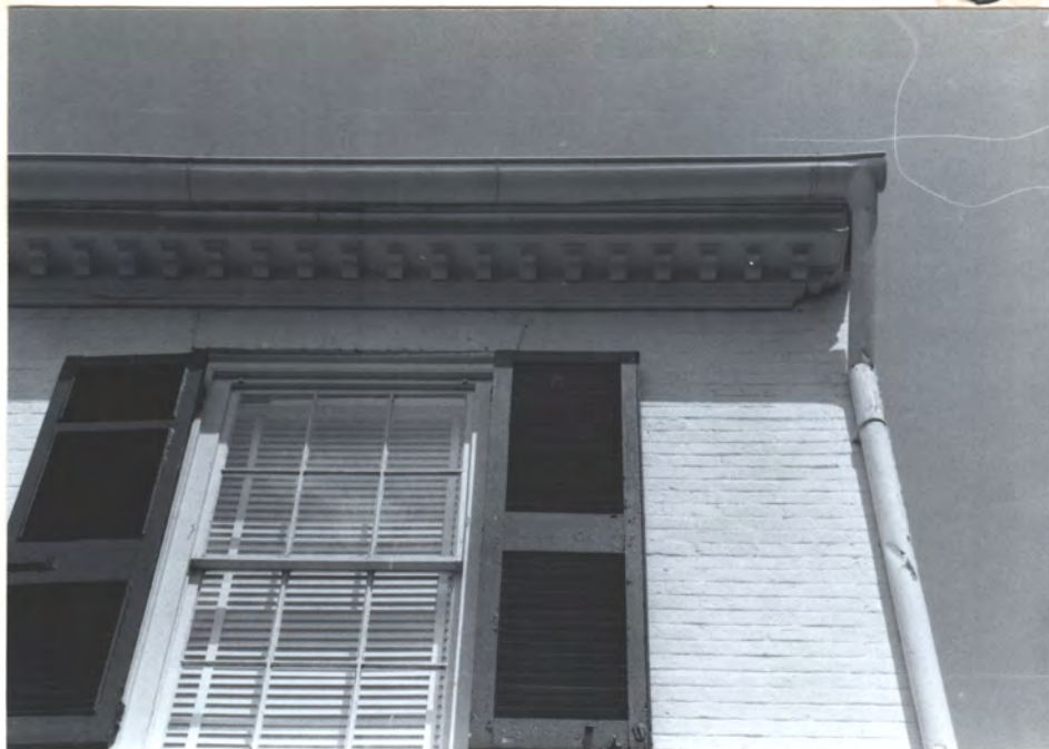
WEST WALL, S. END, 2ND FL.
