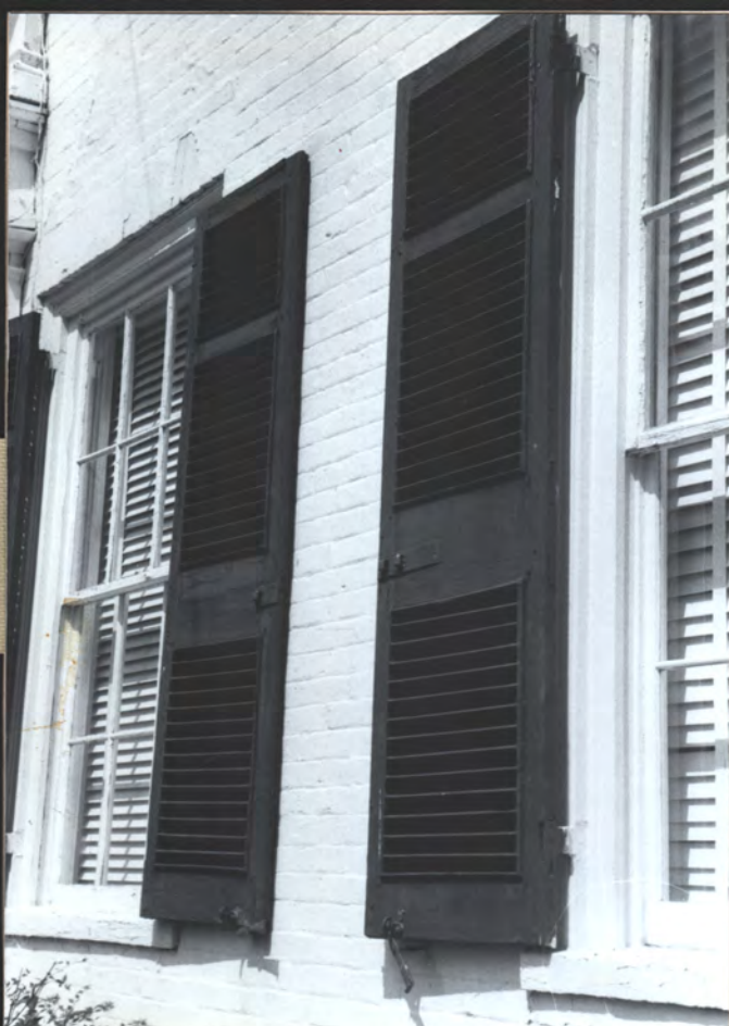
WEST WALL, S. END 1ST FL.
