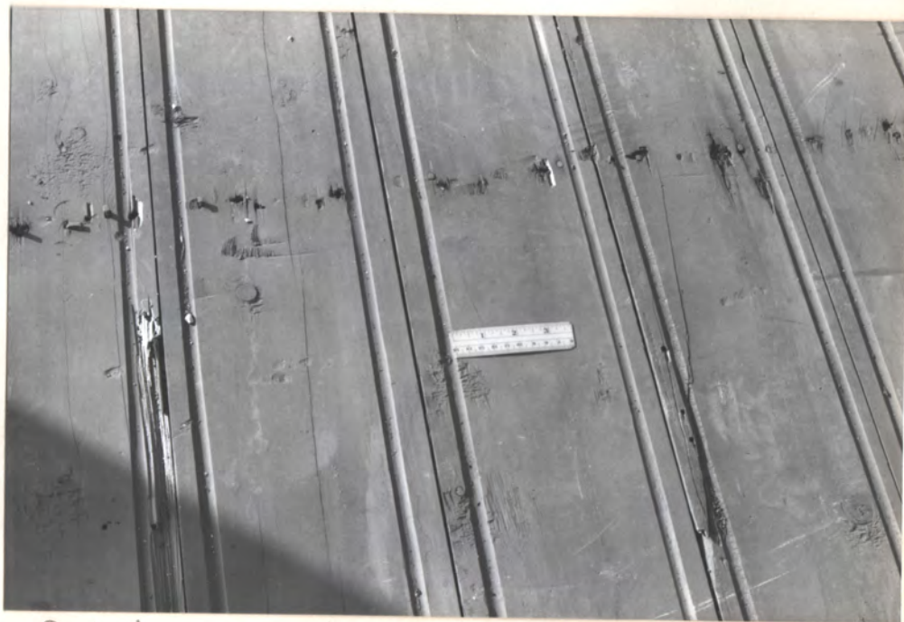
2nd fl. portico fl. - heart cedar, original (was covered by later fl.) - jack plane marks. Grooves to channel water to edge N →
