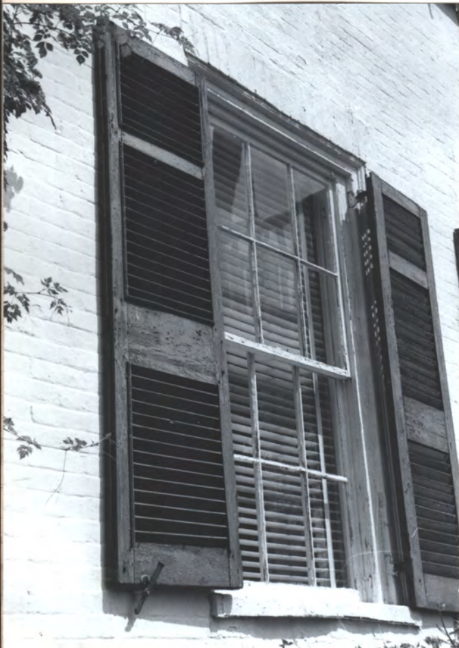
WEST WALL, N. END, 1ST FL.
