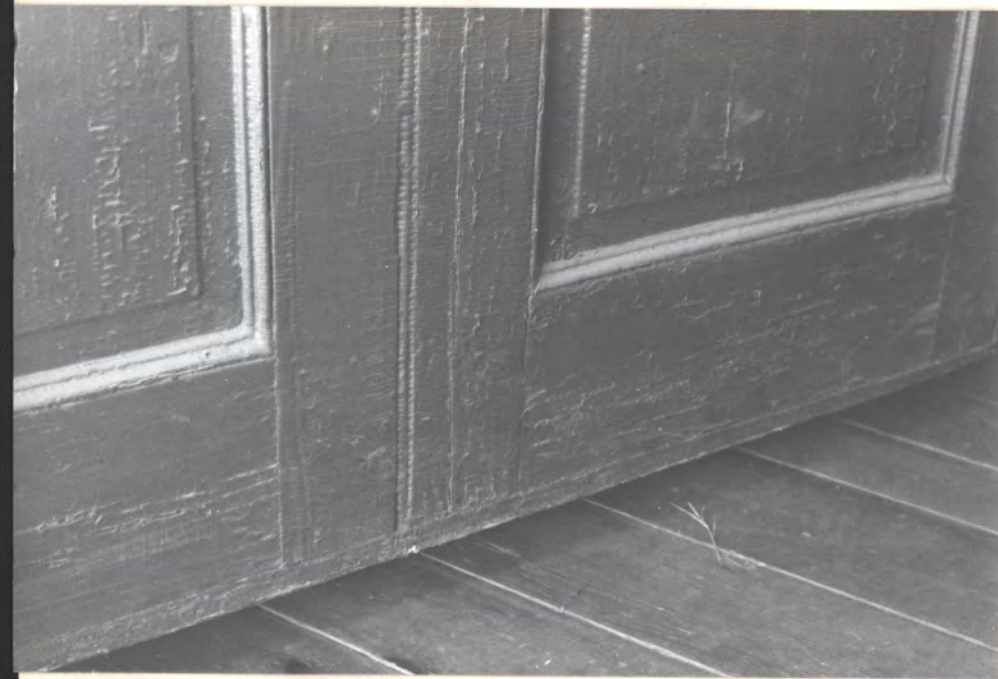
Front door outer face, + entry fl. Door is ± 4' wide & designed to look like a pair of 2' doors. Note false ft. N →
