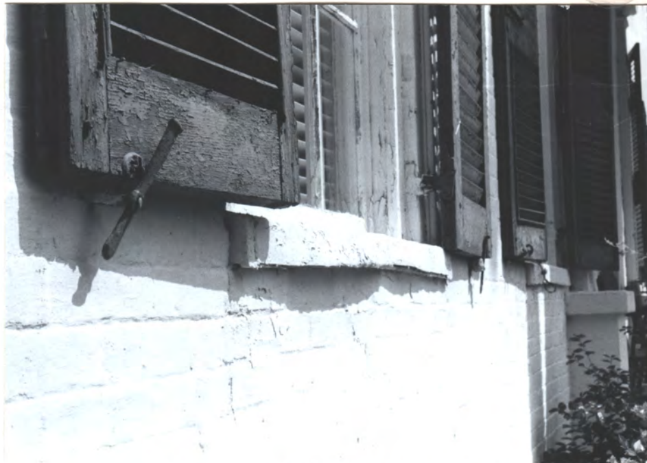
WEST WALL, N. END, 1ST FL
