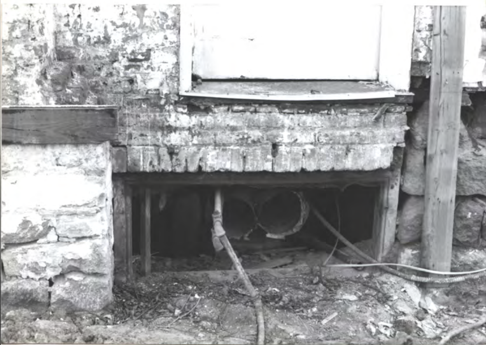
→ N Door is V&Z, but opening is original (see brick jambs)
