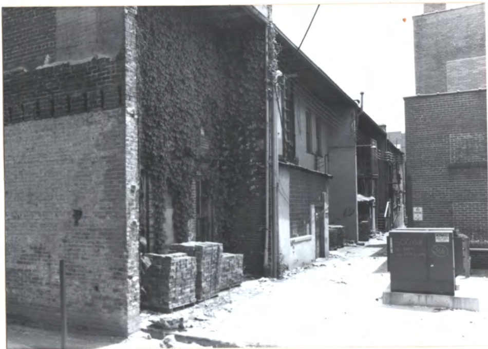
N. end of Alley to W. Clinton Ave
