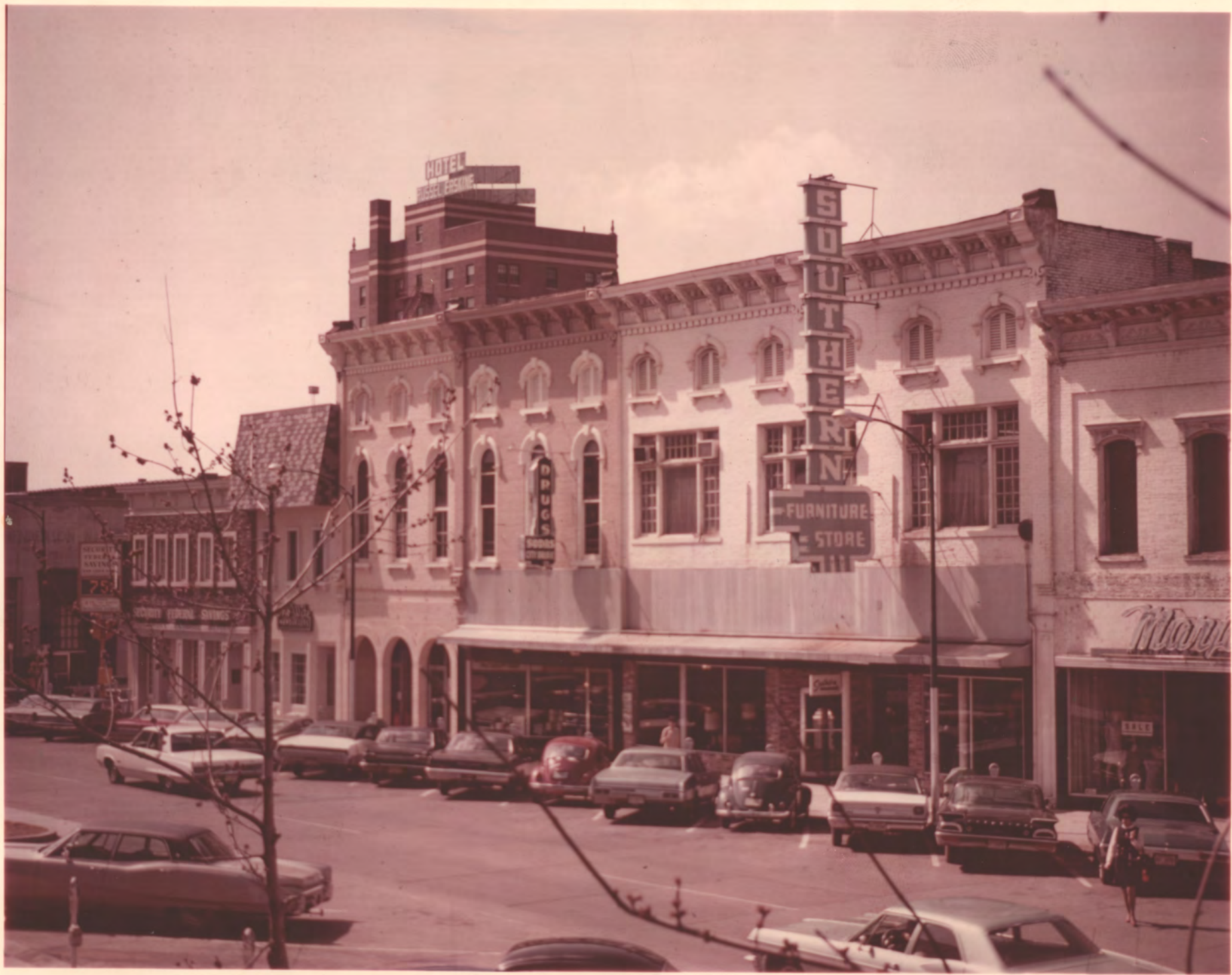
N. Side sign in ca. 1972 From: sign #187D ± w/ 20th c. name building (was on 1871 N. side of Administration) name building again in ca. 1969 by JH, Arch.
