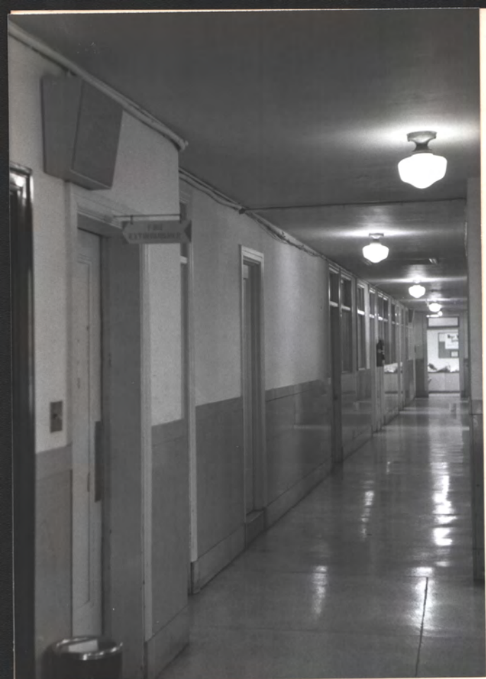
2nd fl. west wing Corr. looking west
