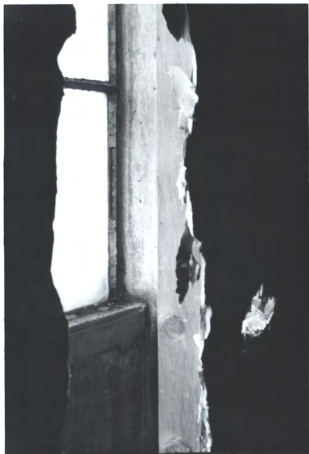
1920's Steel sash + spandrel + col. of conc.
