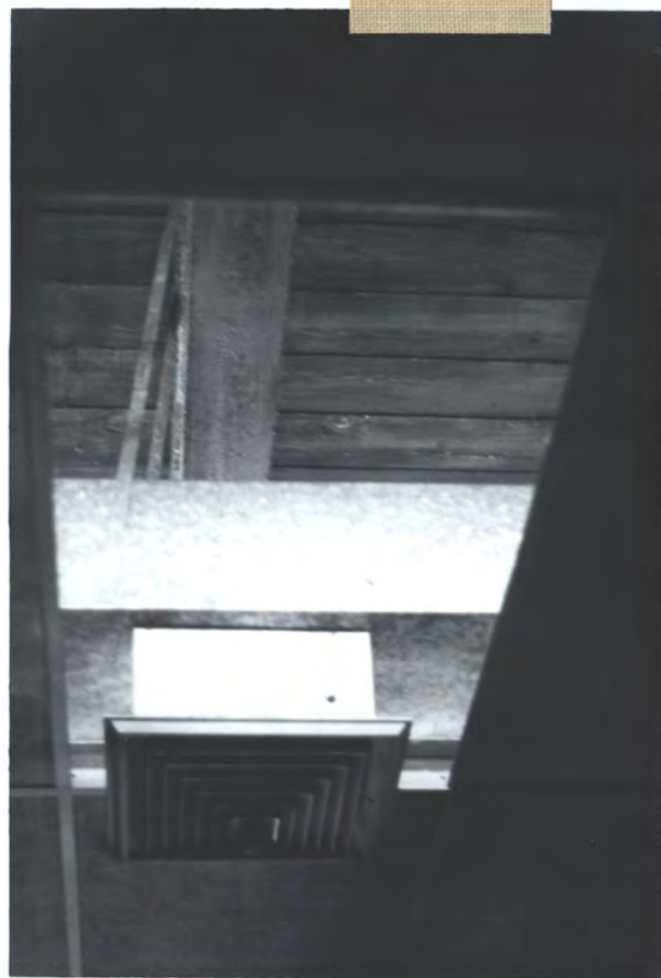
Wood roof or floor (thick, wide) + wood beams, typical. (lower col. is early 1960's acous. tile)
