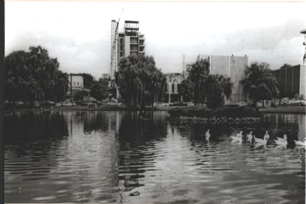
City Hall under constr. - 1963 City Hall, designed by HO for W.E. Dickson, Arch.; 1963
