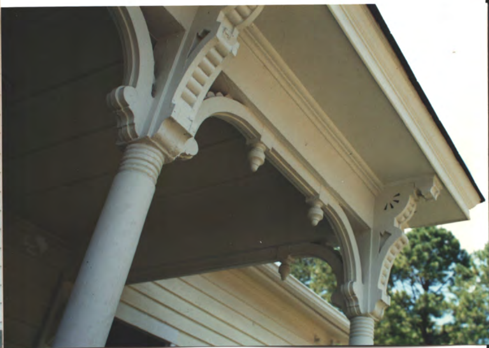
latter 1800's porch (columns) → H
