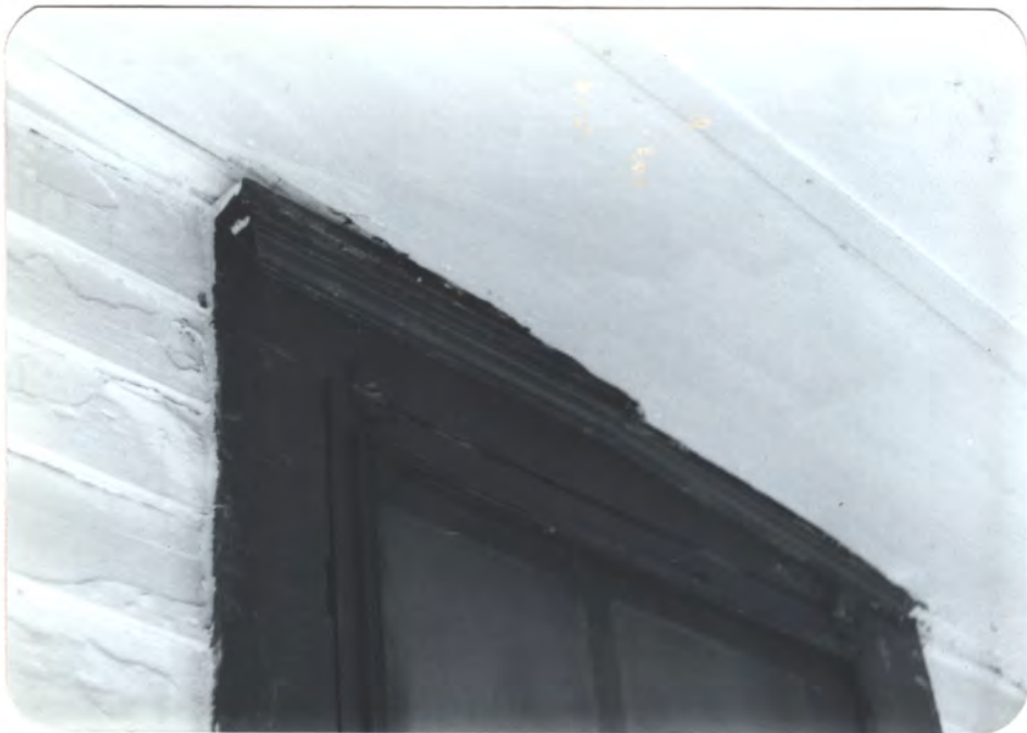
front porch siding
