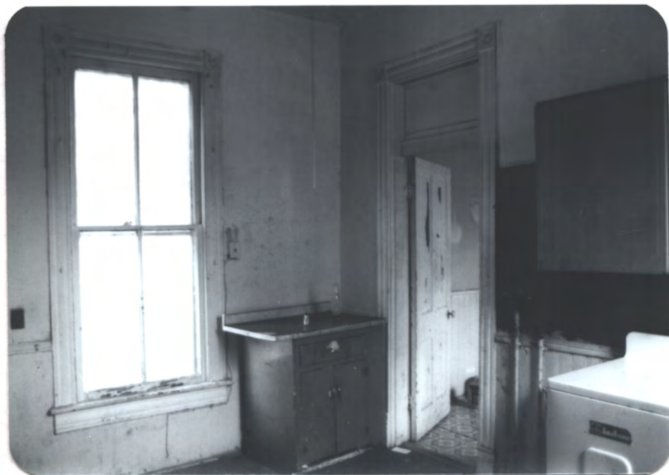
Enclose north porch looking S.E. into W-N.C. Rm.
