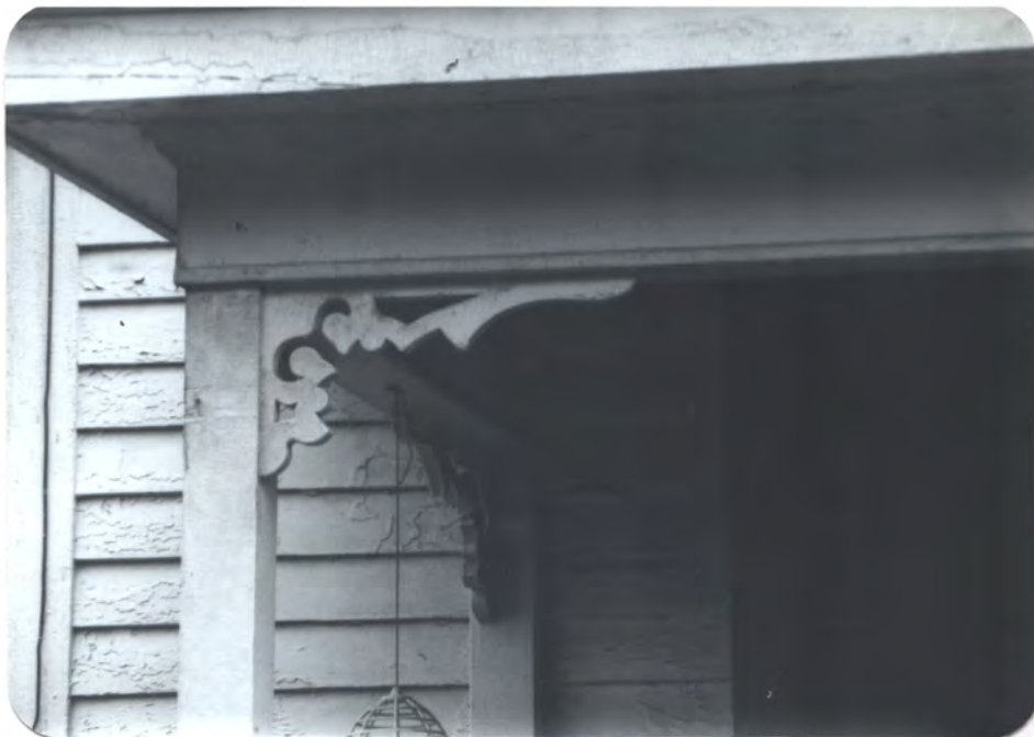
S veranda SW. corner
