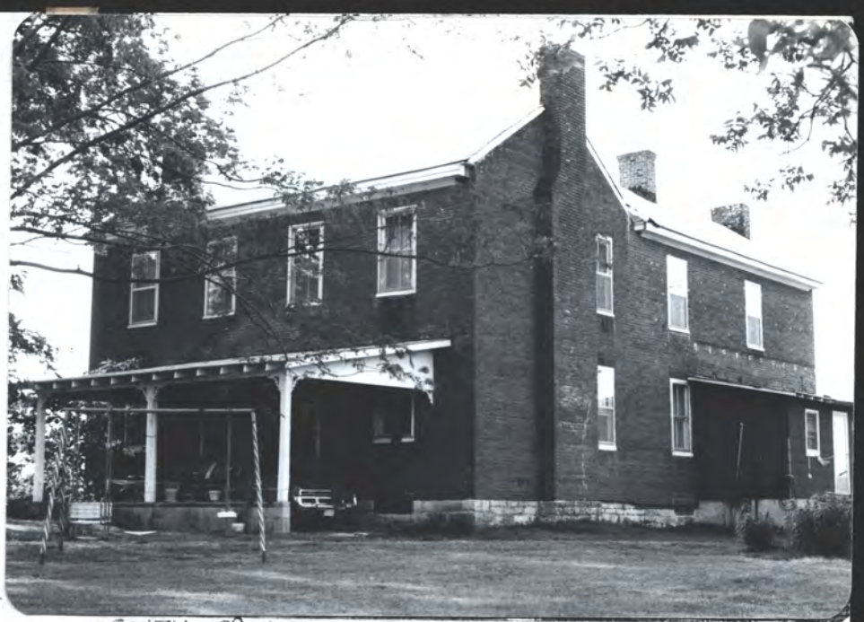
SOUTH FRONT, ADDED PORCH & SHED RM.
