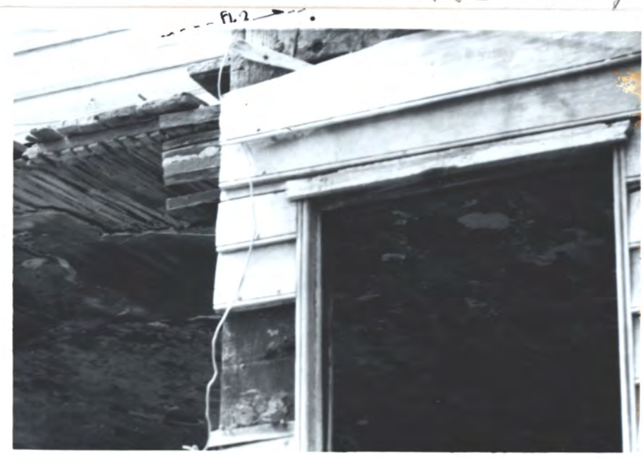
N. front wall beaded pre 1830 jmb (window op.)
