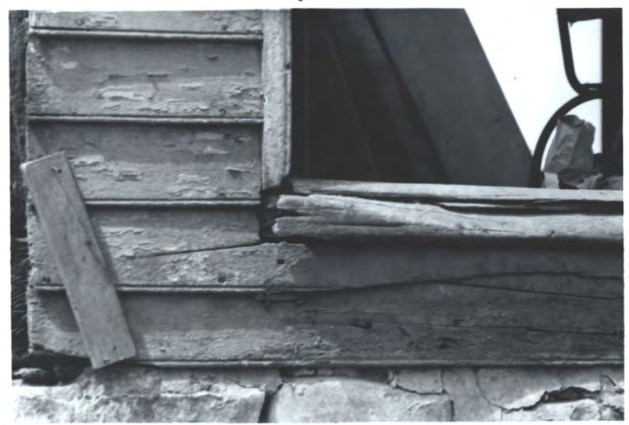
pre 1830 beaded clap'd, beaded sash jamb S.W. CORNER
