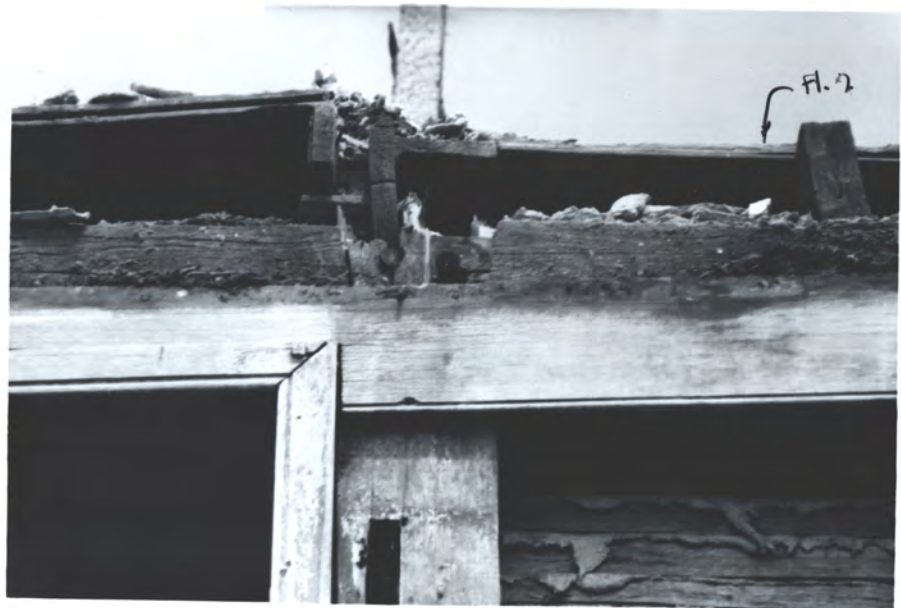
beaded jamb wd. lath (back) & plaster kerns
