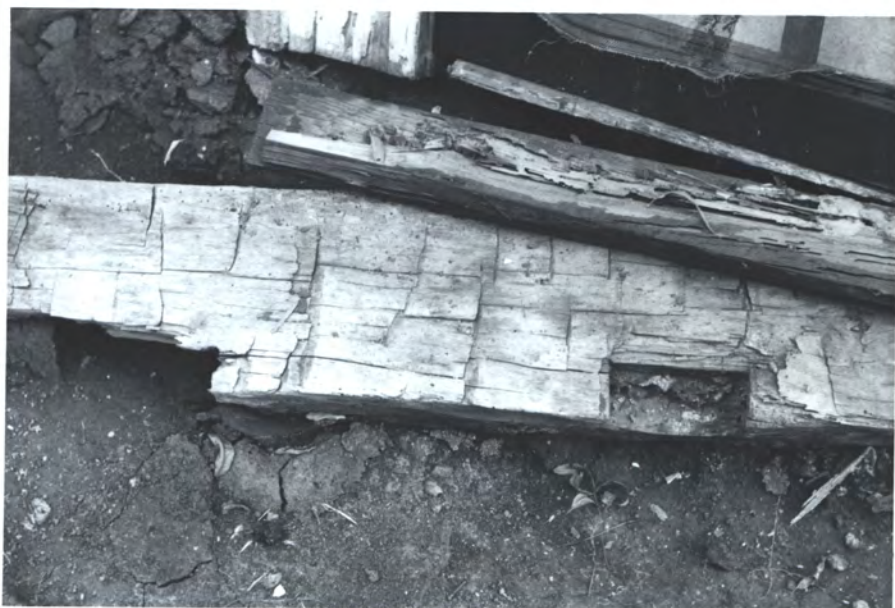
Hem. fl. joist at N.W.M.
