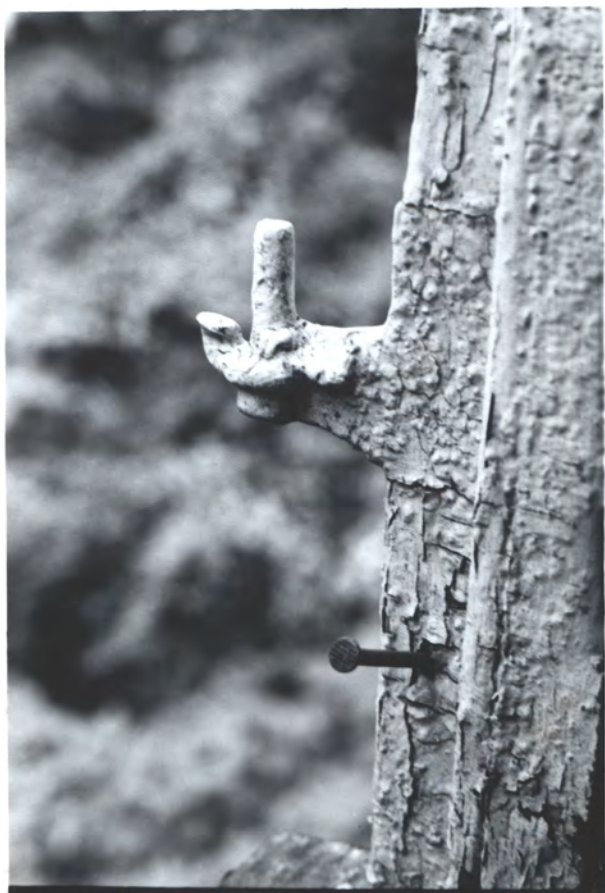
C.I. cam-action blind hinge at Fl. 2 front window
