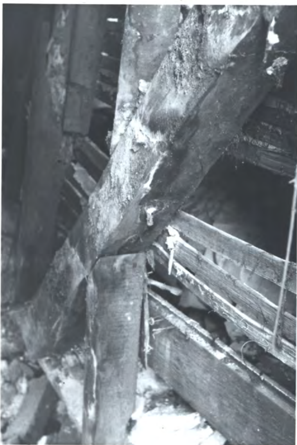
N.W.M., N.W. corner - by the (note SASHAW marks on wall)
