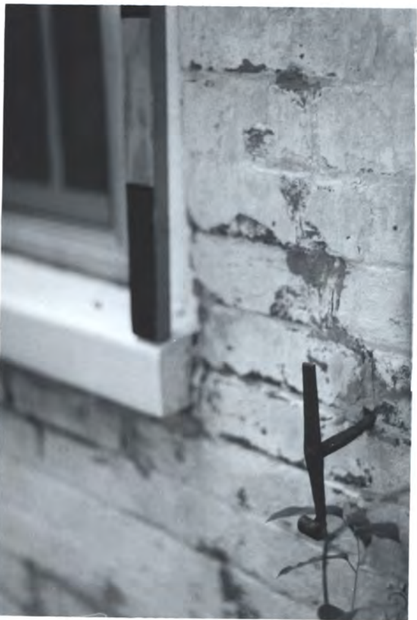
blacksmith-made shutter-holdback (N.I.)
