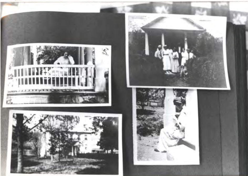
4 early 20th c. photos showing the c.1816 portico (bottom 16" of cols is patched) Porch rebuilt c.1922, raising only the cutoff-cols. (bottom ± 3' cut off)
