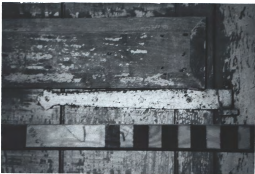
Cellar door, top hinge (W.I.) blacksmith - mark strap
