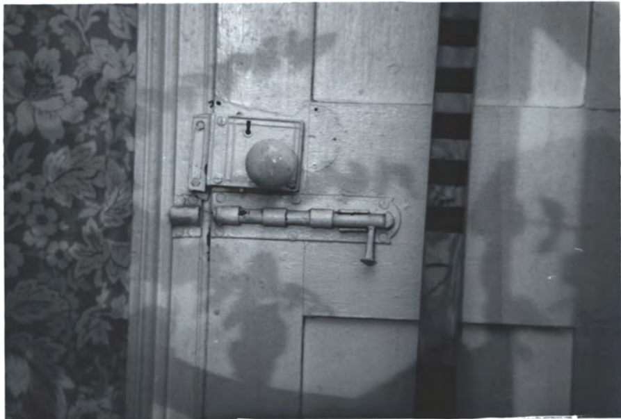
Recent lock, but NOTE shadow of Bolt-latch looks c. 1916 type
